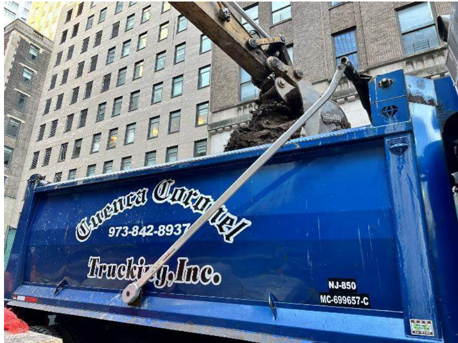
Photo 1: View of Urban live-loading a truck with excavated non-native soil/fill from the southern part of the site (facing west).
