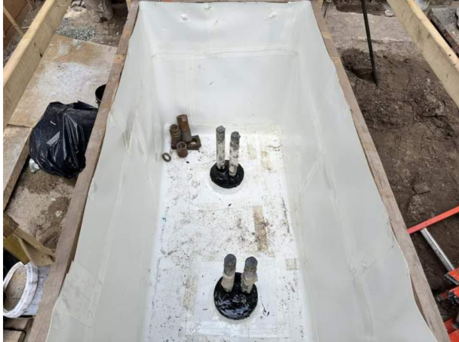
Photo 2: View of reinstalled waterproofing/vapor barrier membrane in the southern part of the site (facing north).
