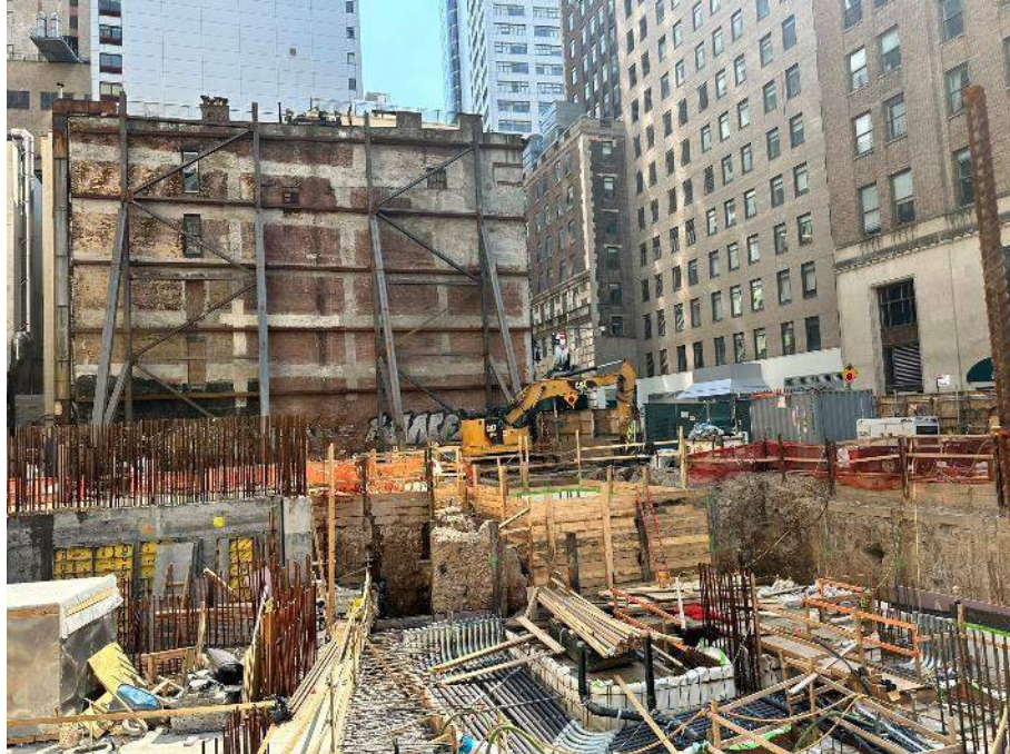
Photo 2: General view of the site at end of day (facing south).
