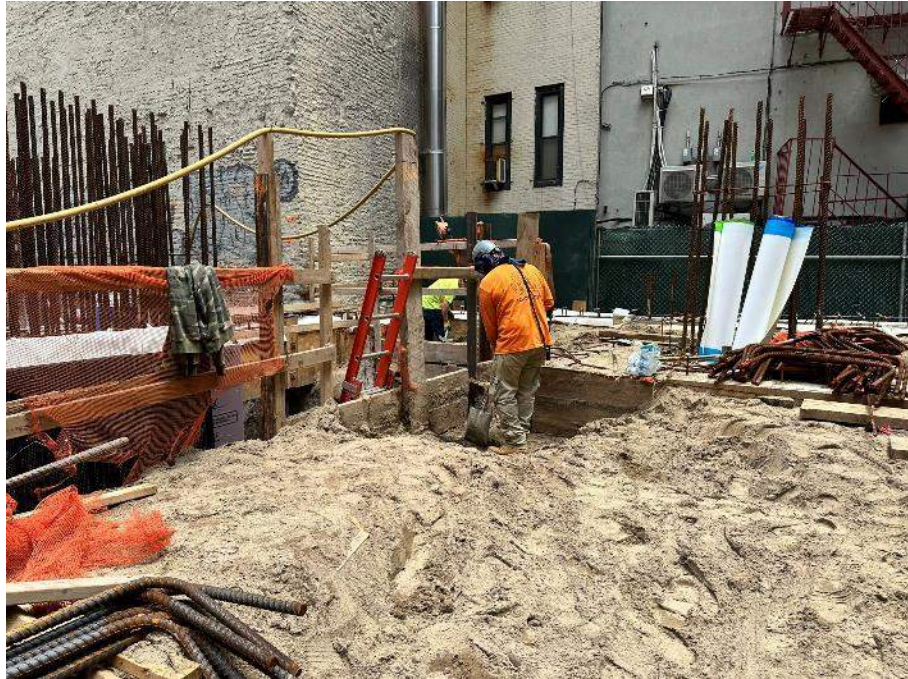
Photo 1: View of Urban excavating clean sand in WC05 (facing east).
