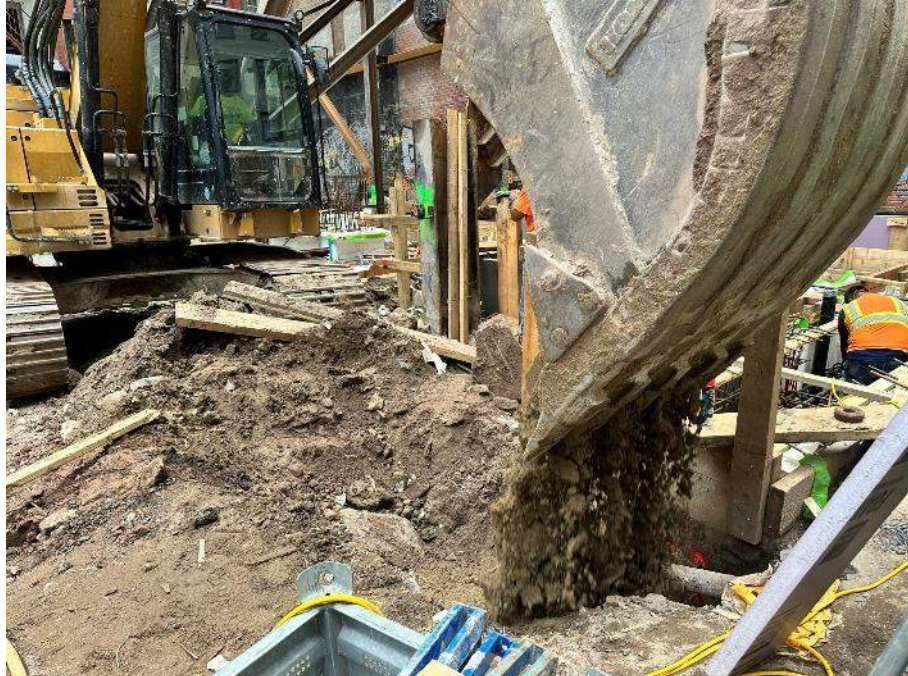
Photo 2: View of Urban backfilling an area of excavation with clean sand in the southwestern part of the site (facing southeast).
