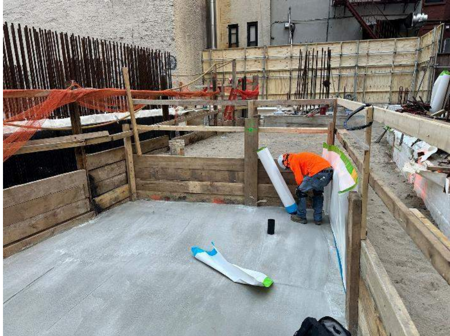
Photo 2: View of Urban installing waterproofing membrane in the southern part of the site (facing east).
