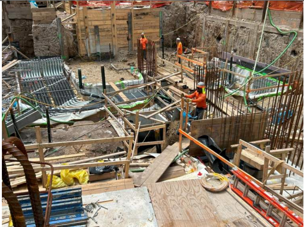
Photo 2: View of backfilled areas in the northwestern part of the site (facing south).
