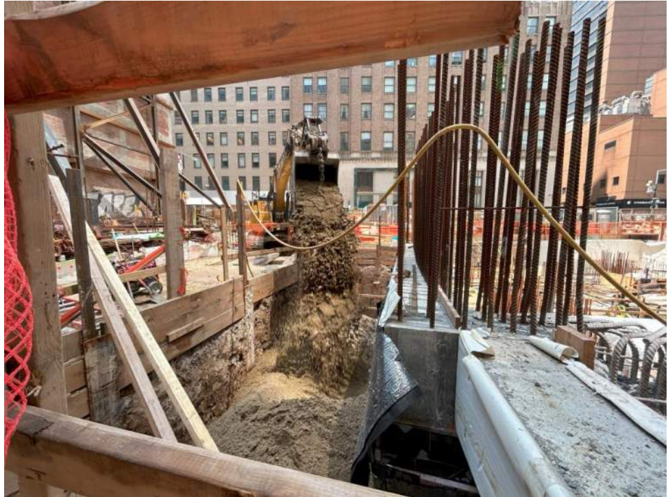
Photo 1: View of Urban backfilling clean sand in the central part of the site (facing east).
