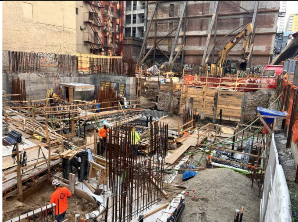
Photo 2: General view of the site (facing southeast).
