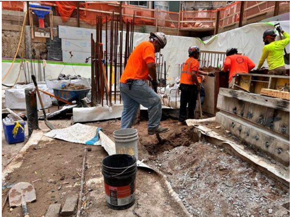
Photo 2: Urban excavating in the northern part of the site (facing west).
