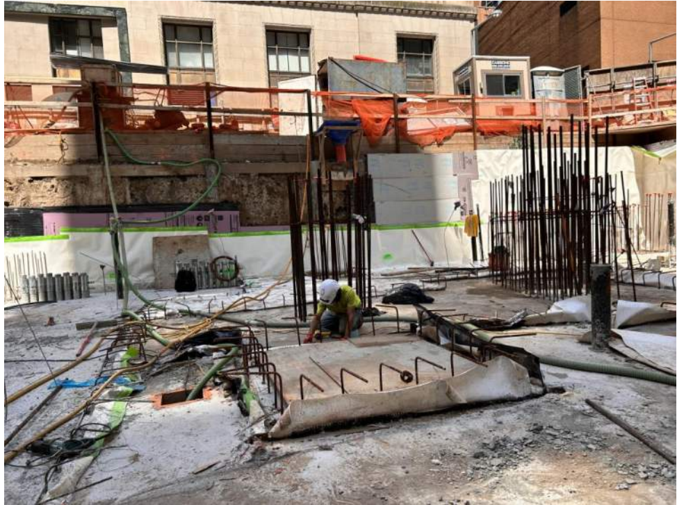
Photo 1: View of Urban installing waterproofing in the central part of the site (facing west).
