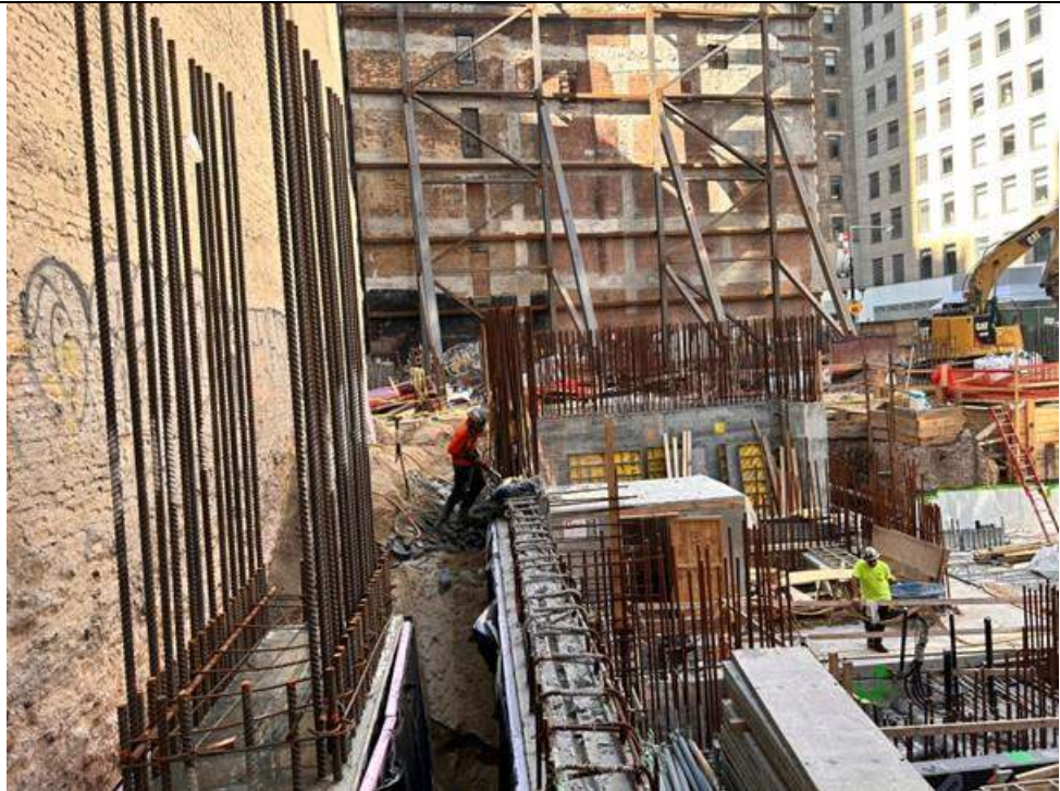
Photo 2: Urban chipping concrete in the eastern part of the site (facing south).
