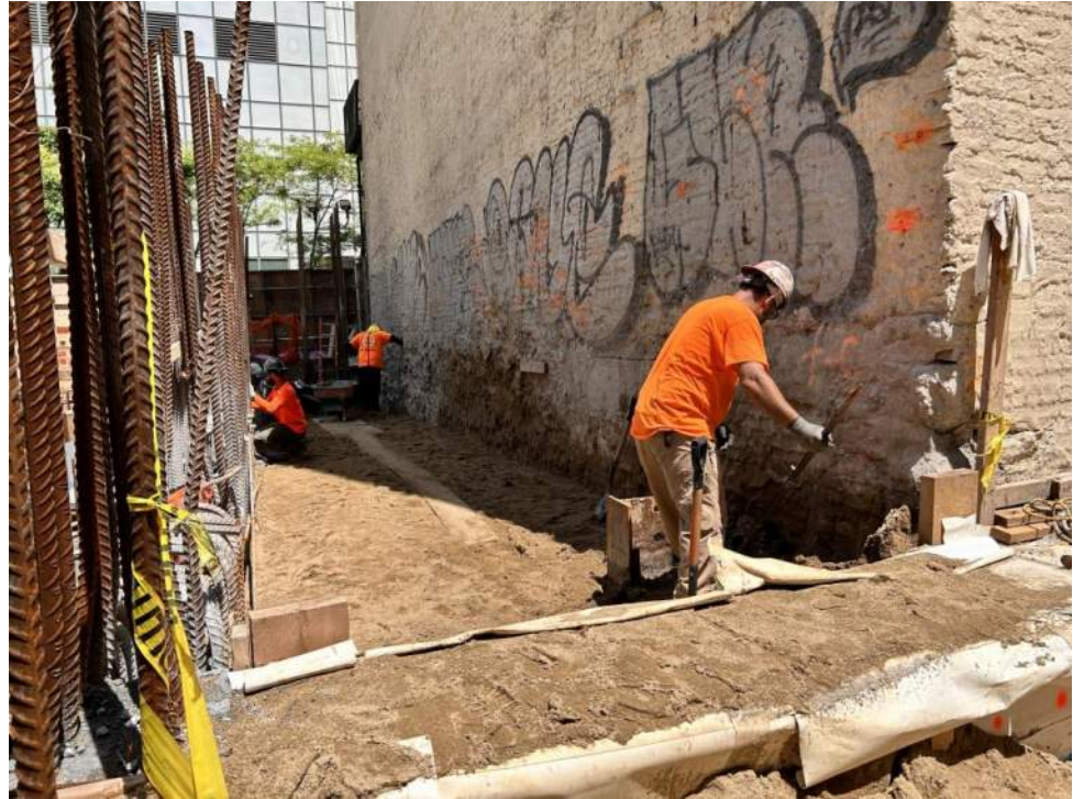
Photo 1: View of Urban grading in the eastern part of the site (facing north).
