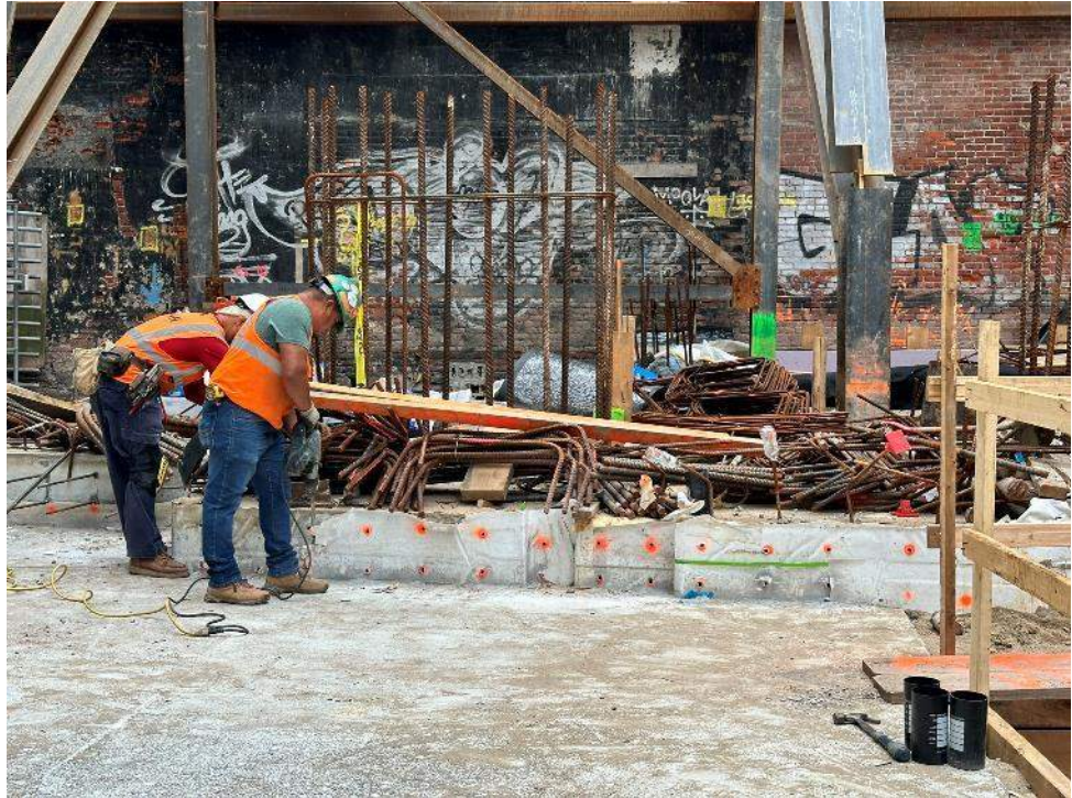
Photo 1: View of Urban drilling in the concrete in the southern part of the site (facing south).
