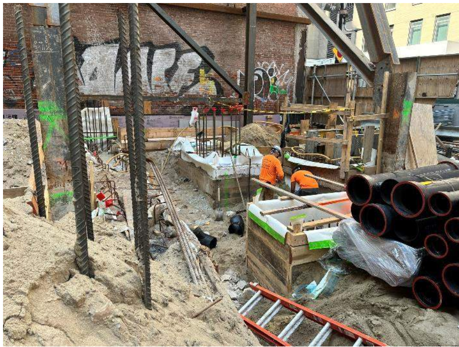
Photo 2: View of Urban using hand tools to excavate clean sand in the southern part of WC04 (facing southwest).
