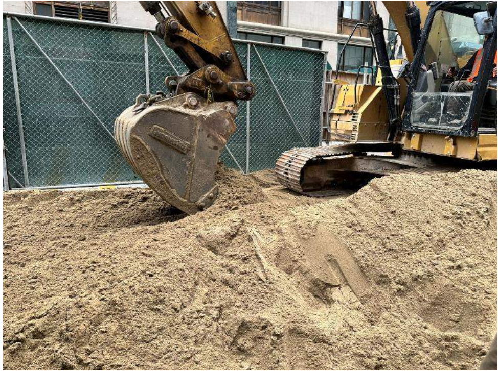
Photo 1: View of Urban consolidating the stockpile of clean sand (facing west).
