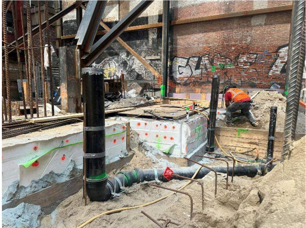
Photo 1: View of Urban drilling into concrete in the southern area of the site (facing southeast).
