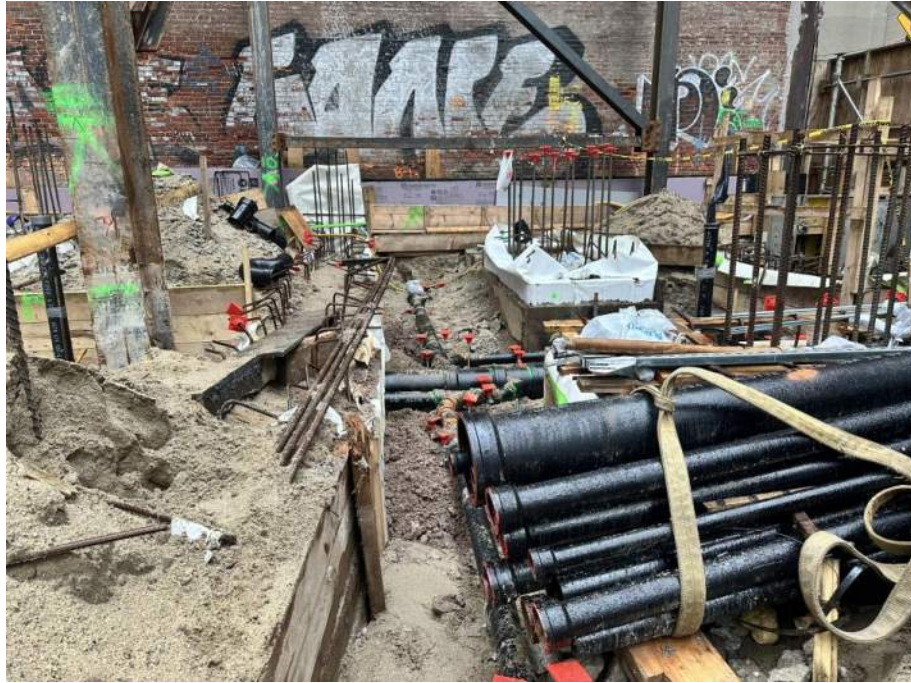
Photo 1: View of backfilled area in the southern part of the site (facing south).
