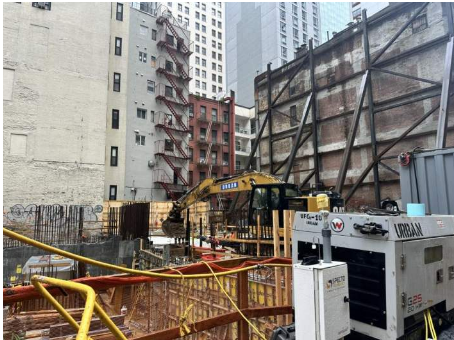
Photo 2: View of Urban backfilling in the southern part of site (facing southeast).
