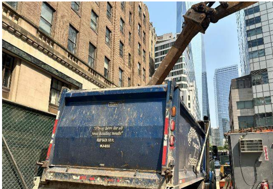
Photo 2: View of Urban loading a truck with non-native soil/fill for off-site disposal (facing north).
