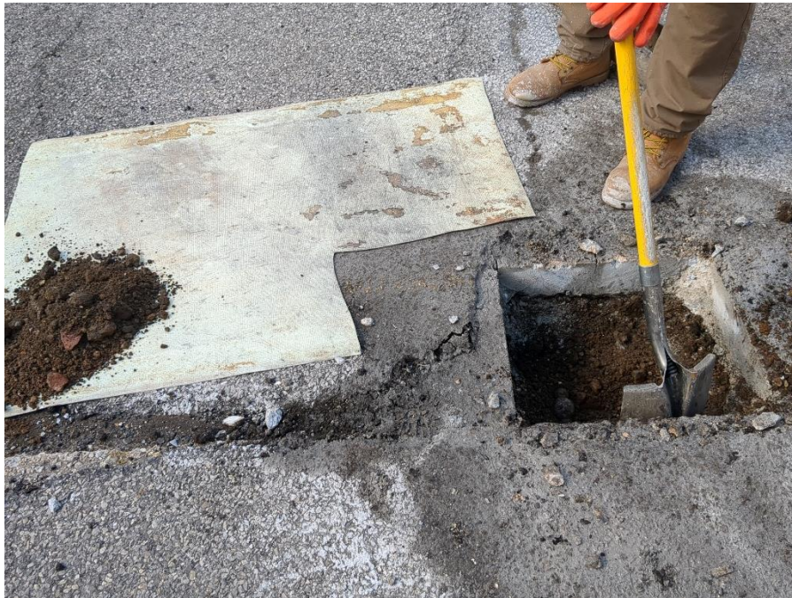
Photo 1: AARCO using a shovel to remove soil/fill for the advancement of soil boring SB11 (facing west).
