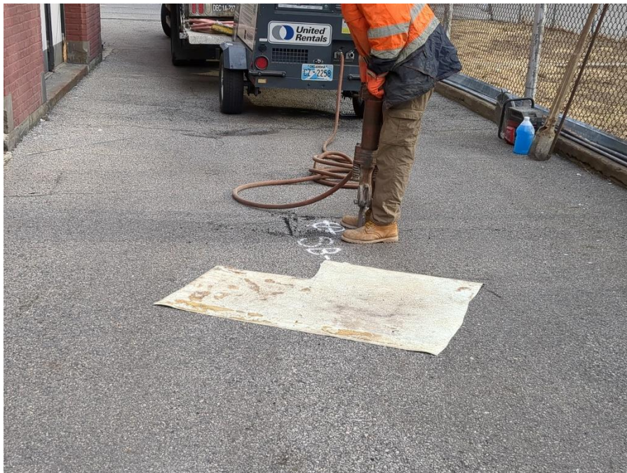
Photo 2: AARCO using a jackhammer to remove asphalt for the advancement of soil boring SB23 (facing northeast).
