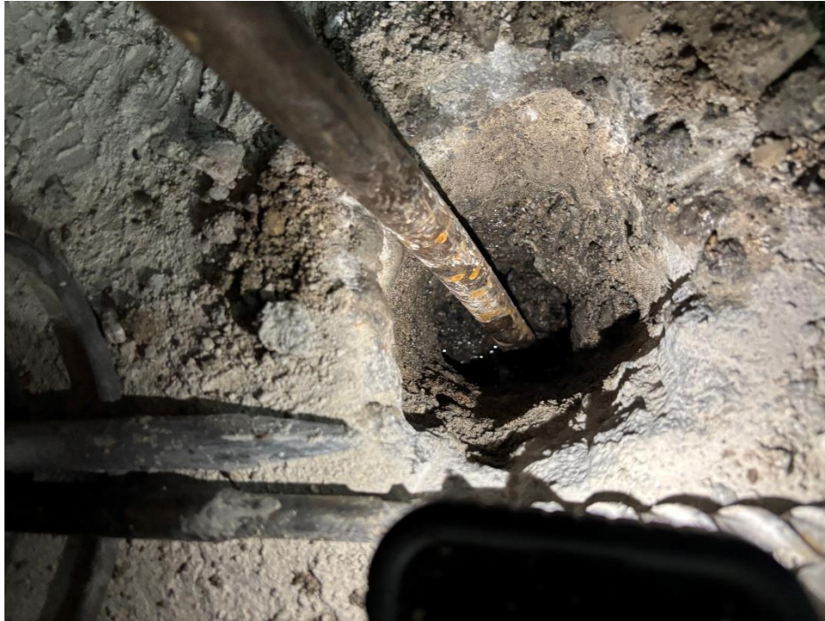
Photo 1: Lakewood hand clearing boring WC07C in building cellar (facing down).
