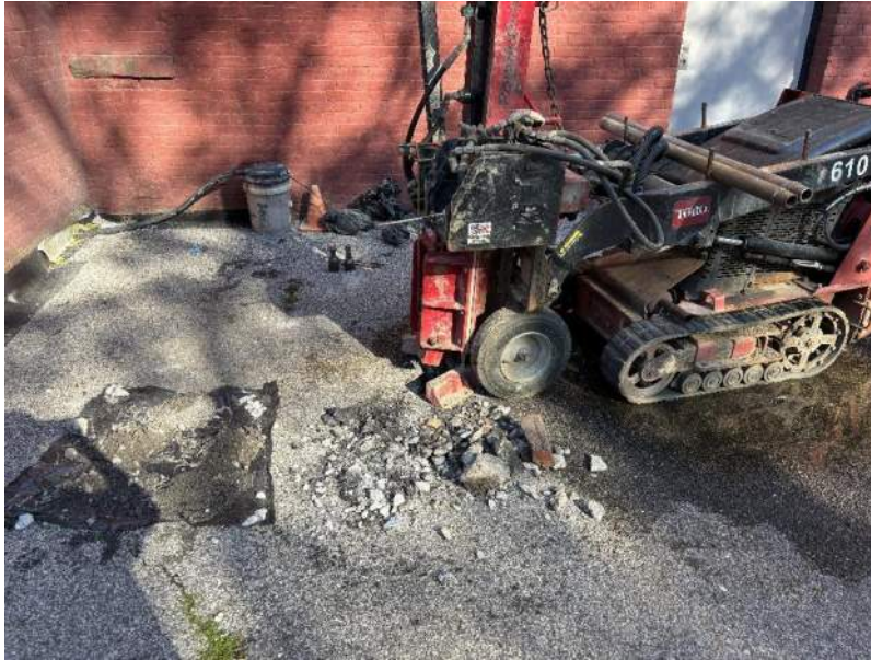
Photo 1: View of Lakewood advancing soil boring WC04C in the northeastern part of the site (facing west).
