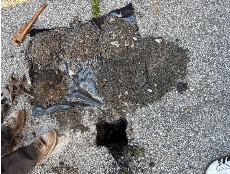
Photo 1: Lakewood hand clearing boring WC01C in the northern part of the site (facing down).
