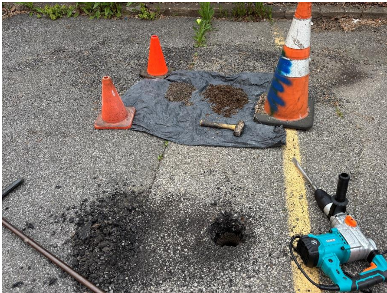
Photo 1: Lakewood hand auguring soil boring WC06B in the southwestern part of the site (facing south).
