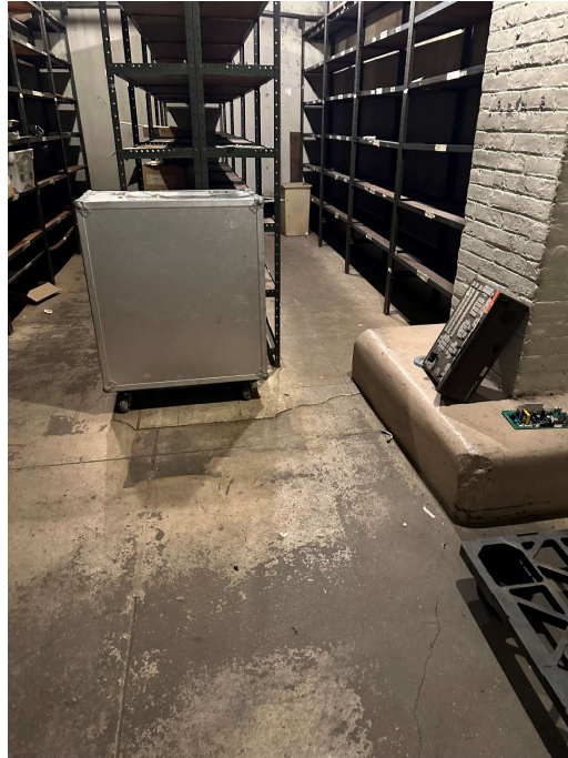
Concrete slab with epoxy coating and linoleum tiles
