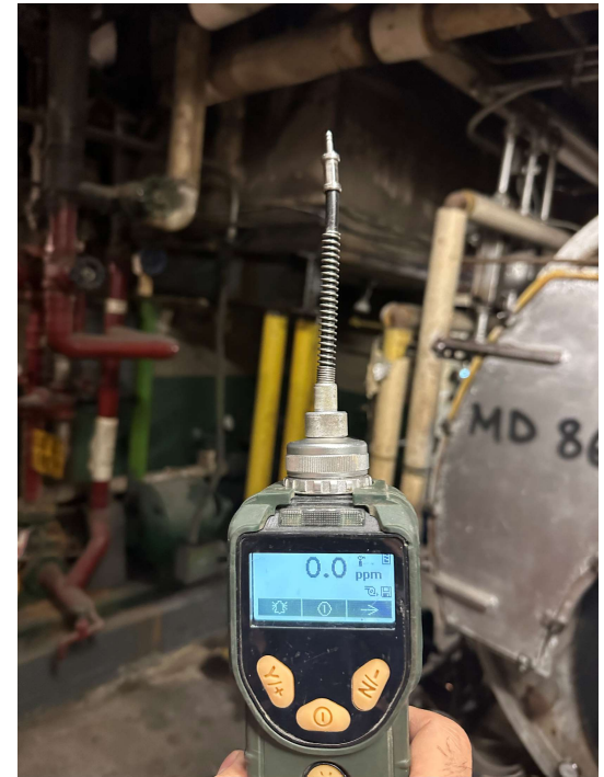
PID survey of indoor air
