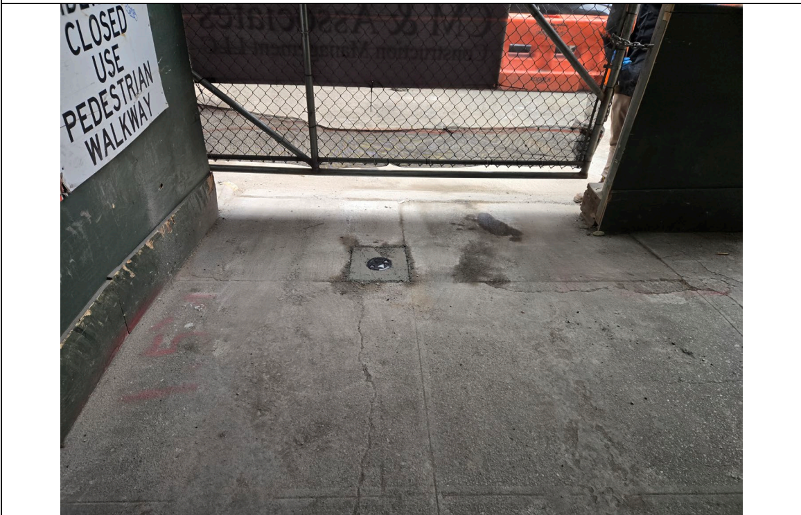
Photo 2: Completed monitoring well MW-8.
