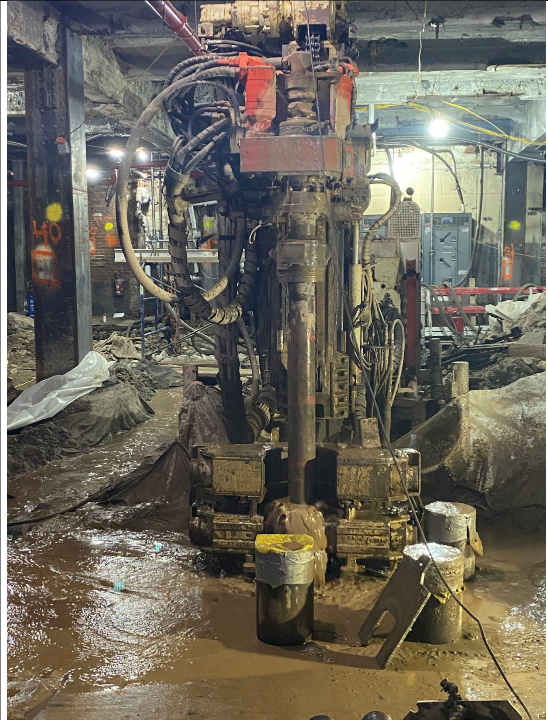
Photo 1: Drilling activities at Pile #23, adjacent to the completed Pile #22.
