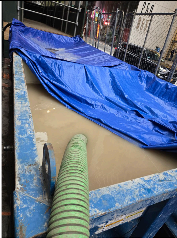
Photo 1: Water holding tank located along West 55 th Street, prior to disposal and cleaning.
