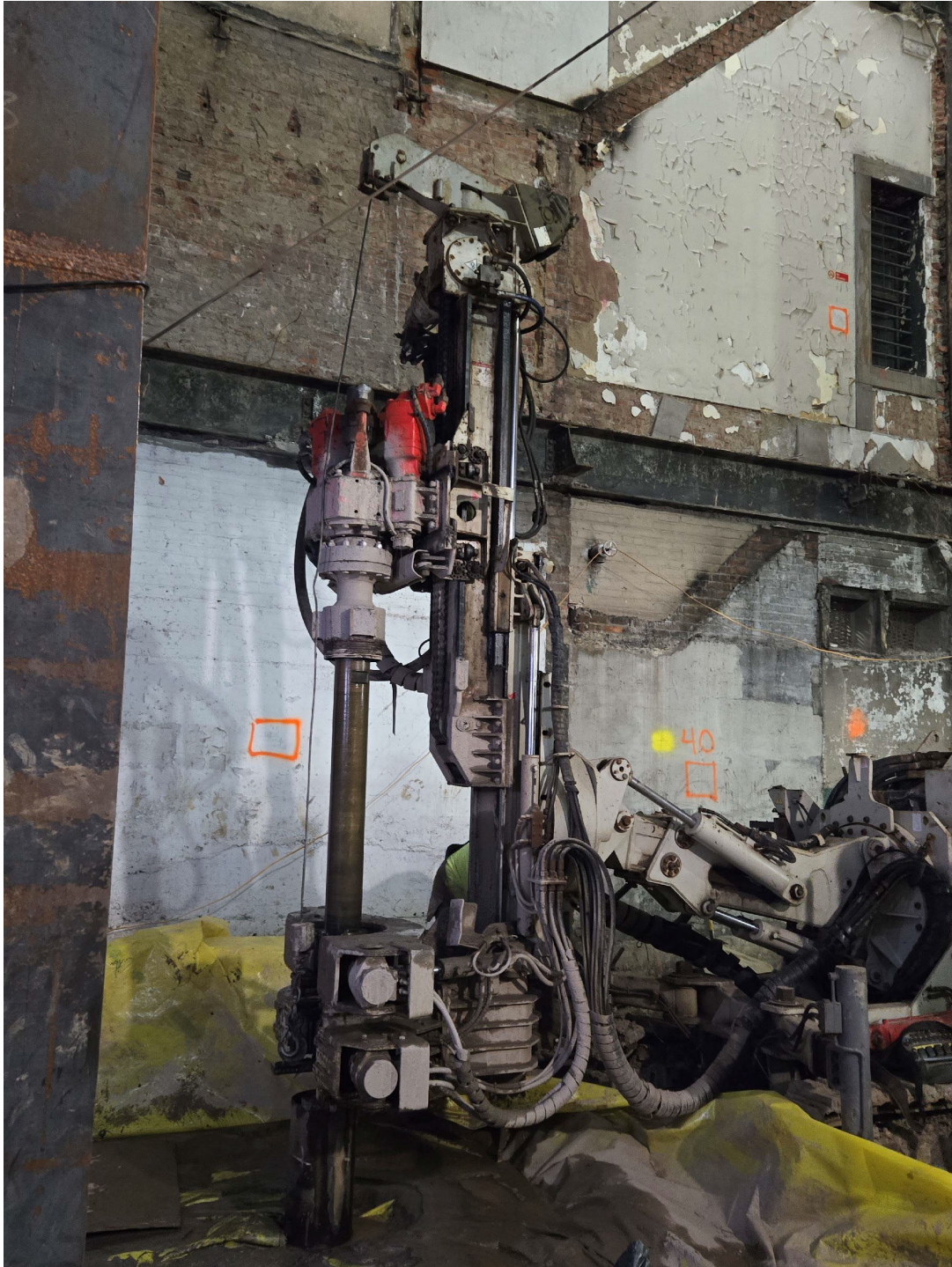
Photo 1: Drilling of Pile #26
