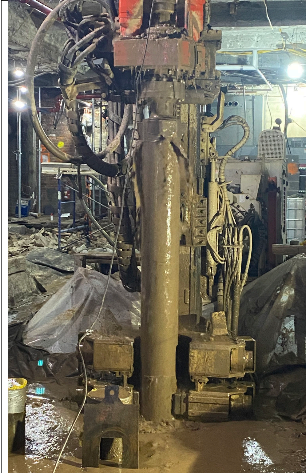
Photo 1: Drilling activities at Pile #21, adjacent to the completed Pile #20.
