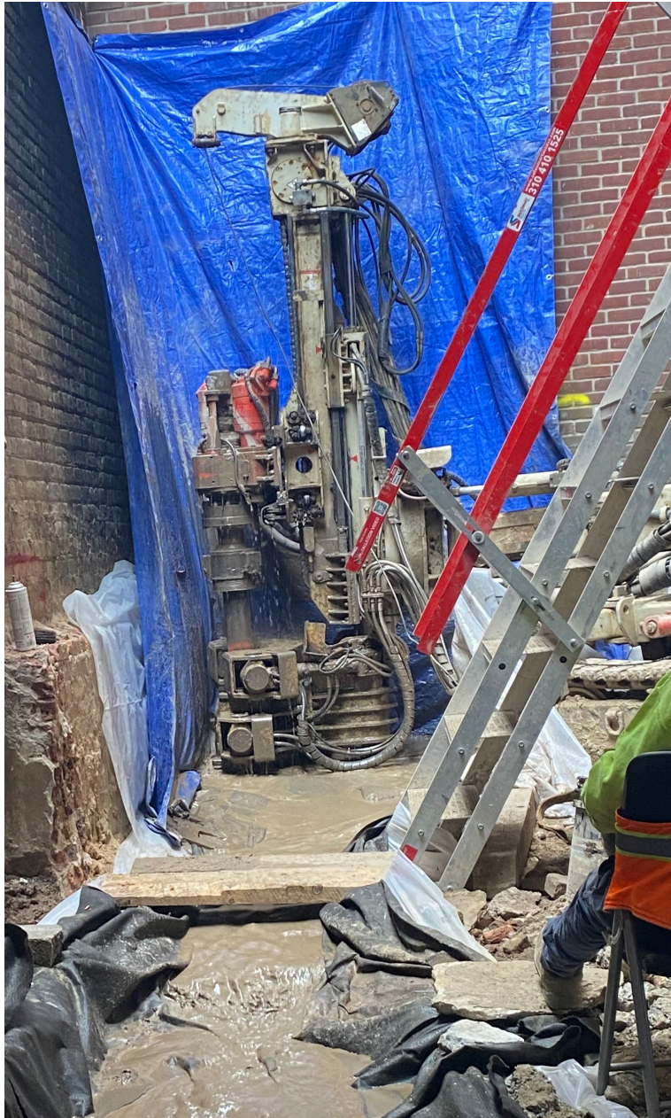
Photo 1: Drilling activities at Pile #4.
