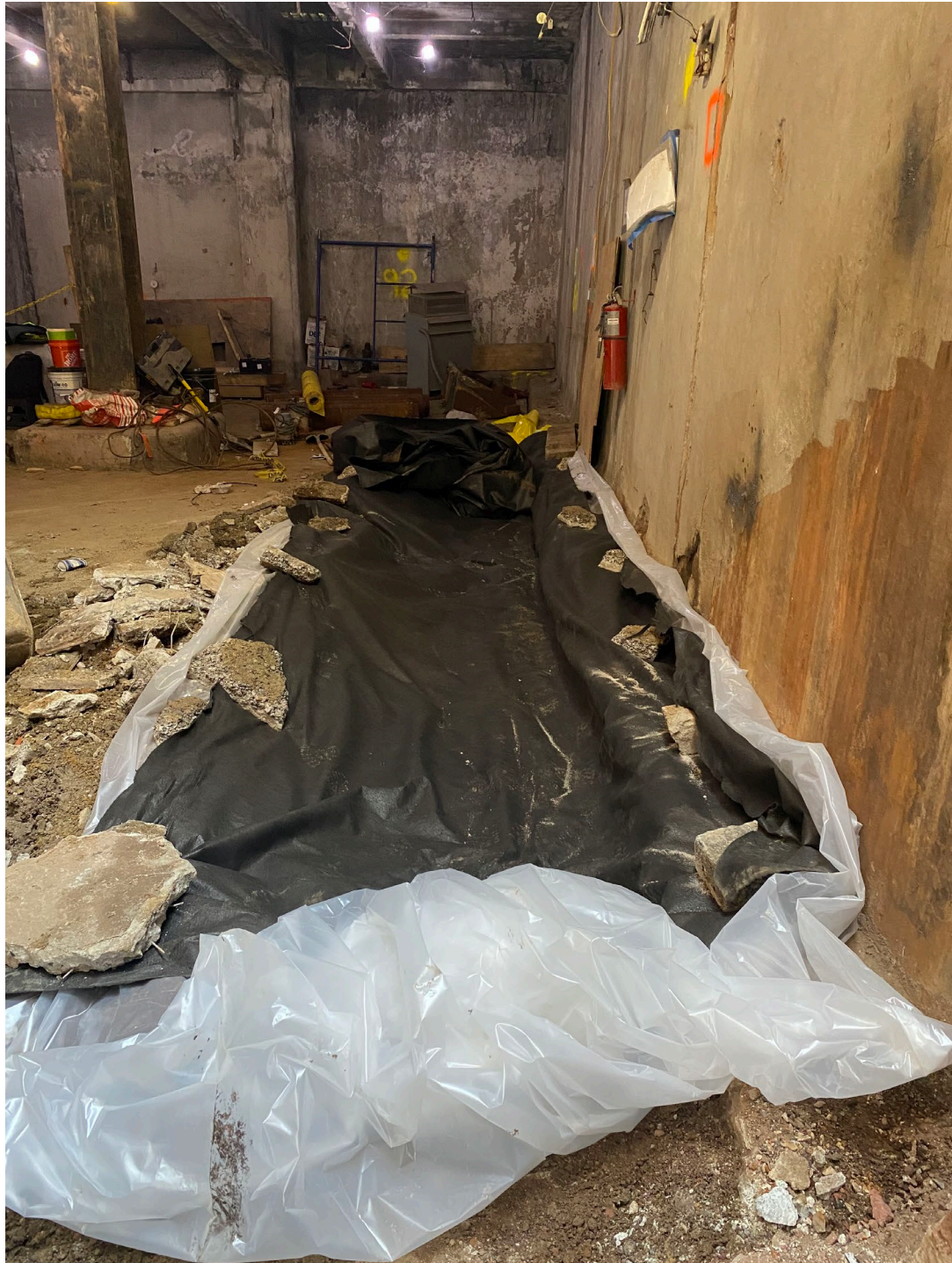
Photo 2: Plastic lining and filter fabric of trench along rear wall of the building
