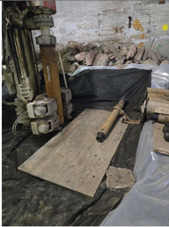
Photo 1: Repositioned plastic sheeting and filter fabric around Pile #20.
