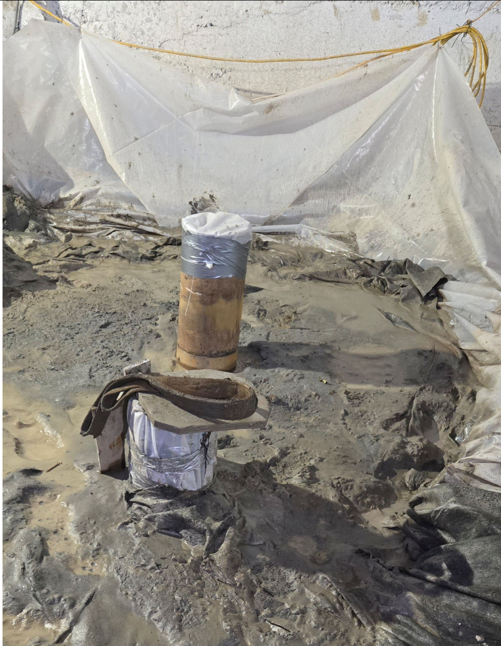
Photo 1: The completed Pile #27 situated behind the previously completed Pile #26.
