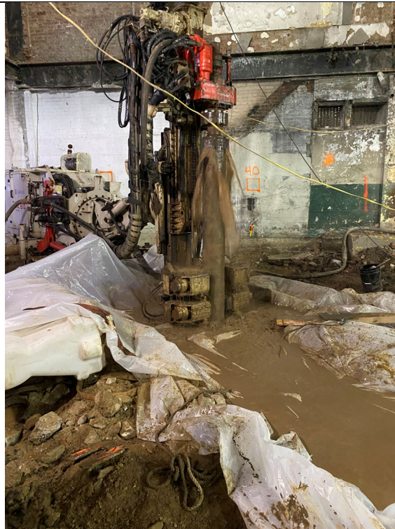
Photo 4: Drilling of Pile #33. Plastic liner is utilized around the drilling location to capture the drill fluid (potable water) for containerization and off-Site disposal.
