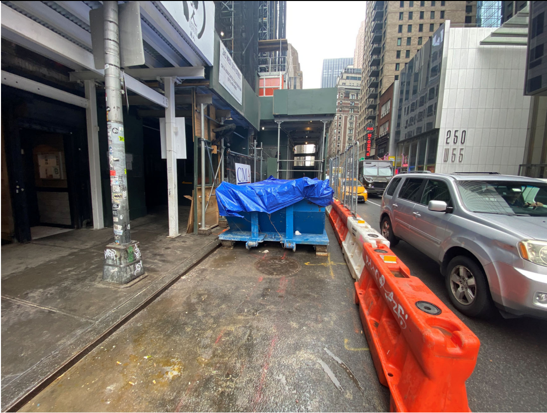
Photo 3: 4,000-gallon tank staged outside the front entrance for drill water.
