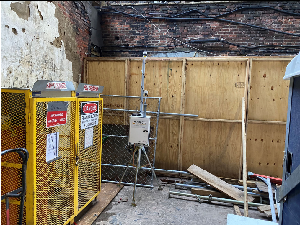
Photo 2: Location of CAMP monitoring station along the back of the building (1 st Floor, NW corner). This location is north of the ramp (former freight elevator) opening to the basement where drilling activities are taking place.
