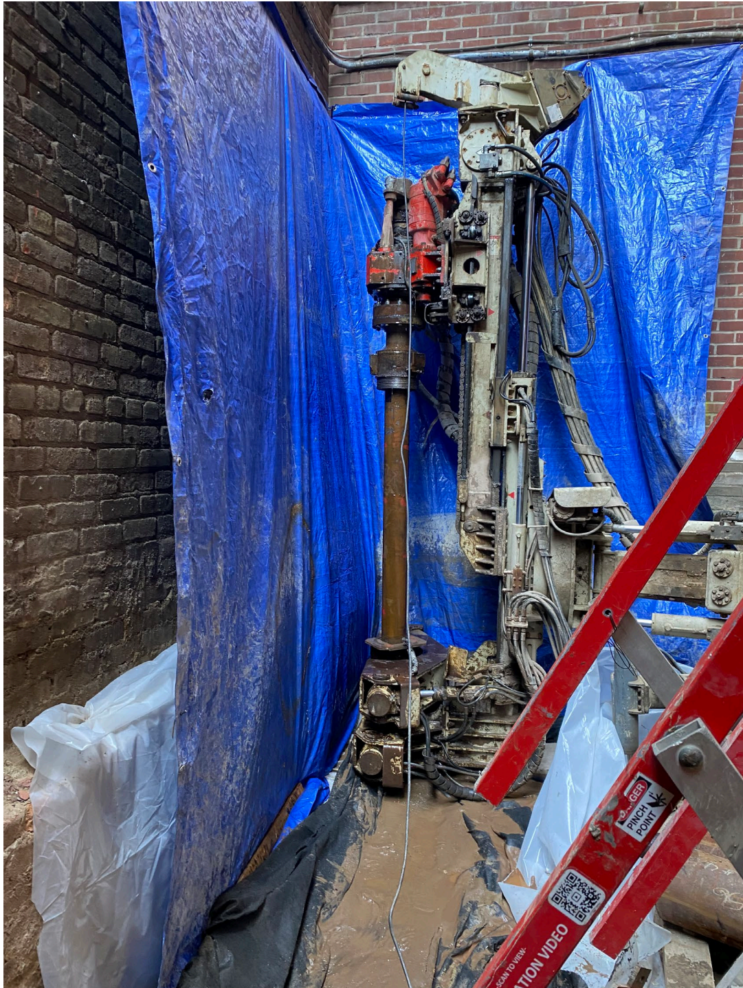
Photo 2: Drilling Activities for Pile #4.
