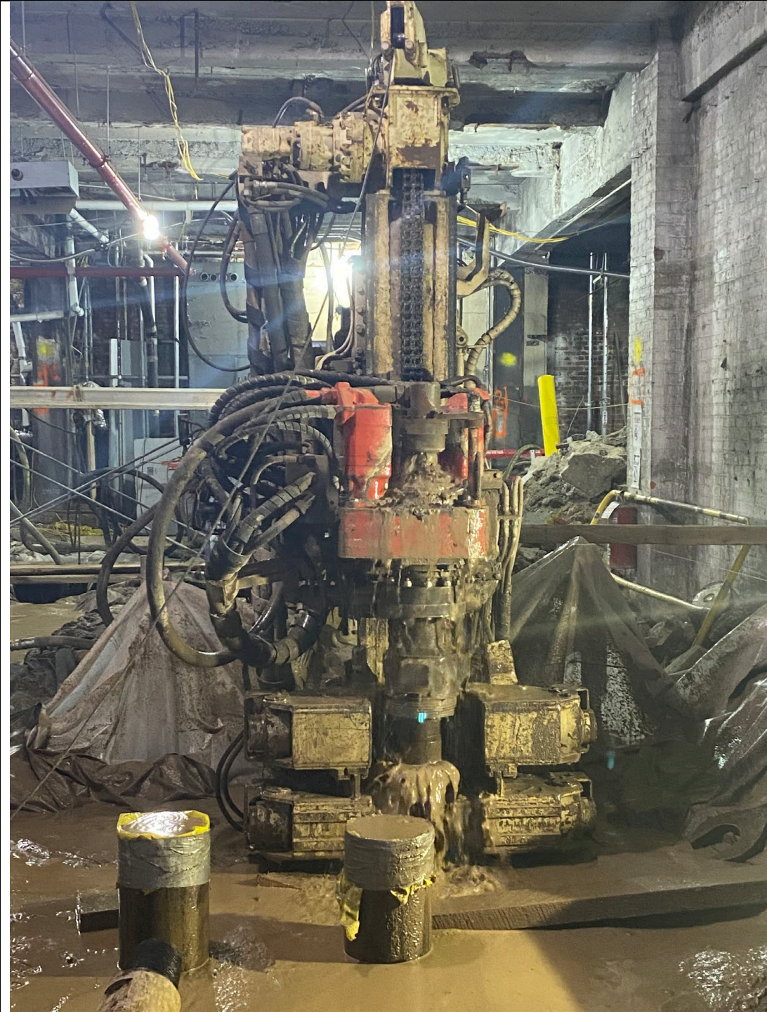
Photo 1: Drilling activities at Pile #22, adjacent to the completed Pile #20.
