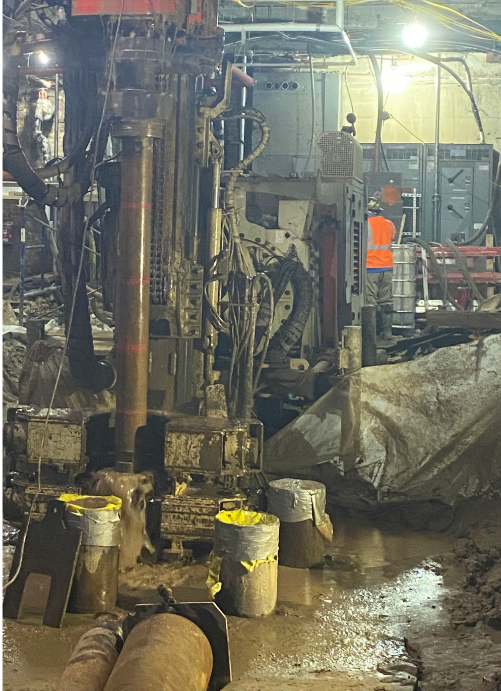
Photo 1: Drilling activities at Pile #23, adjacent to the completed Pile #22. Pile #23 was completed.
