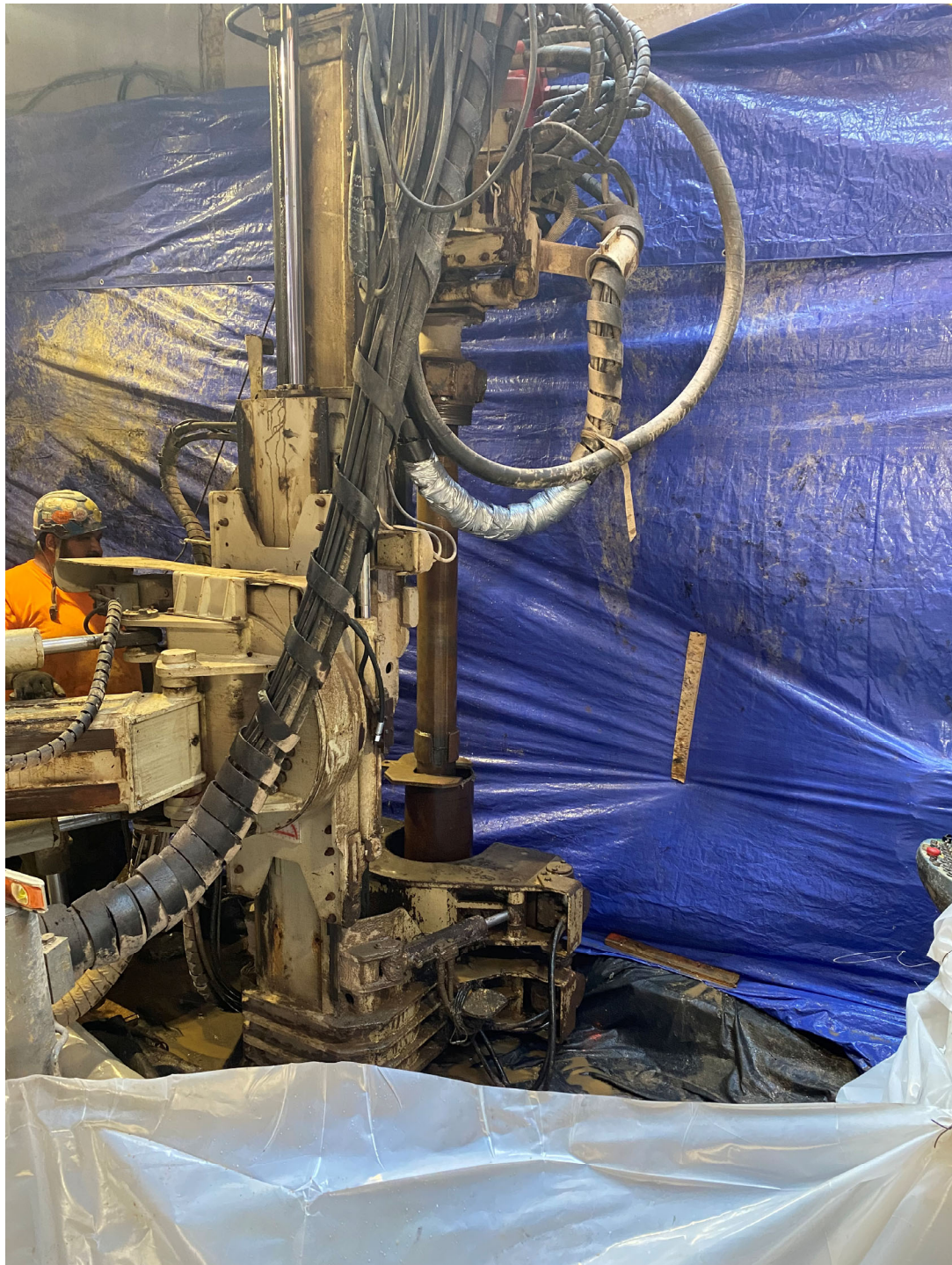
Photo 1: Drilling activities at Pile #3.
