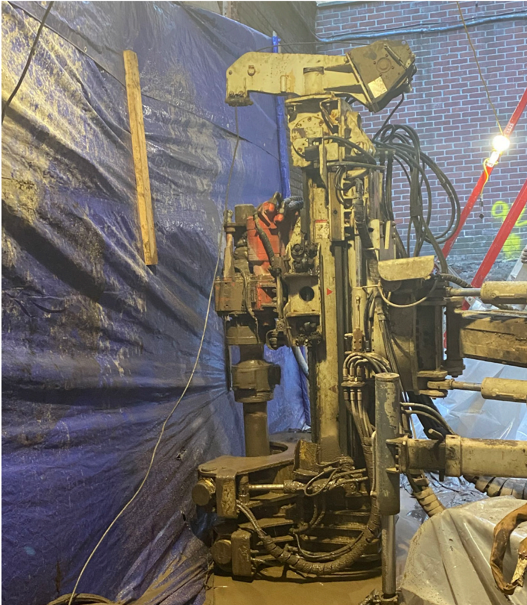
Photo 1: Drilling activities at Pile #3.
