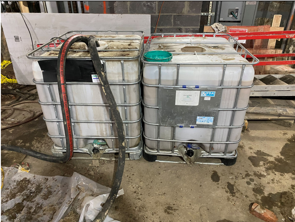
Photo 2: Totes that receive drill water for staging, prior to being conveyed to the 4,000-gallon tank located outside.
