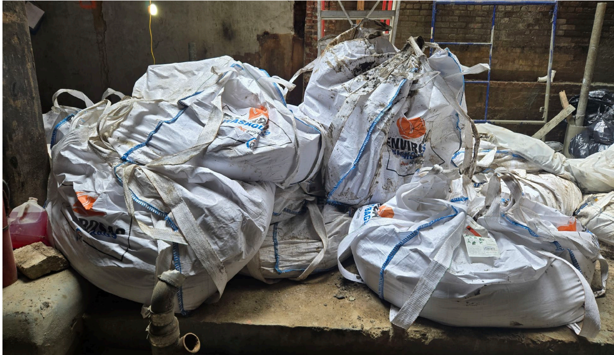
Photo 2: Drill cuttings and basement soils collected in washout bags and staged.
