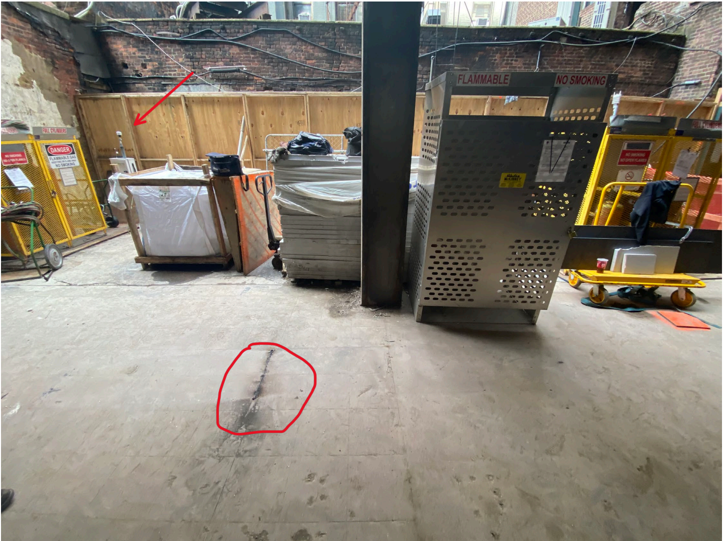
Photo 2: Residual slag on floor where welding triggered exceedance of PM-10 showing proximity to air monitor. Welding activities were relocated to avoid triggering further PM-10 exceedances.
