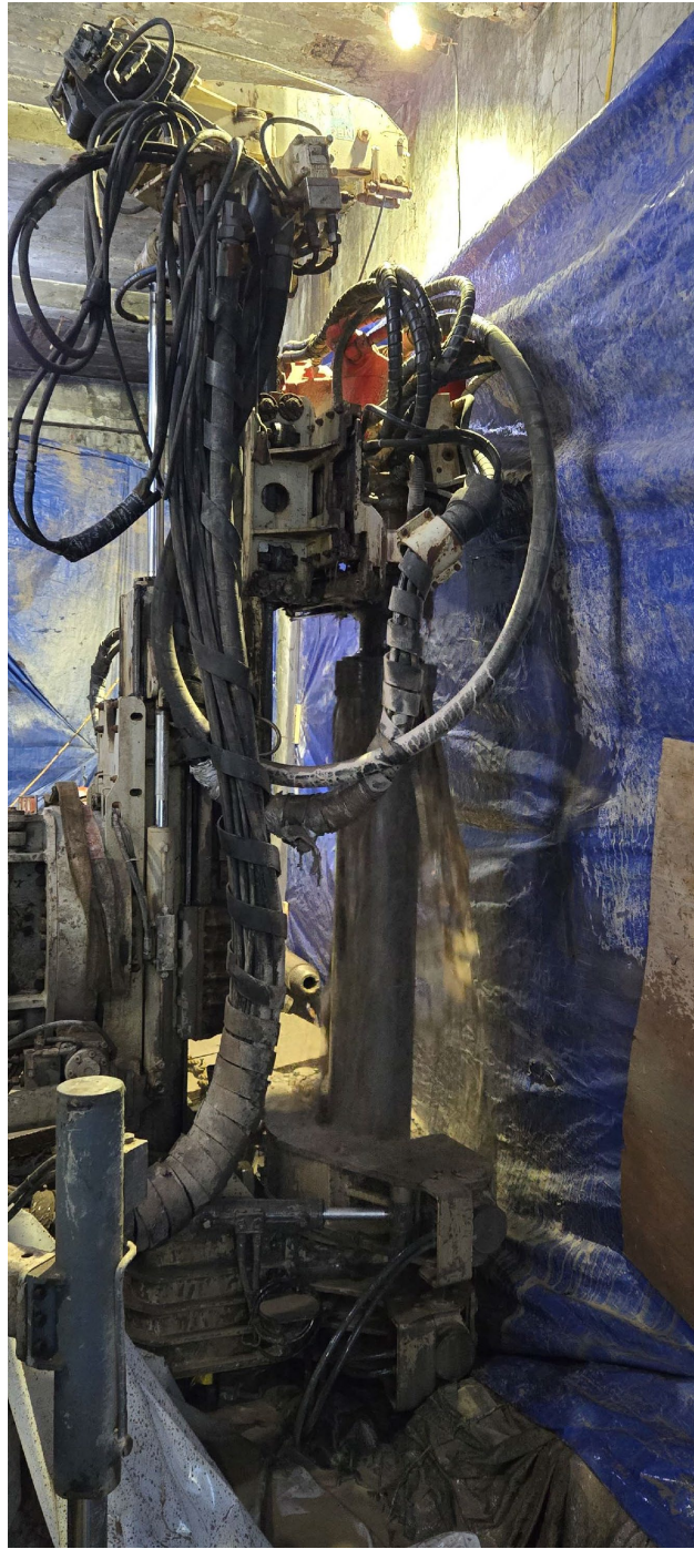
Photo 1: Drill rig set up at Pile #2.
