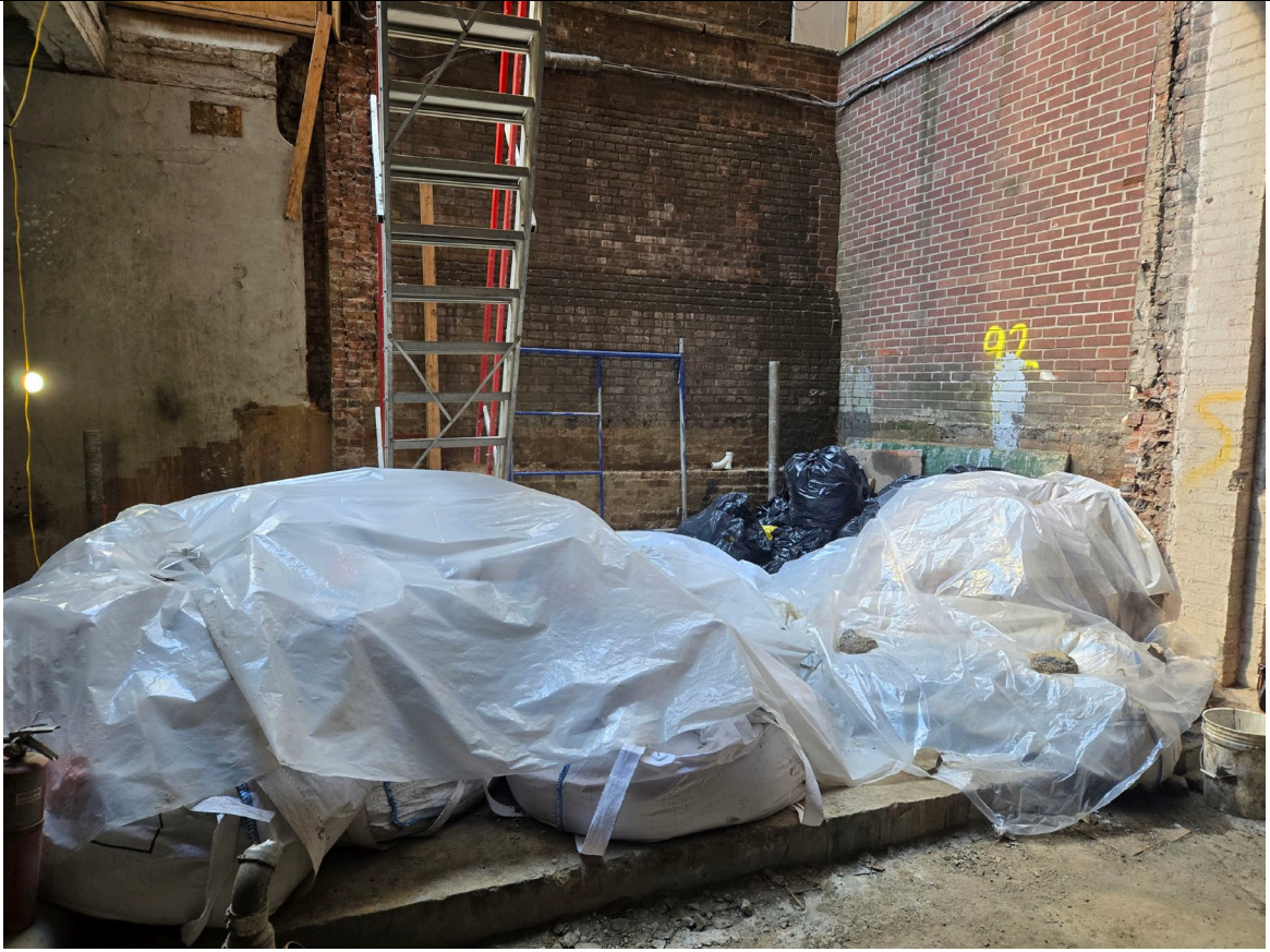
Photo 2: Drill cuttings and basement soils collected in washout bags and staged.
