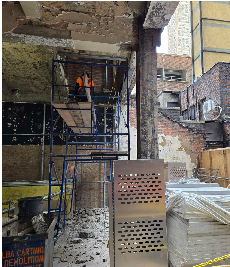
Photo 3: Demolition causing elevated Particulate Matter (PM-10) readings.
