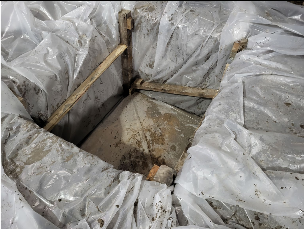
Photo 2: Lining pit with new plastic before drilling of next pile
