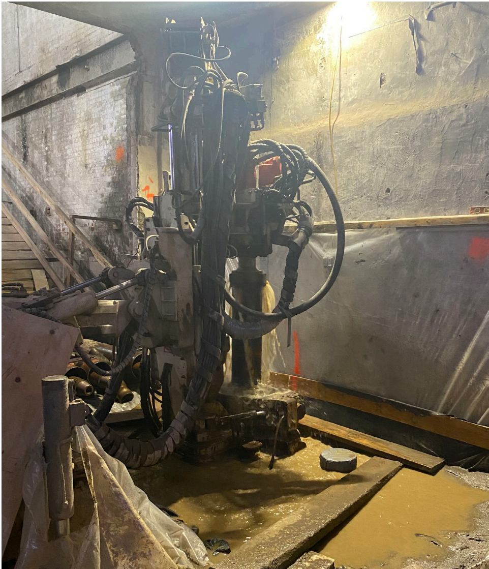
Photo 1: Drilling operations continued at Pile #6, along the west wall of the building.
