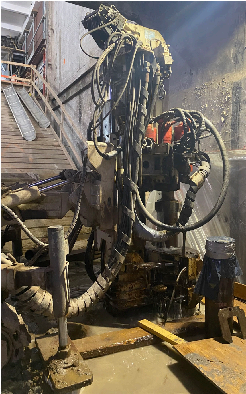
Photo 1: Drilling operations started on Pile #7, along the west wall of the building.
