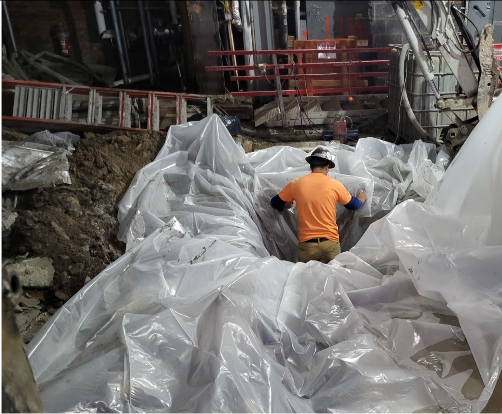
Photo 1: Lining pit with new plastic before drilling of next pile
