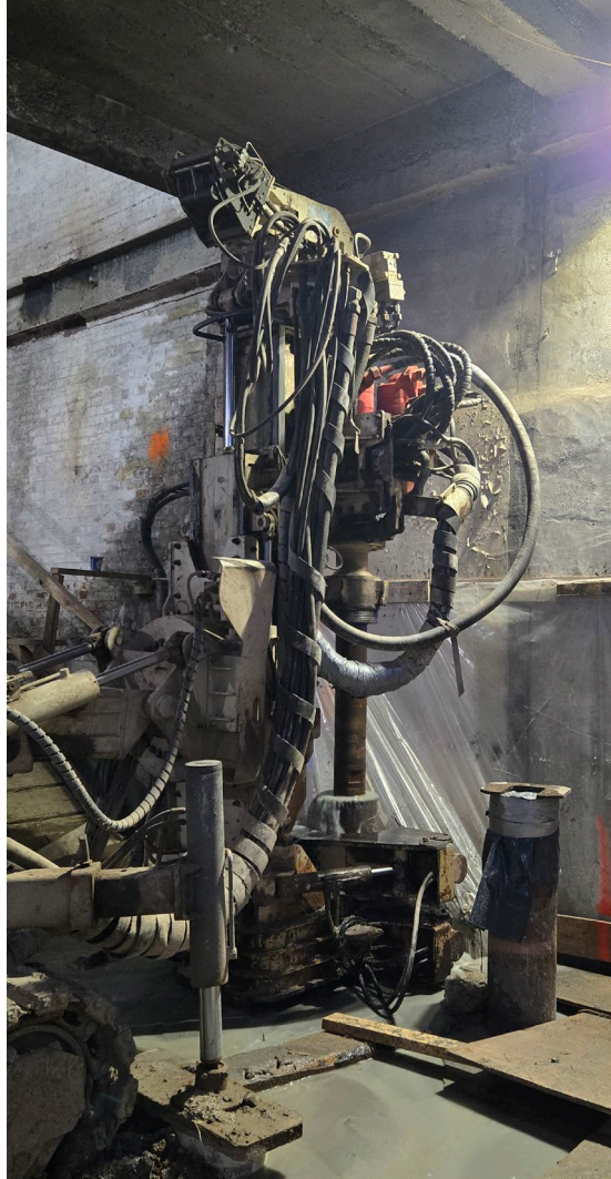
Photo 1: Drilling operations for Pile #7, along the west wall of the building.
