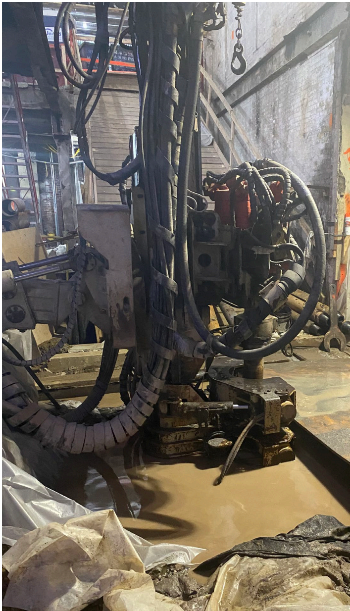
Photo 1: Drilling operations began at Pile #8, along the west wall of the building.
