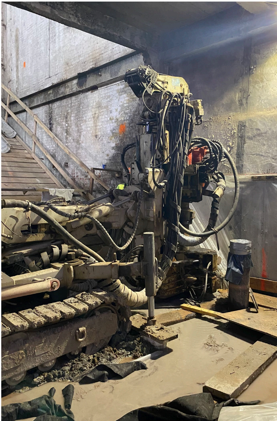
Photo 1: Drilling operations started on Pile #7, along the west wall of the building.
