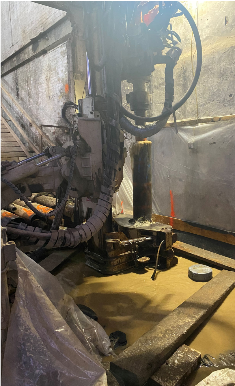
Photo 1: Drilling operations continued at Pile #6, along the west wall of the building.
