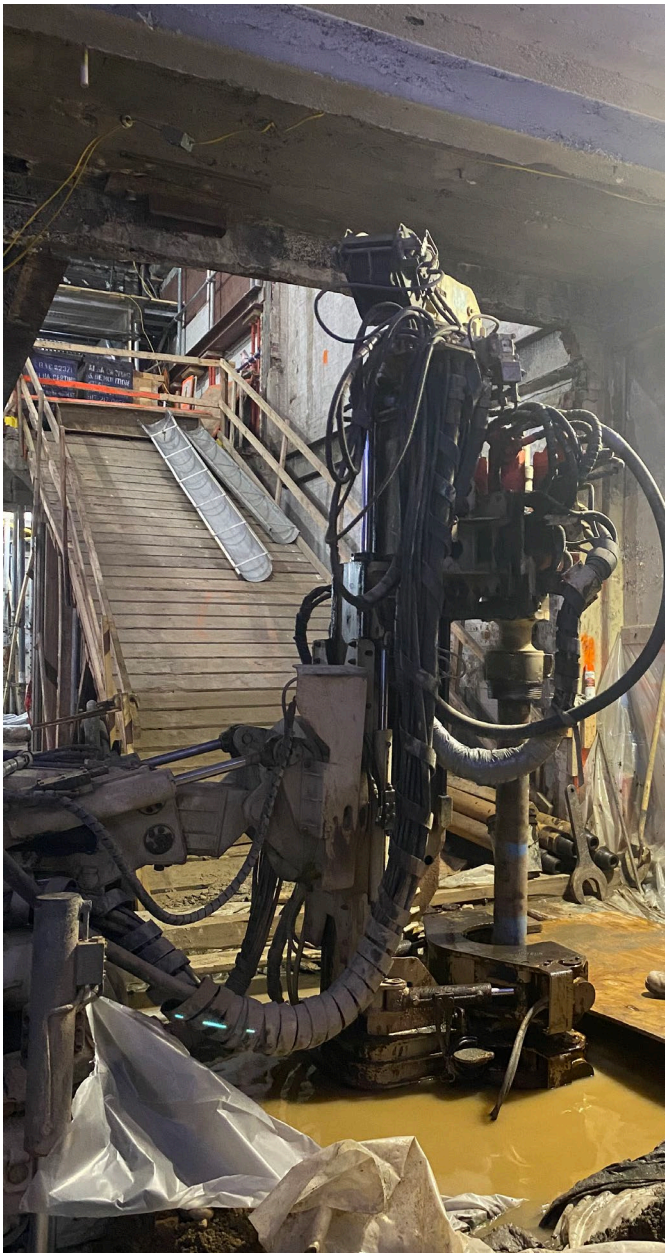
Photo 1: Drilling operations continued and were completed at Pile #8, along the west wall of the building.
