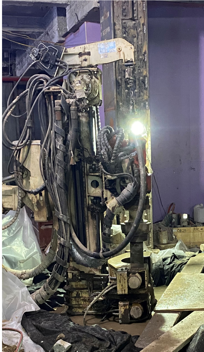
Photo 1: Drilling operations for Pile #24.
