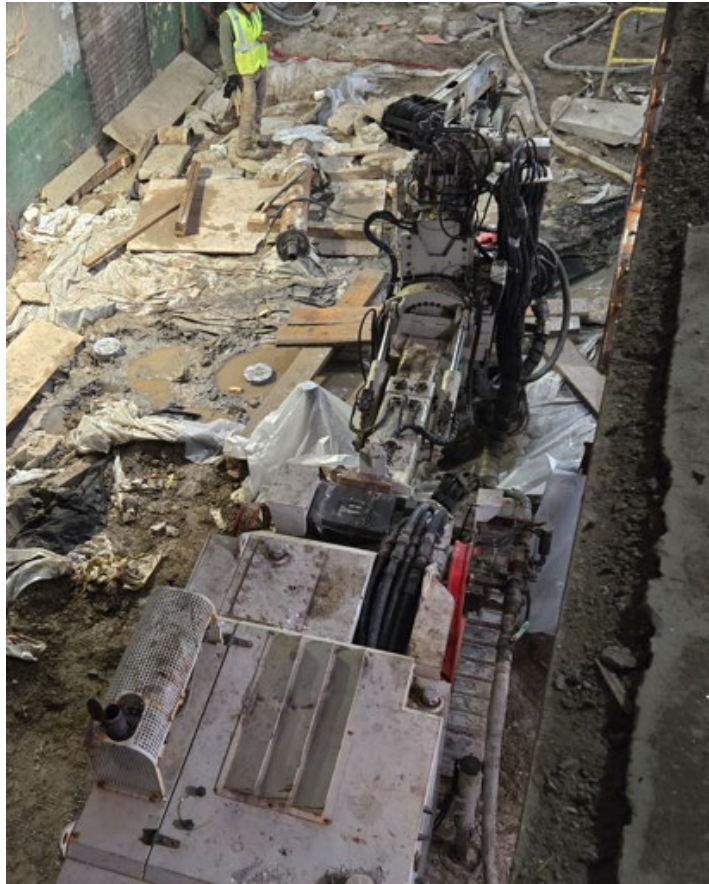
Photo 1: View of drill rig from first floor of building starting SOE pile 52. Completed SOE piles 53 and 54 shown to left of drill rig.
