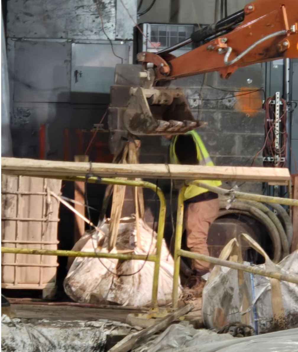
Photo 1: Drill cuttings being loaded into washout bags for disposal
