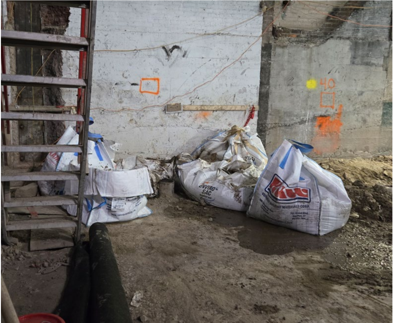
Photo 2: Washout bags with drill cuttings for disposal
