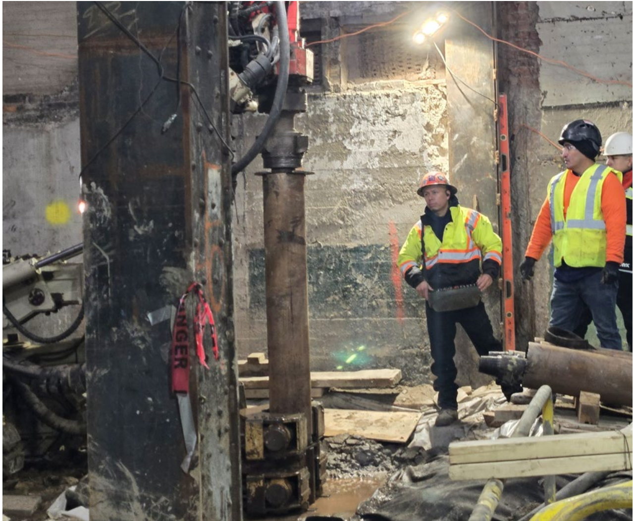
Photo 2: Drilling activities on SOE Pile #53
