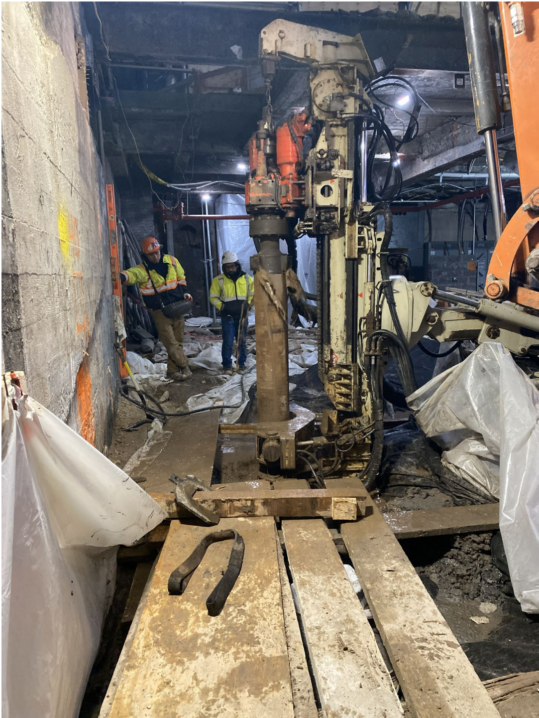
Photo 1: Drilling activities at SOE Pile #55
