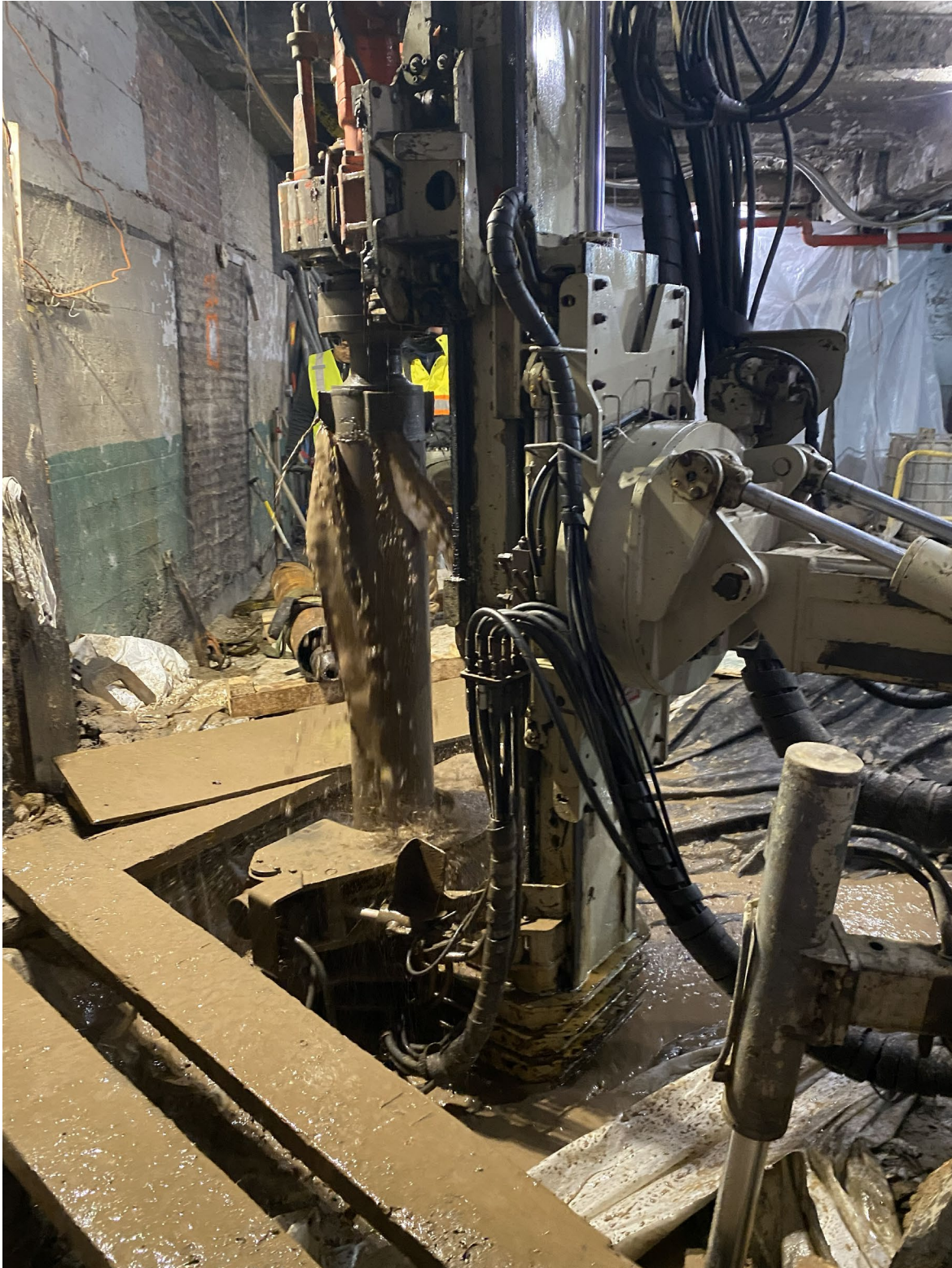
Photo 2: Drilling activities were started but not completed on SOE Pile #54
