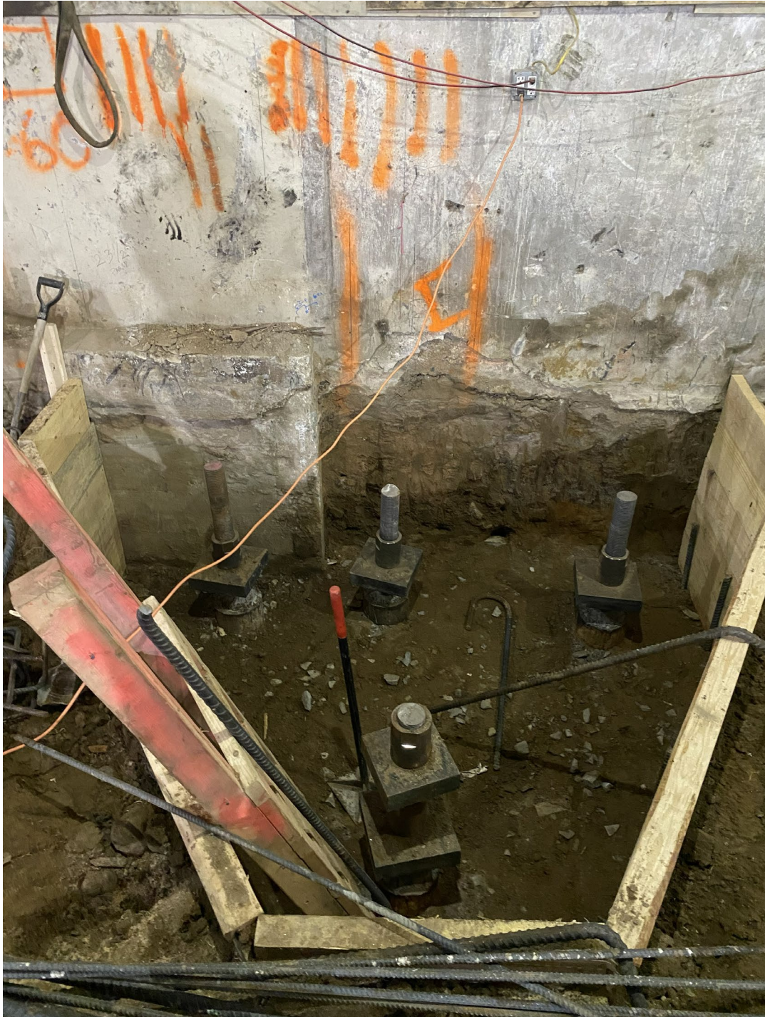
Photo 2: Forms installed at pile cap location PC-4ANW.
