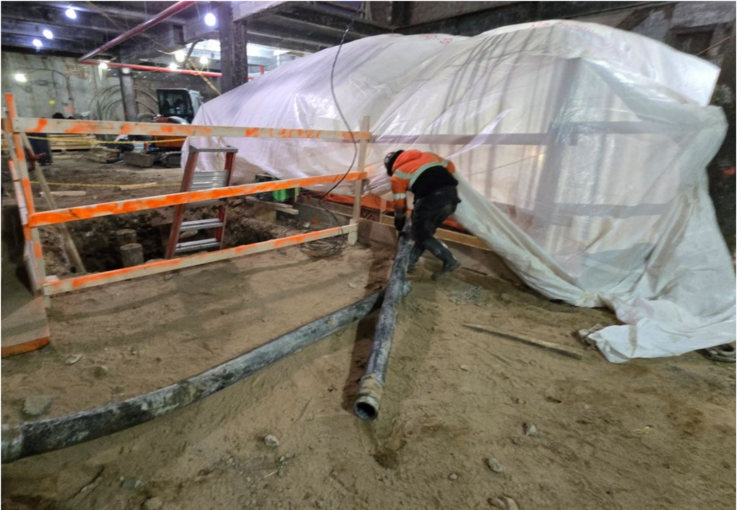
Photo 1: Concrete pouring continued into RO1A.
