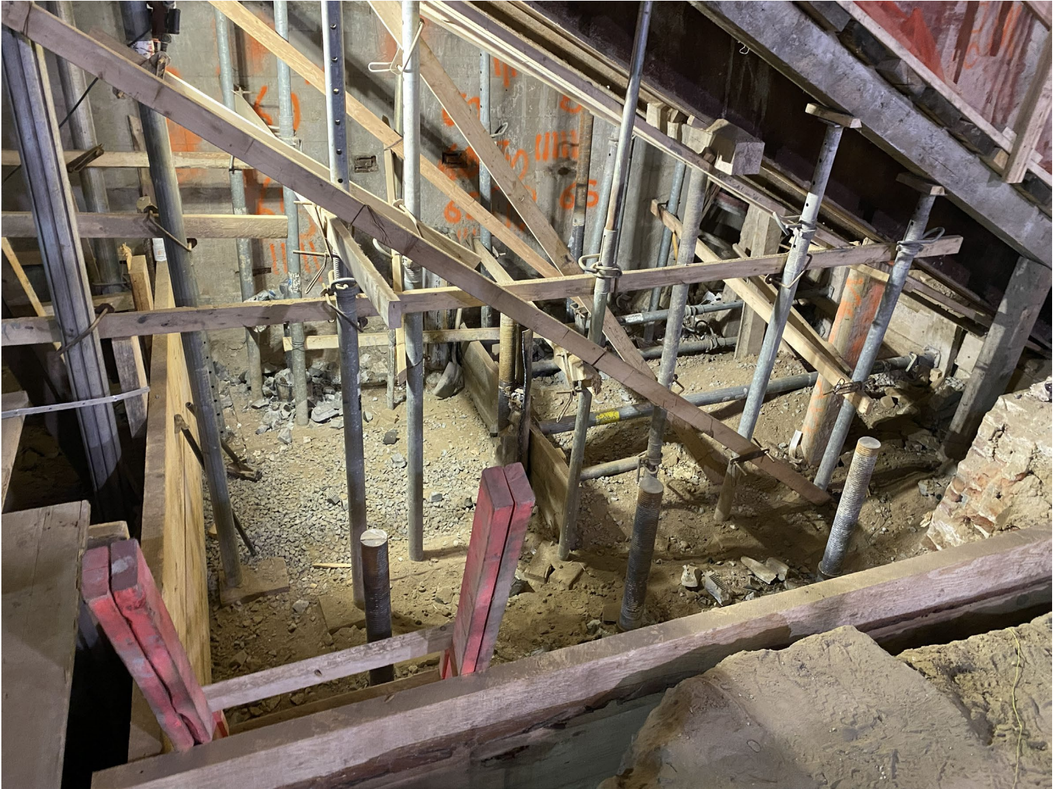
Photo 1: Preparation of the RO1 pile cap continued.
