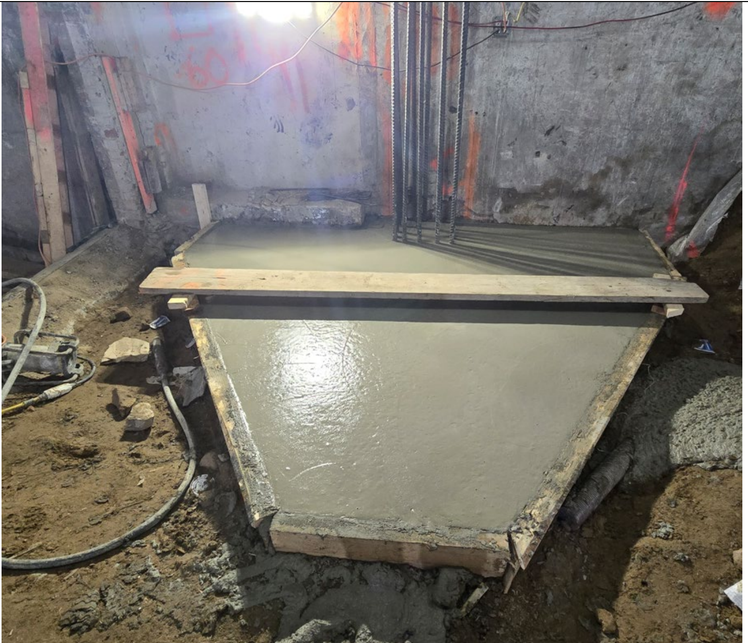
Photo 2: Concrete pouring was completed at location PC-4ANW.
