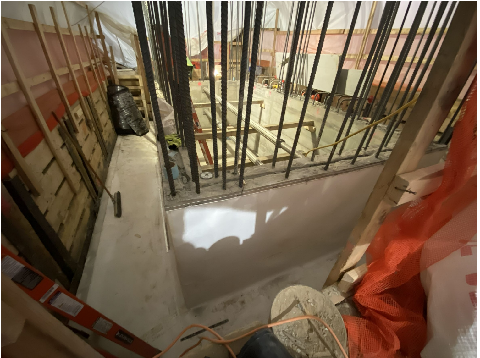
Photo 4: Water proofing layer installed in RO1A
