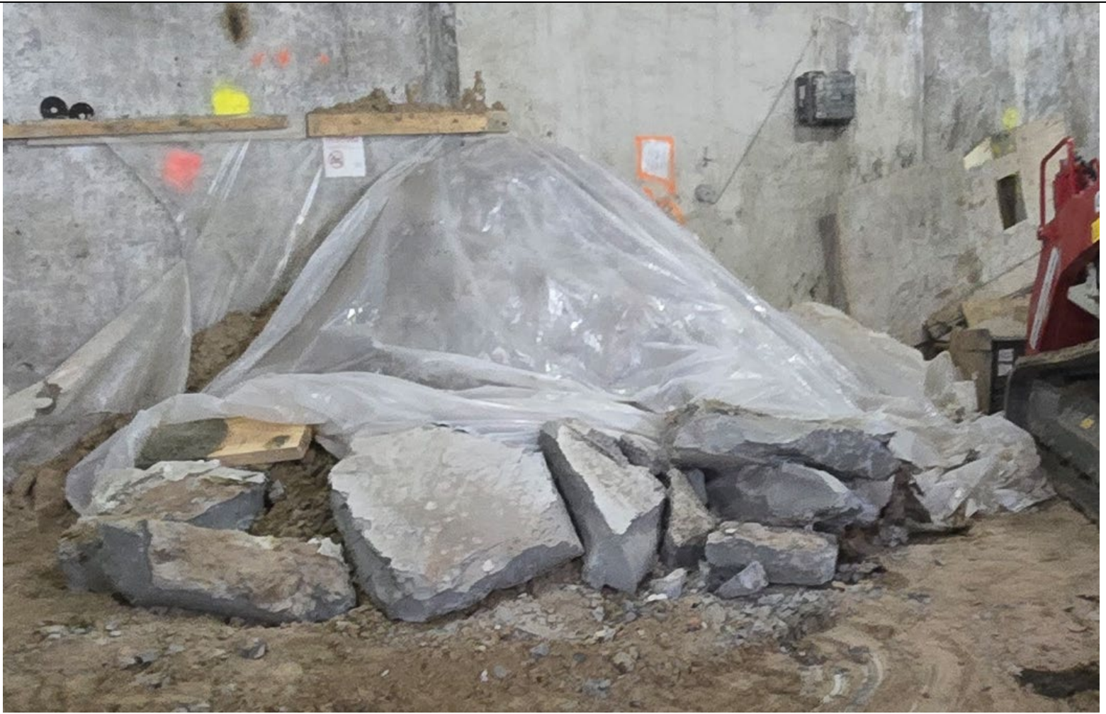
Photo 2: Soil stockpile covered with plastic.
