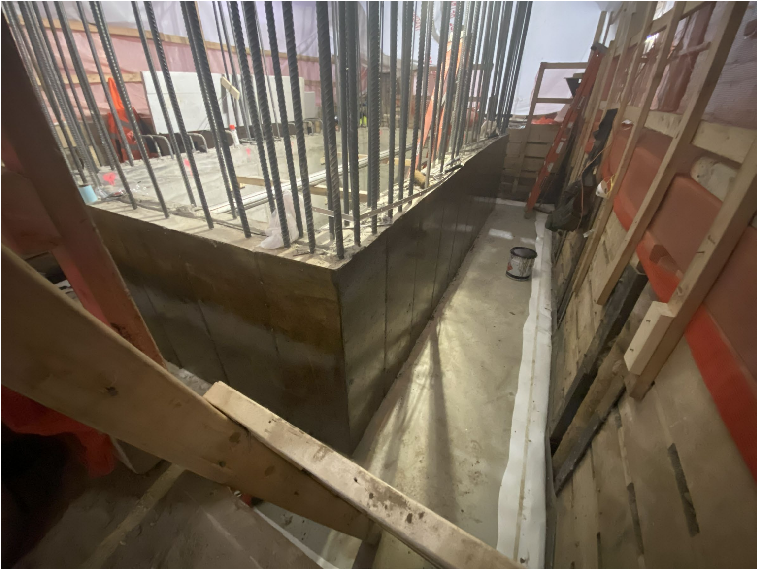
Photo 4: Water proofing layer installed in RO1A
