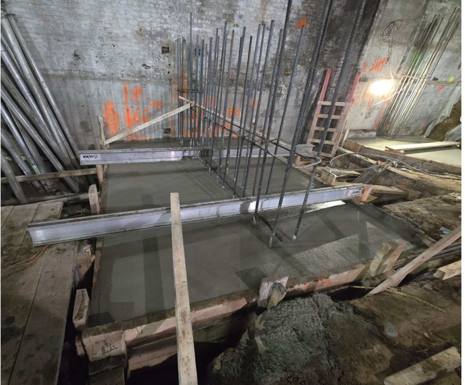
Photo 1: Concrete pouring was completed at location RO1.
