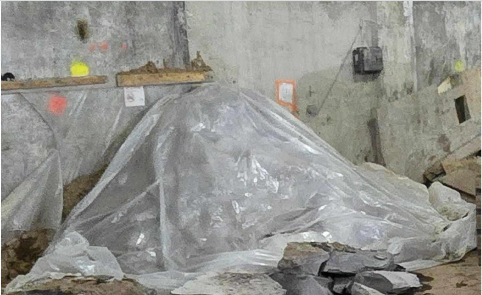
Photo 2: Soil stockpile covered with plastic.
