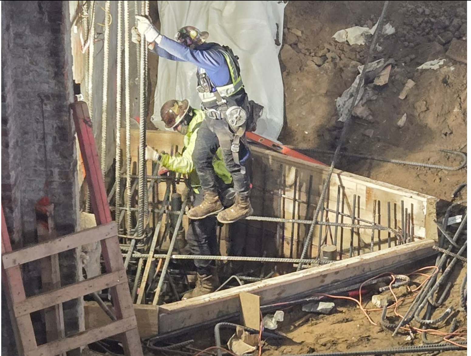
Photo 2: Rebar installation at pile cap location PC-4ANW.
