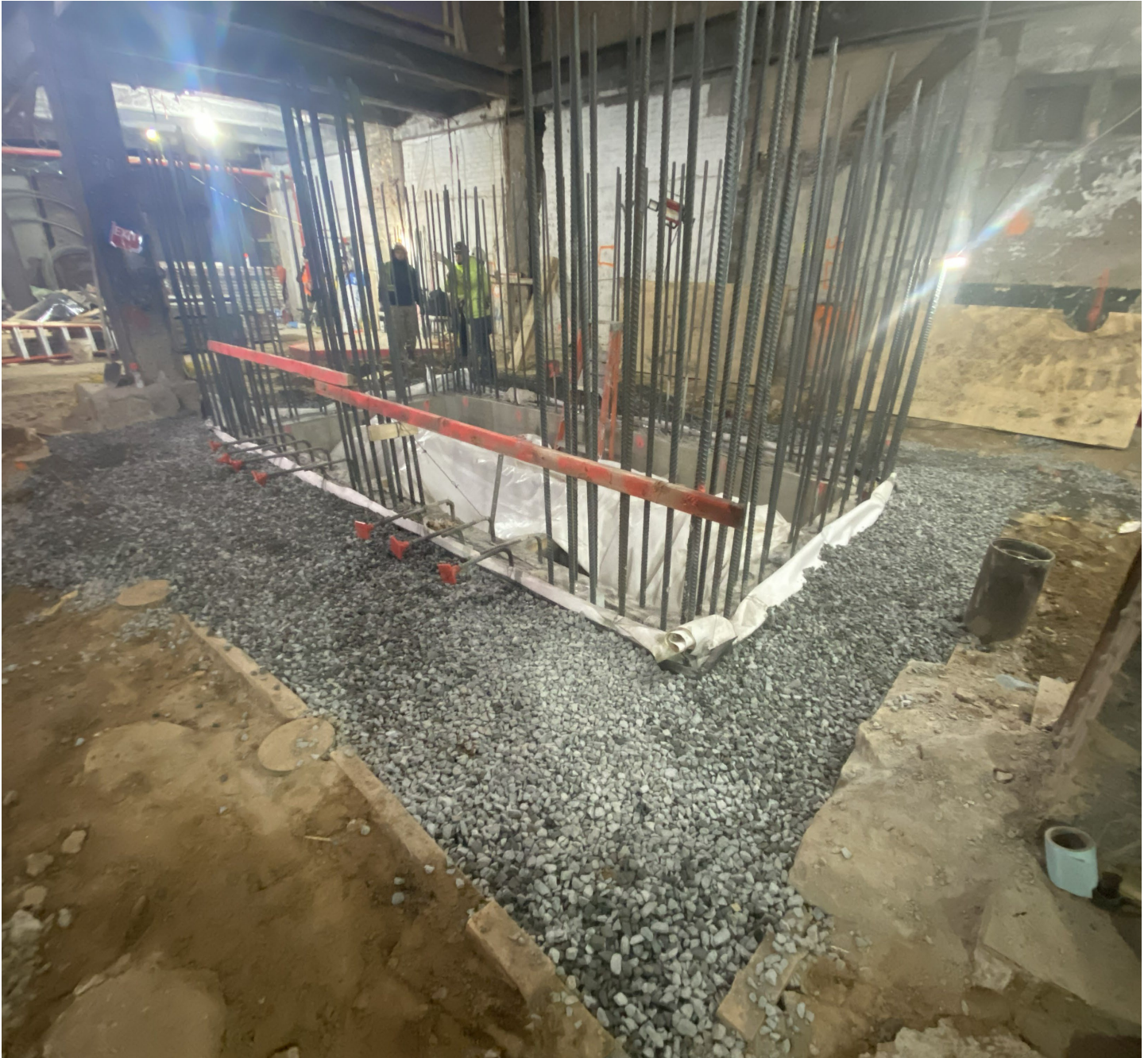
Photo 3: Stone installed at the new elevator pit area (RO1A)
