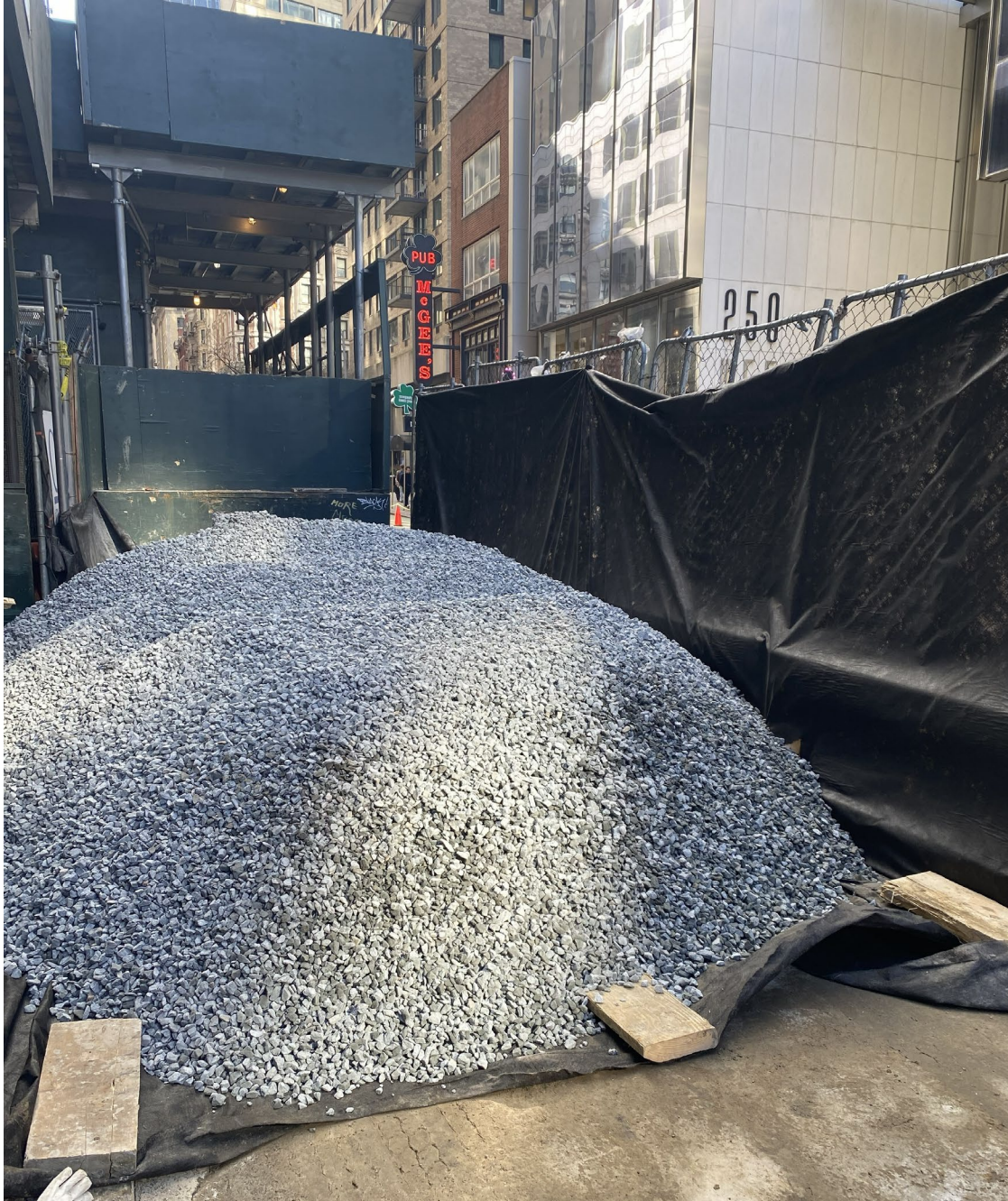
Photo 2: Stone (ASTM #5) delivered to the site
