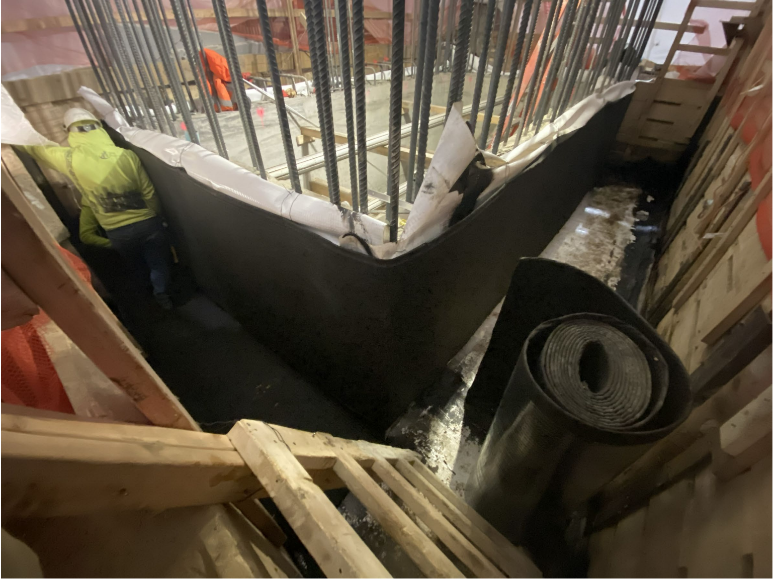
Photo 3: Installation of drainage mats
