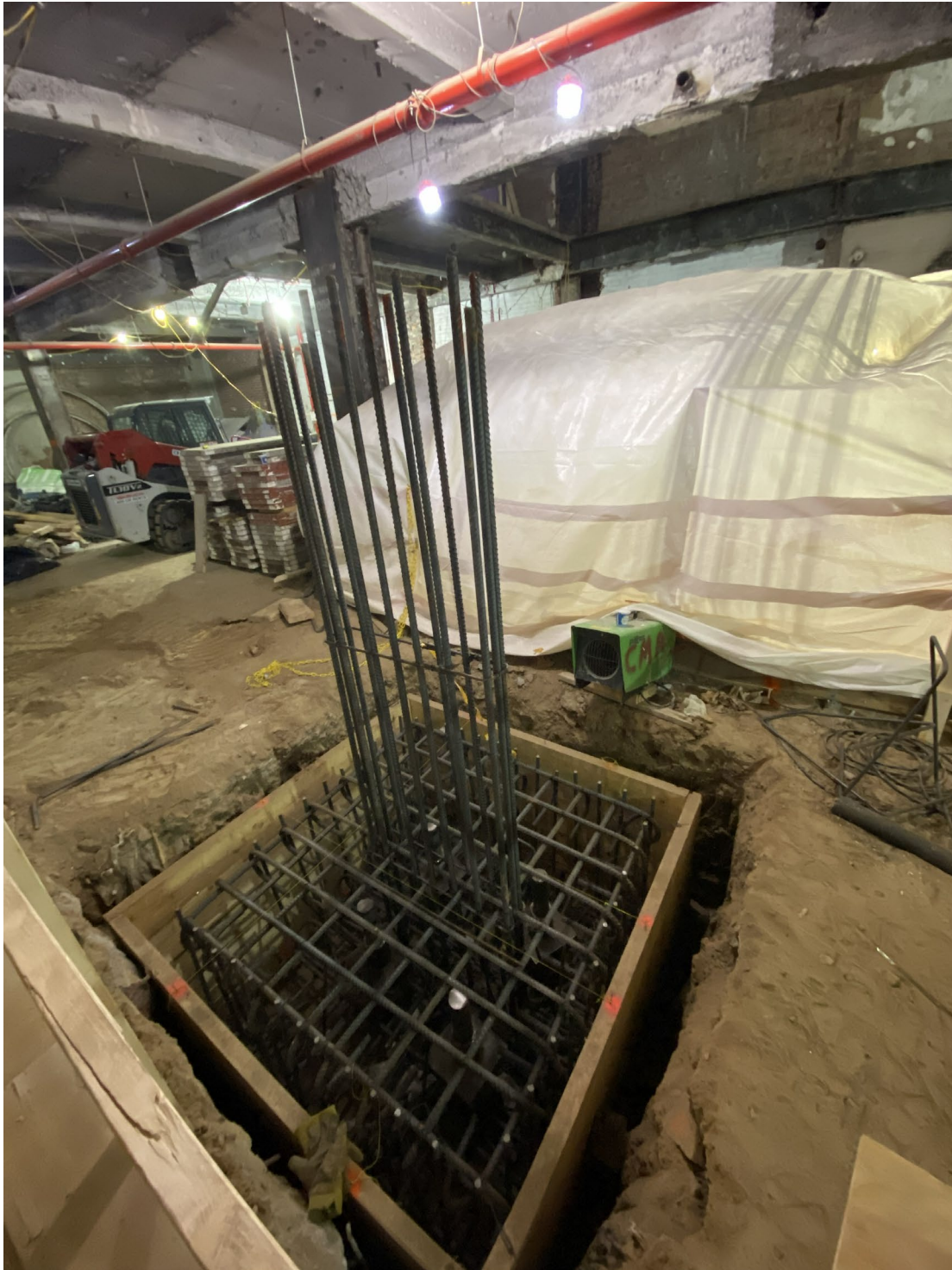
Photo 2: Rebar install continued at PC-4
