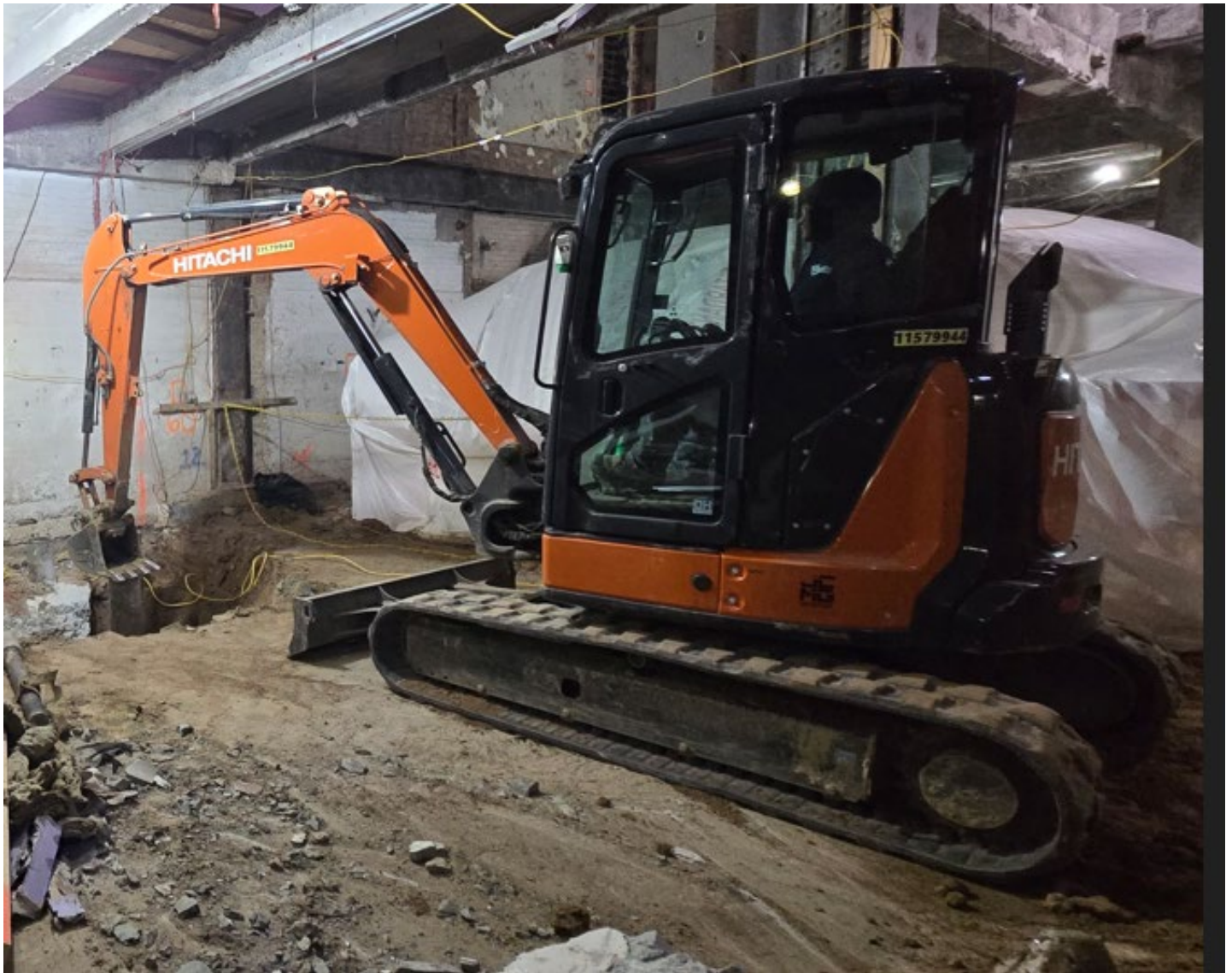
Photo 1: Excavation of PC-4ANE continues
