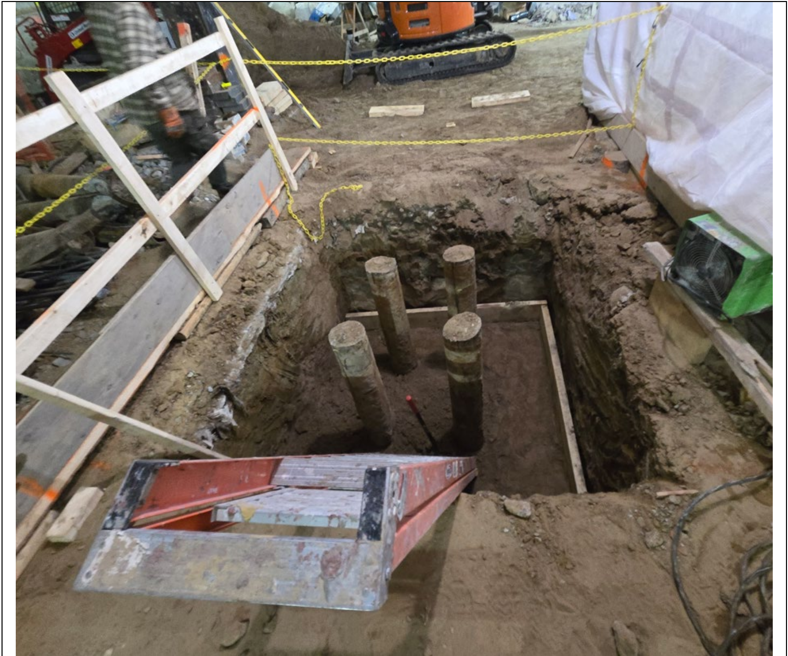
Photo 1: Excavation of PC-4.
