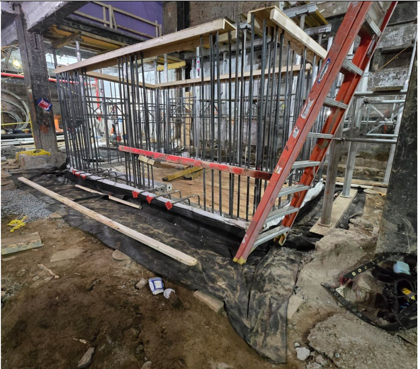
Photo 3: Preparation for installation of concrete forms at RO1A continued.
