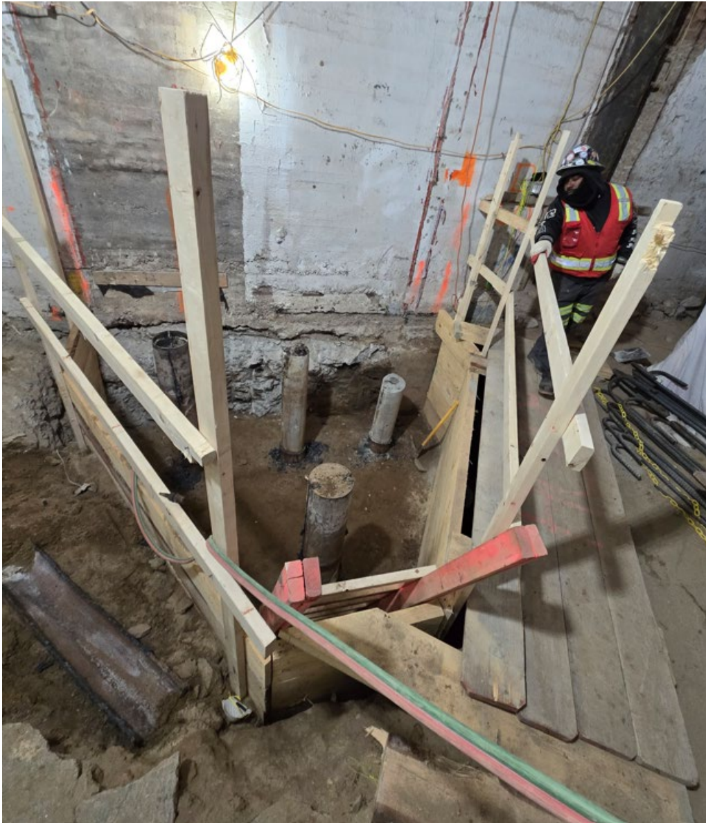
Photo 1: Excavation of PC-4ANE completed.
