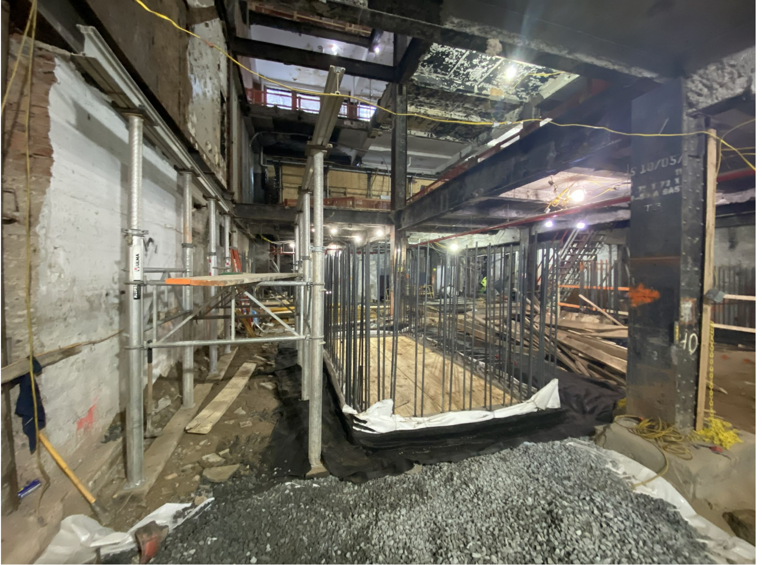
Photo 3: Preparation for pouring concrete at RO1A
