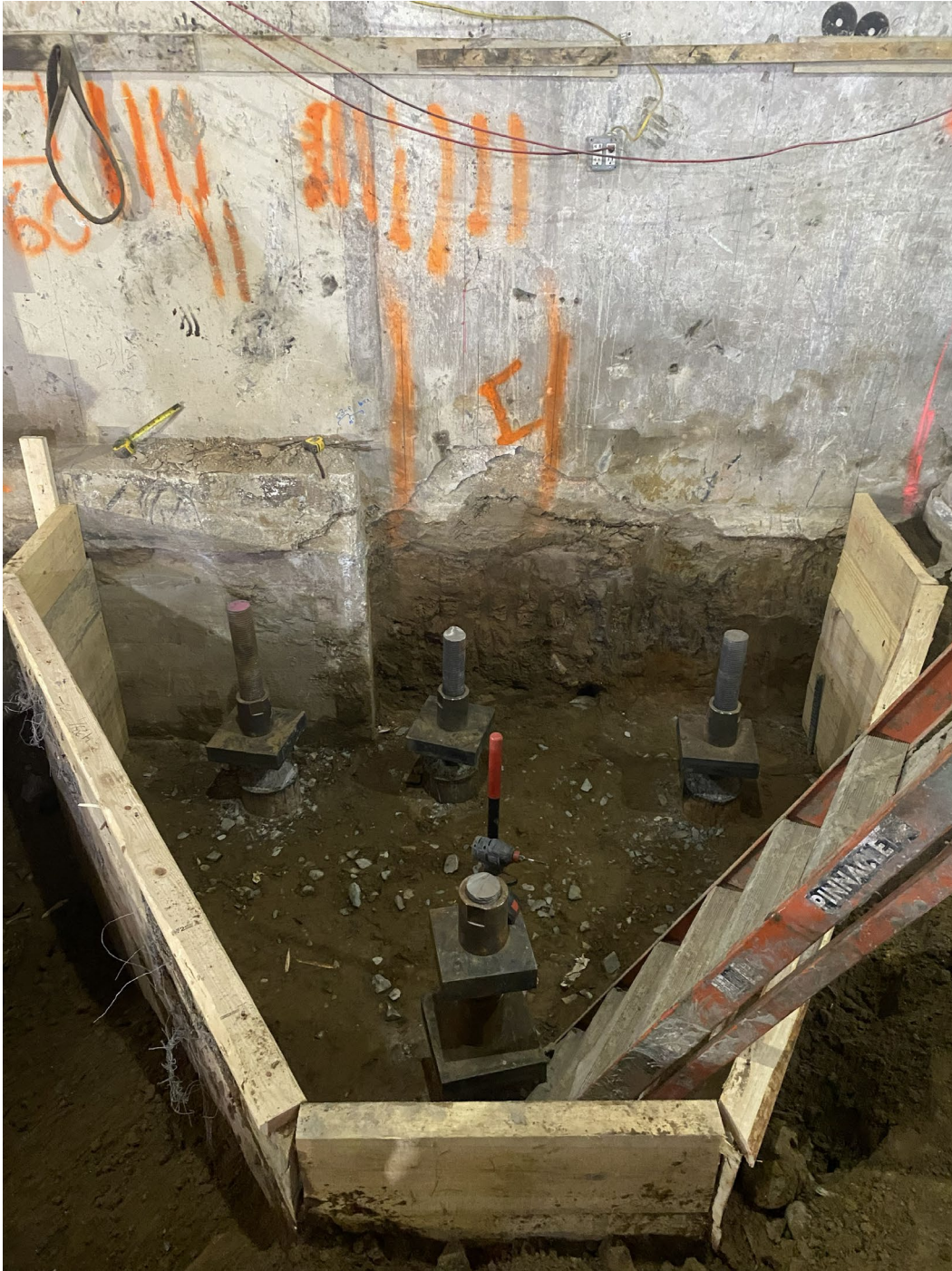
Photo 2: Forms installed at pile cap location PC-4ANW.
