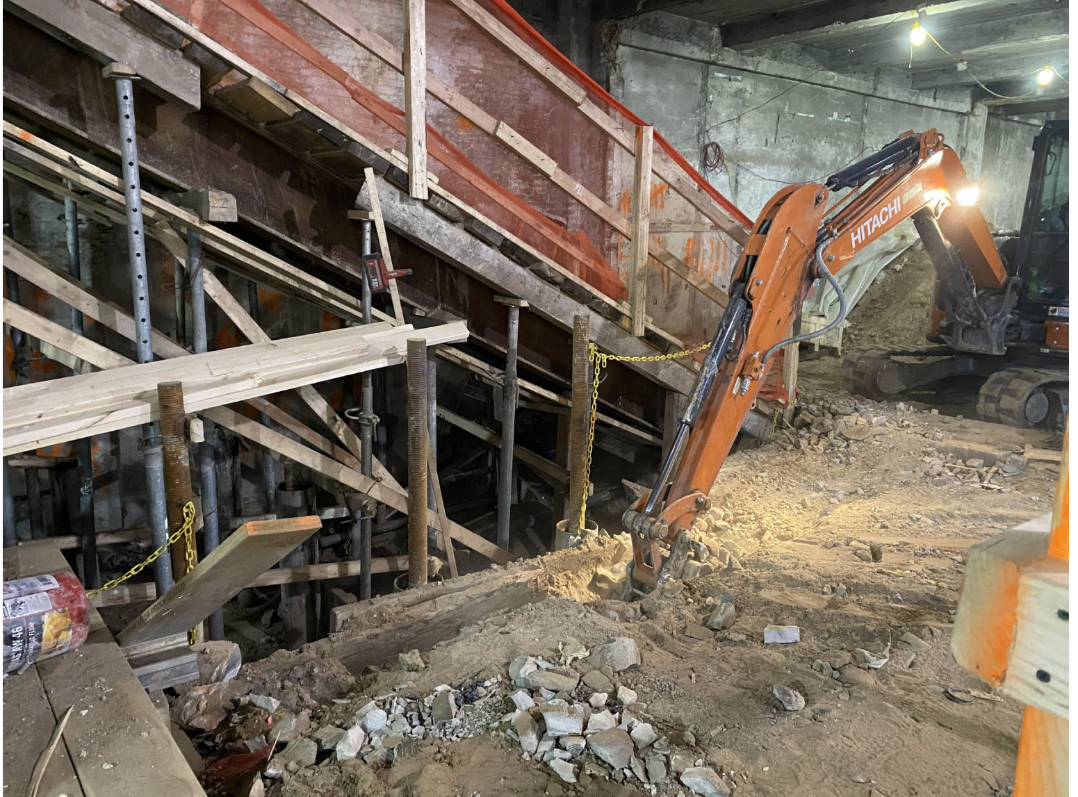
Photo 1: Removal of the Former Elevator Pit (RO1) wall.
