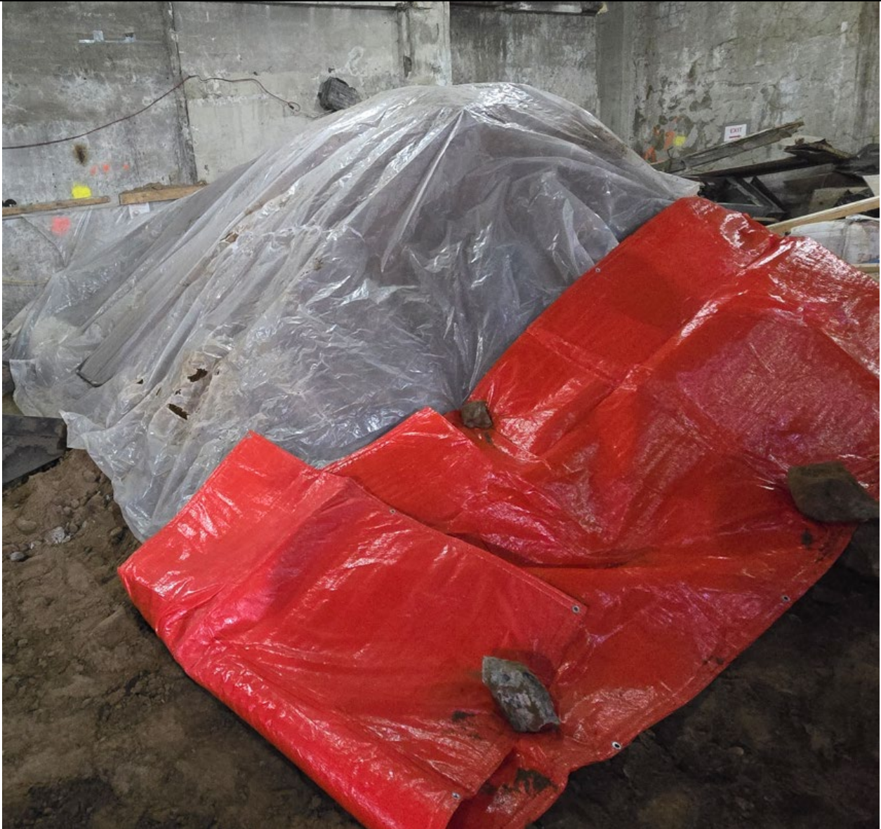
Photo 3: Soil stockpile in basement covered in poly sheeting and tarp.
