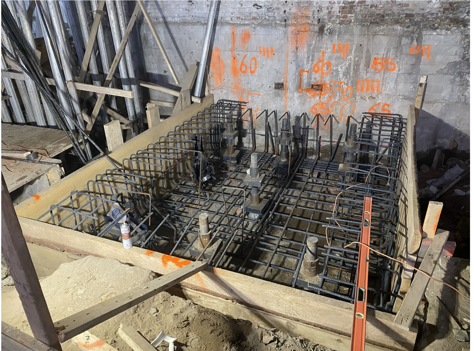
Photo 1: Preparation of the RO1 pile cap continued.
