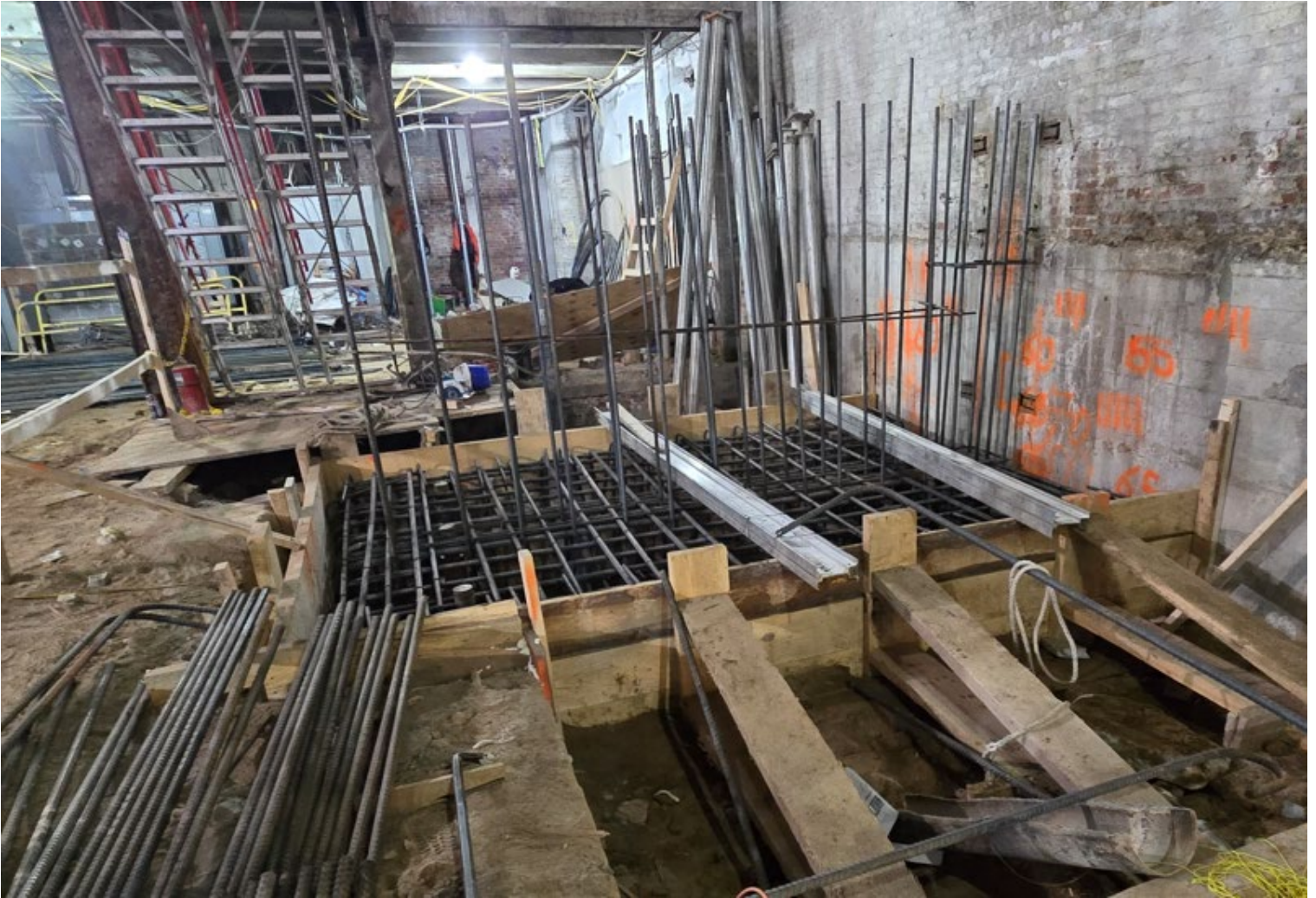
Photo 1: Installation of rebar at RO1
