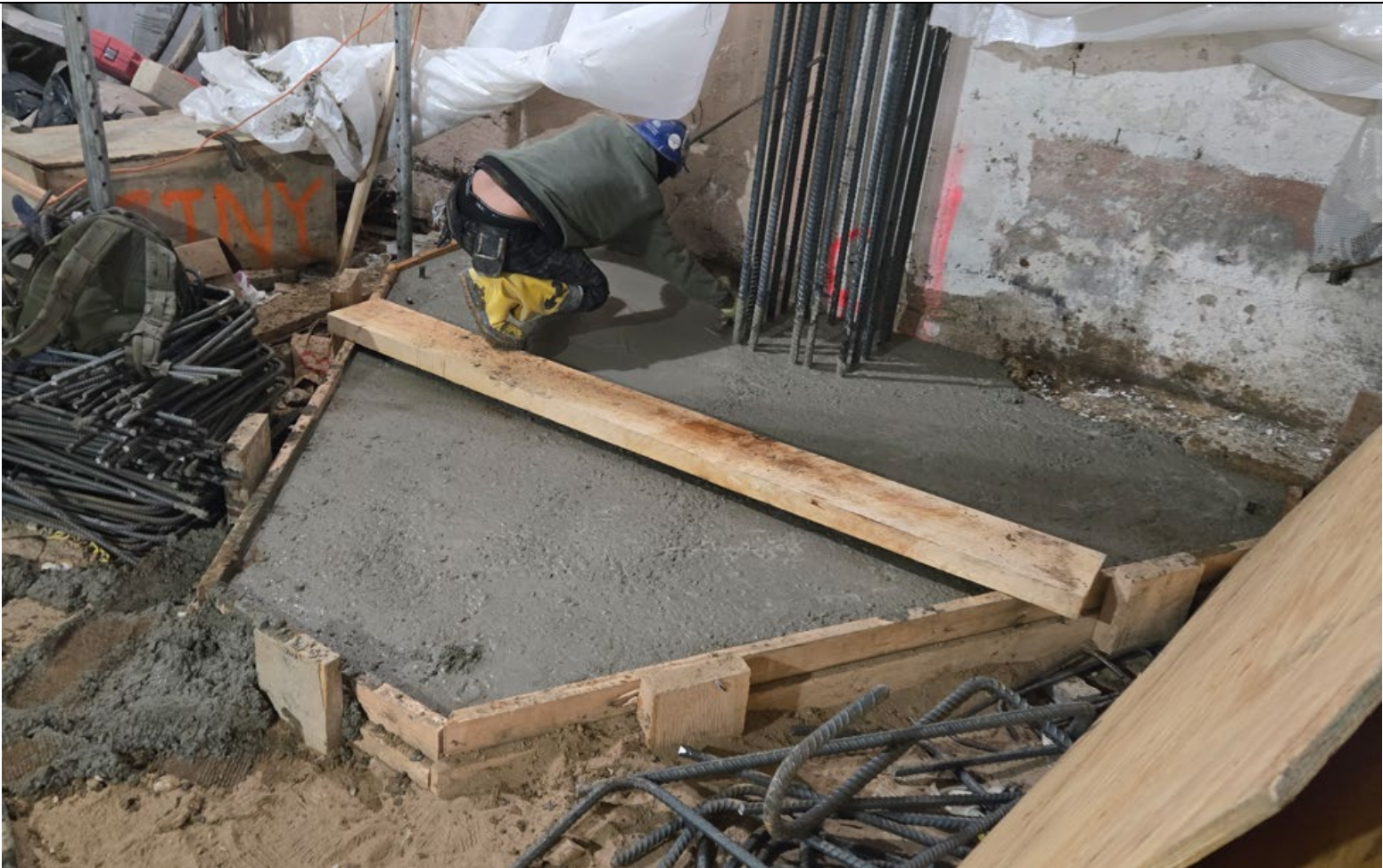
Photo 1: Concrete was poured for PC-4ASW
