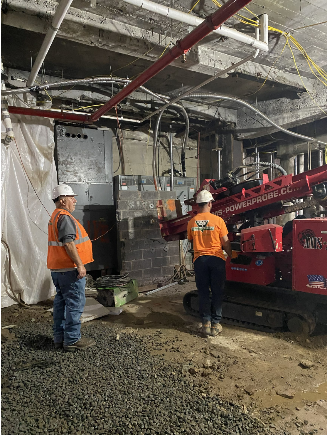
Photo 2: Drill rig positioned over SVE-2
