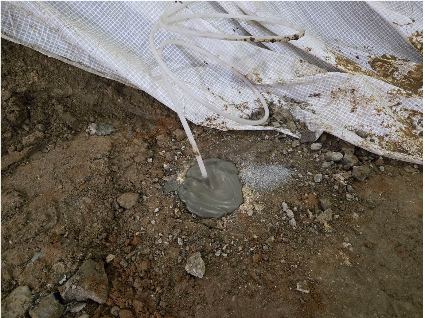
Photo 6: Installed vapor monitoring point (VP-10)
