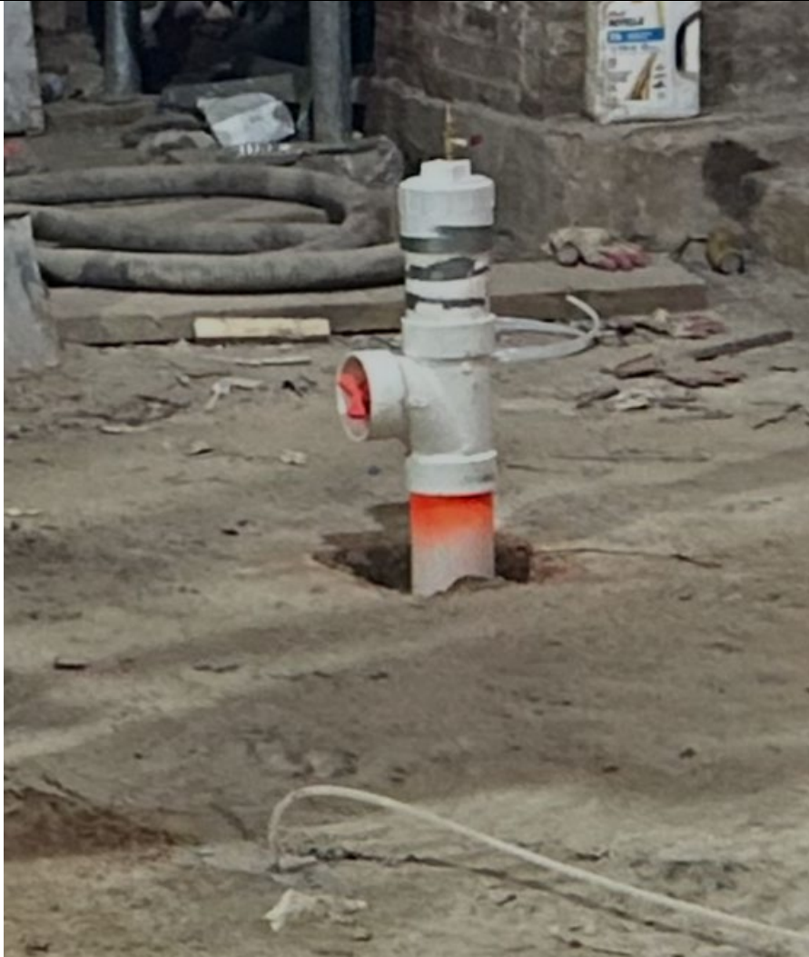
Photo 2: Completed installation of Vapor Probe at 5' NE of SVE-3
