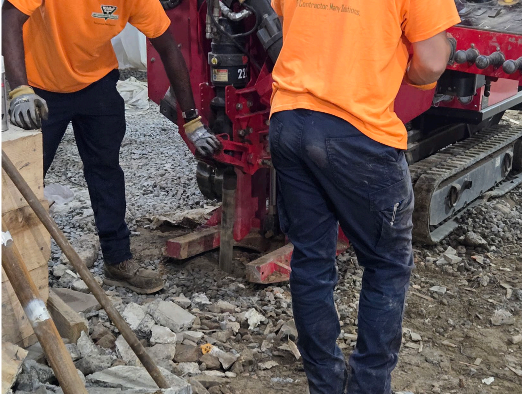
Photo 1: Installation of vapor monitoring points (VP-6)
