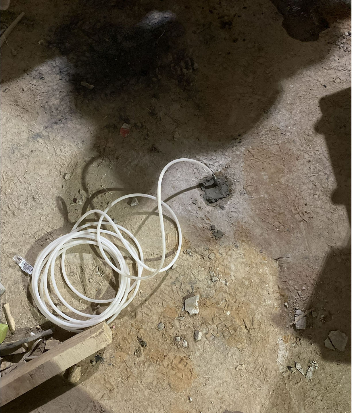
Photo 2: Completed installation of Vapor Probe at 10' east of SVE-3
