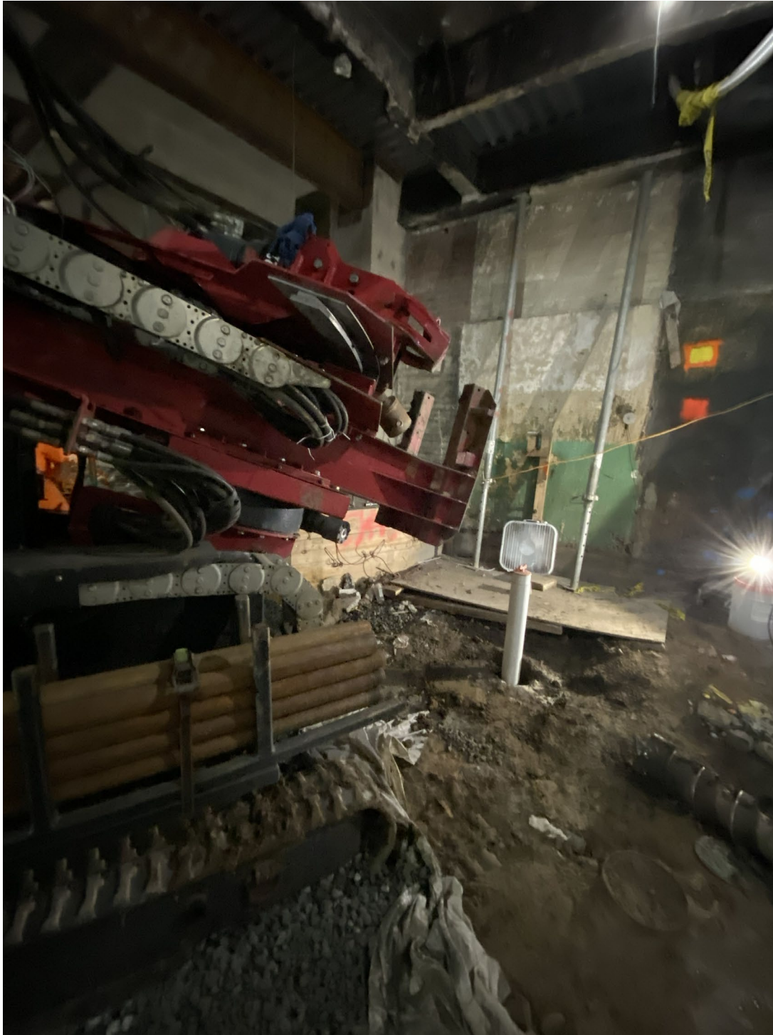
Photo 3: Completed test well SVE-1
