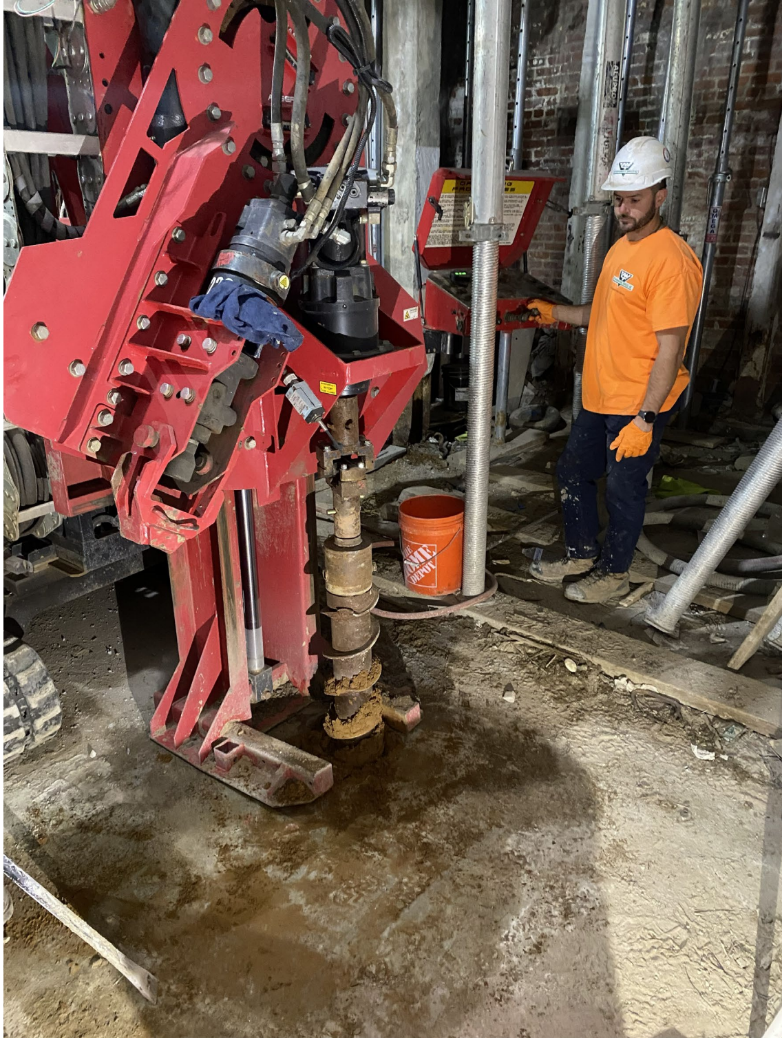
Photo 1: Drilling of test well, SVE-3
