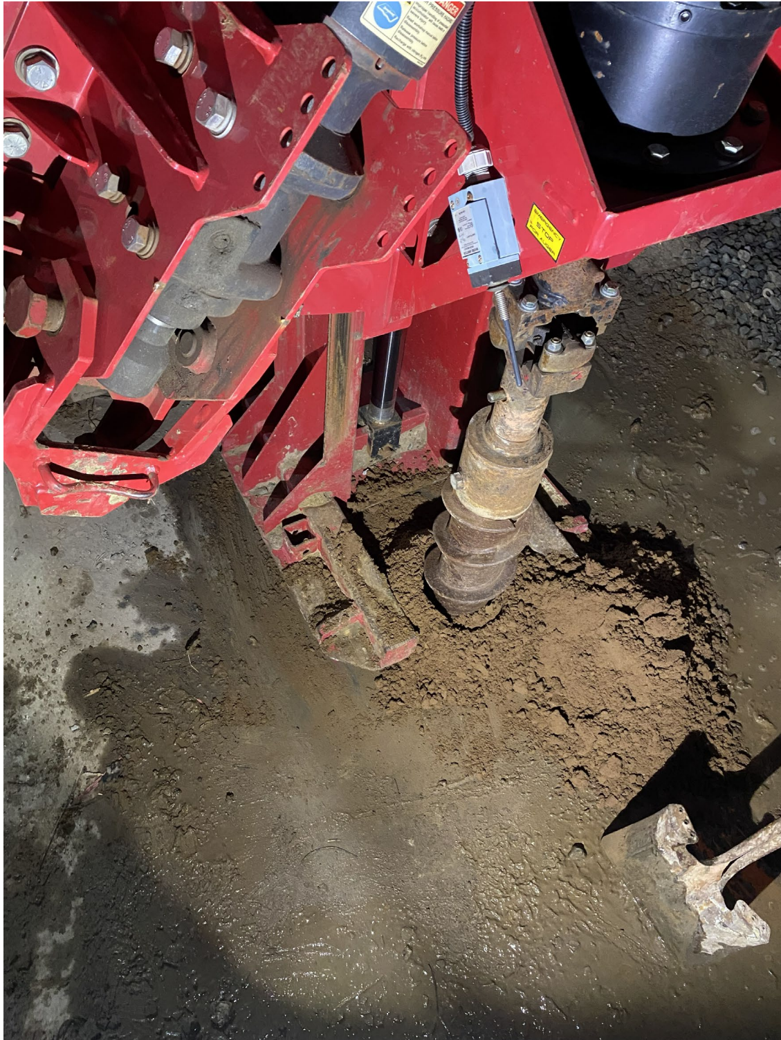
Photo 1: Drilling of test well, SVE-2
