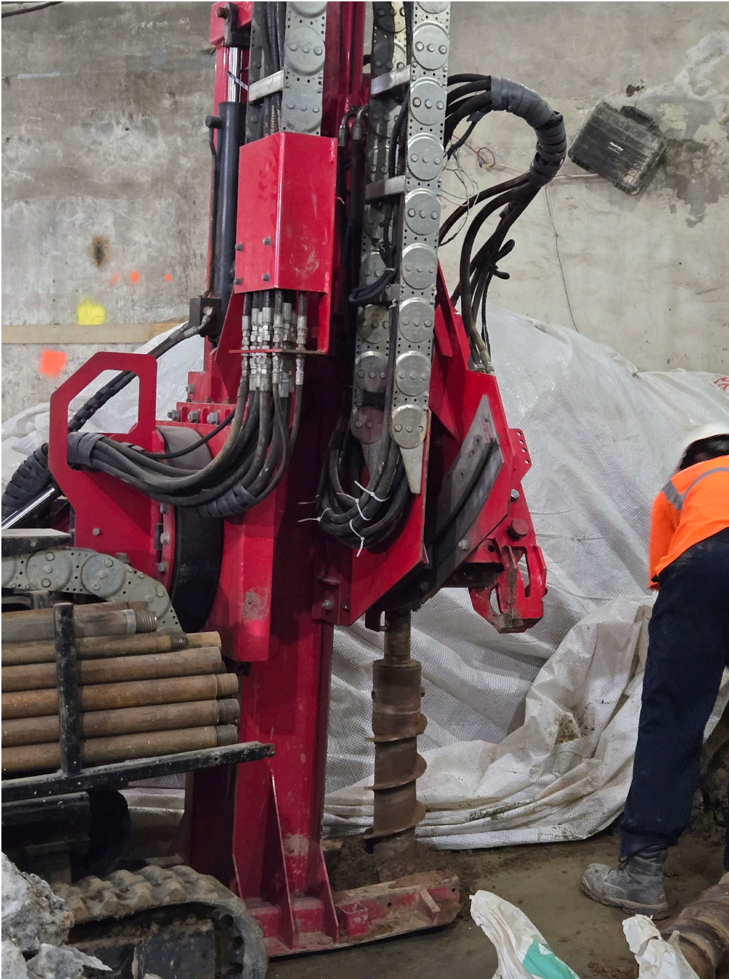
Photo 3: Installation of SVE-8
