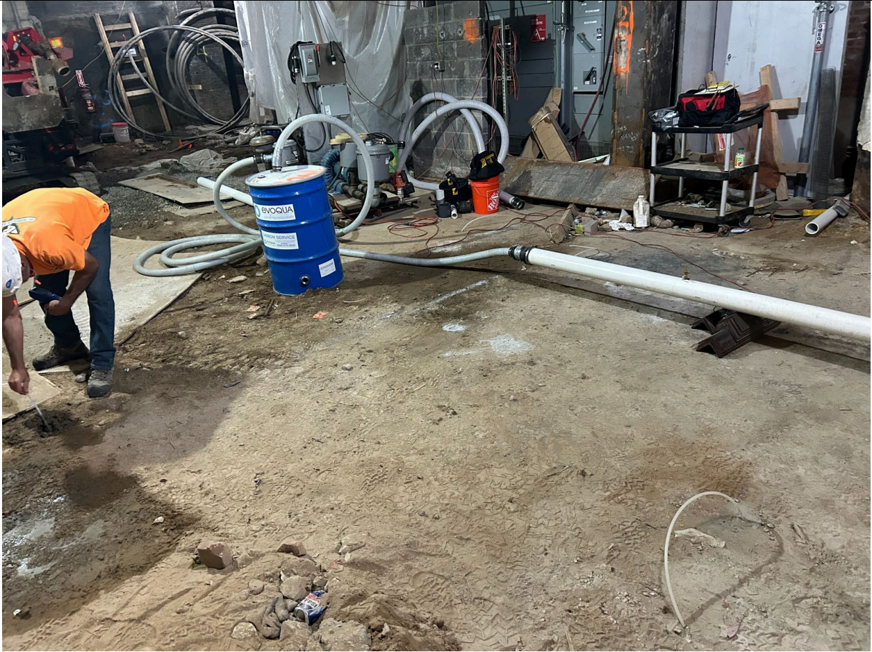
Photo 3: Vapor point installation of point 15' NE of SVE-3
