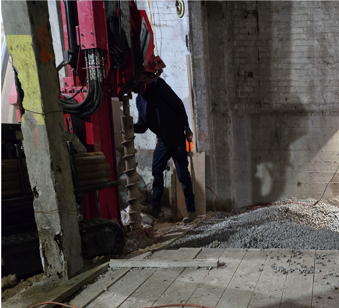
Photo 1: Installation of SVE-4
