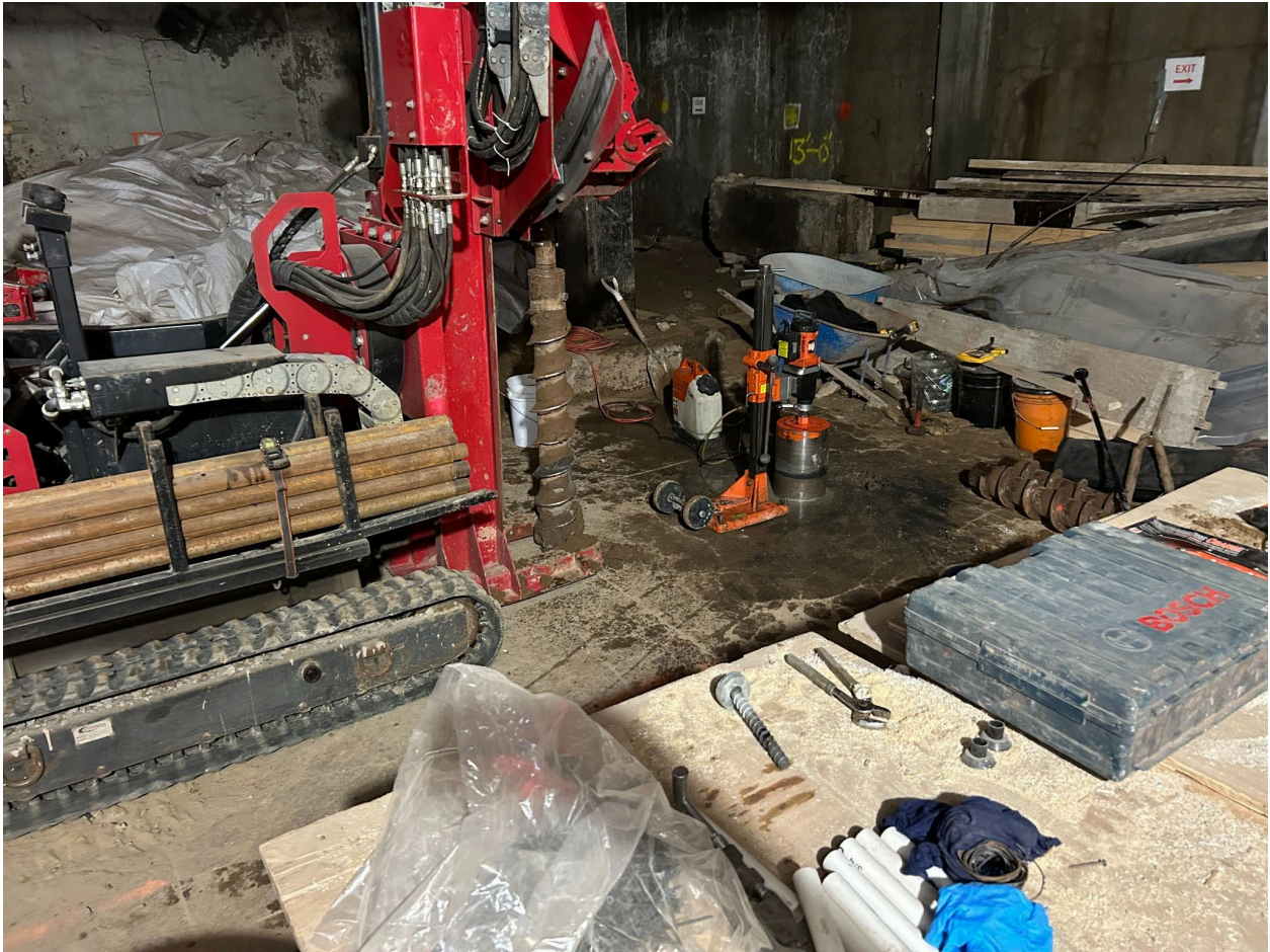
Photo 6: Installation of SVE-12
