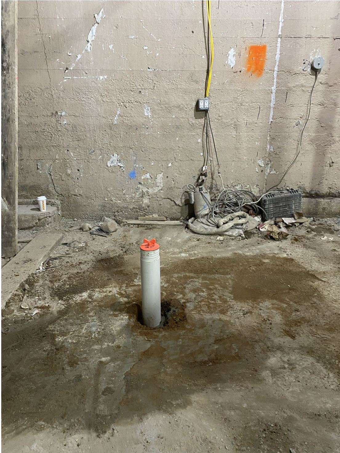
Photo 2: Completed test well, SVE-3
