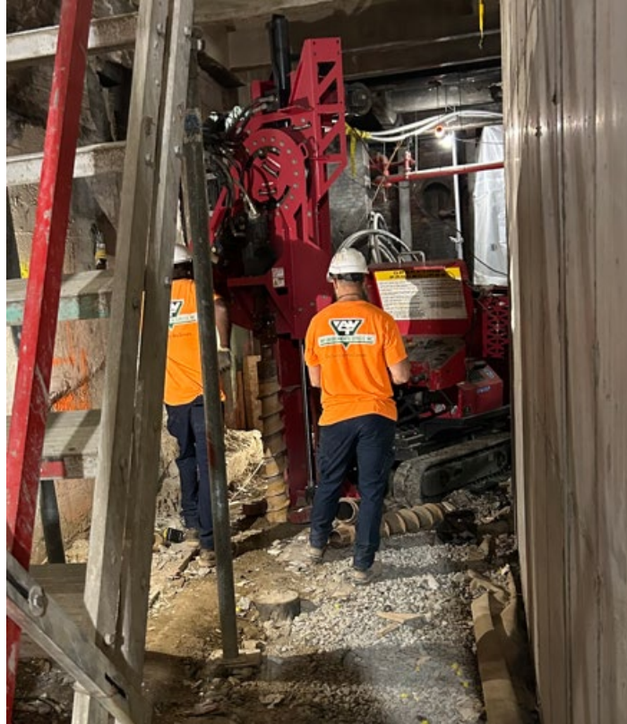
Photo 1: Installation of SVE-5
