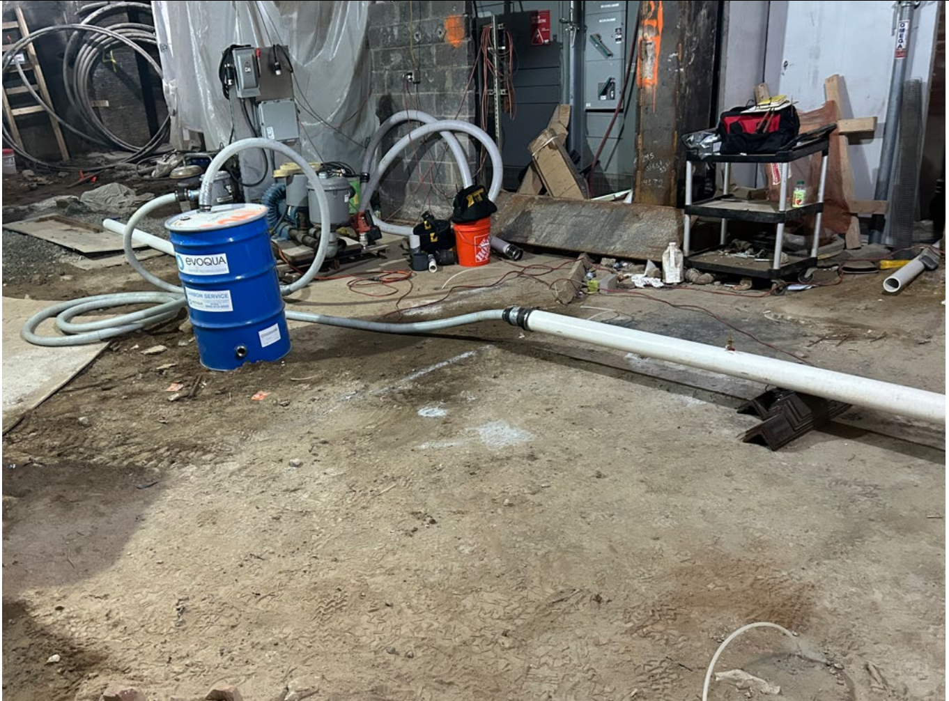
Photo 4: Pilot Testing on SVE-3
