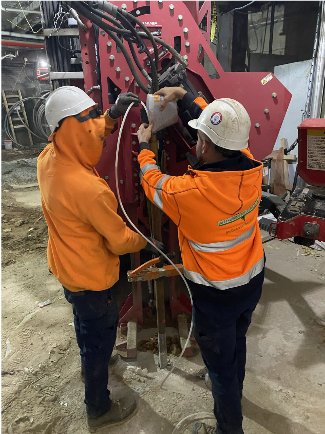
Photo 3: Installation of Vapor Probe at 5' northeast of SVE-3
