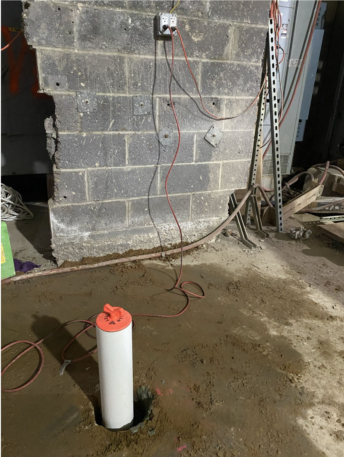
Photo 2: Completed test well, SVE-2
