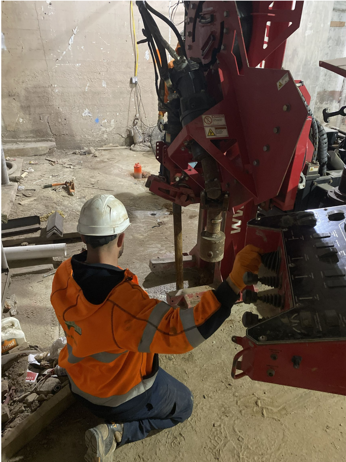
Photo 1: Installation of Vapor Probe at 10' east of SVE-3
