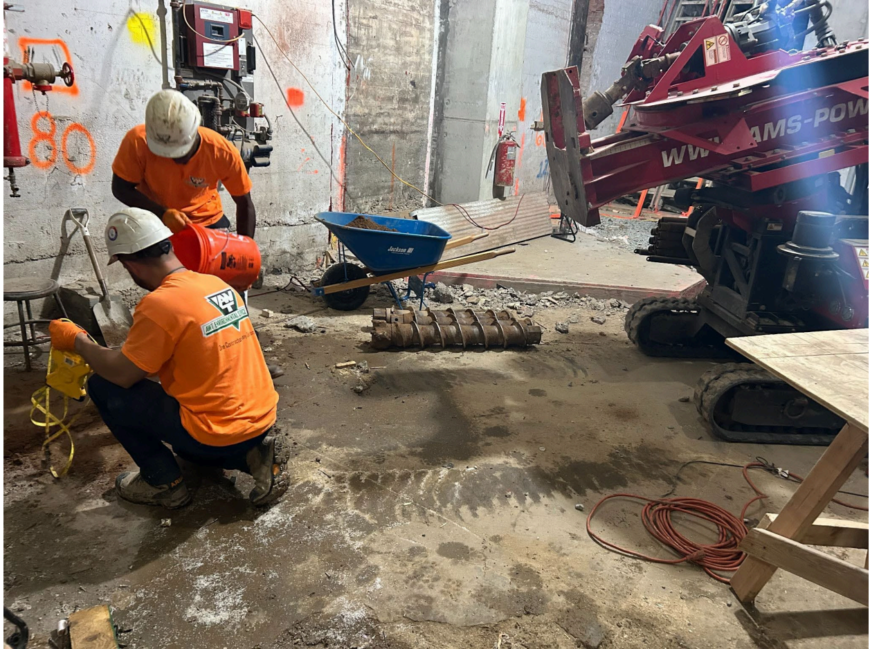
Photo 1: Installation of SVE-9
