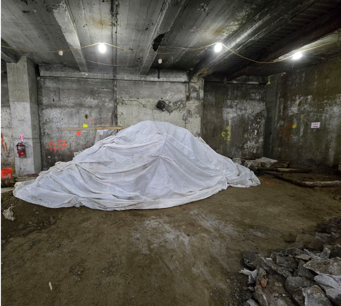
Photo 9: Stockpiled soils covered with plastic sheeting
