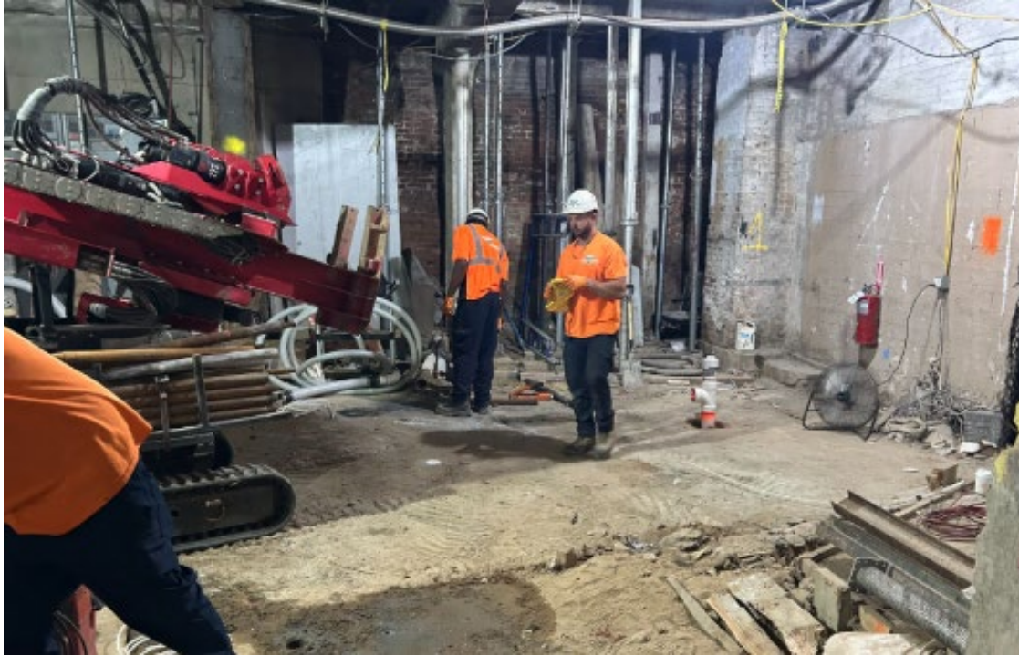
Photo 1: Installation of Vapor Probe at 5' NE of SVE-3
