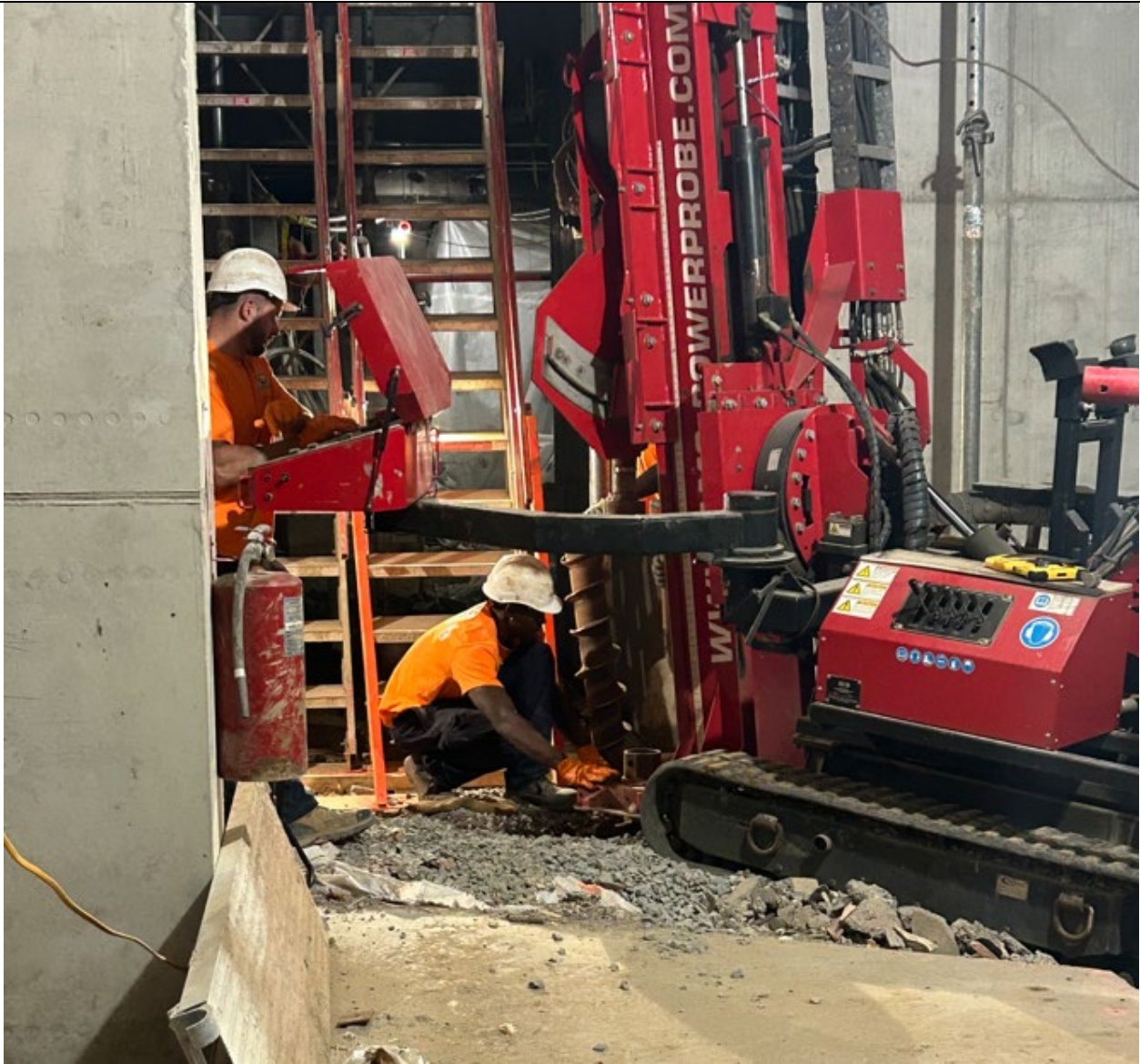
Photo 3: Installation of SVE-7
