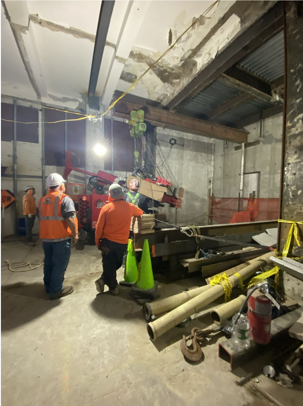
Photo 1: Drill rig lowered into basement with hoist and beam system.
