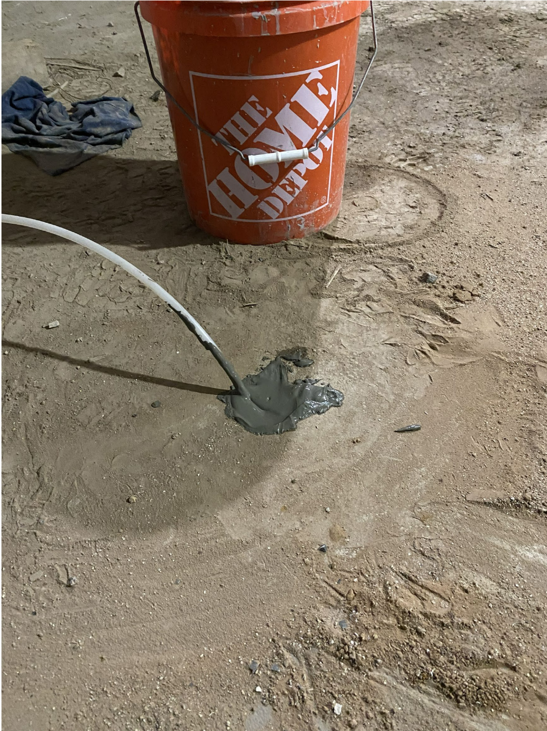
Photo 2: Completed installation of Vapor Probe at 15' east of SVE-3
