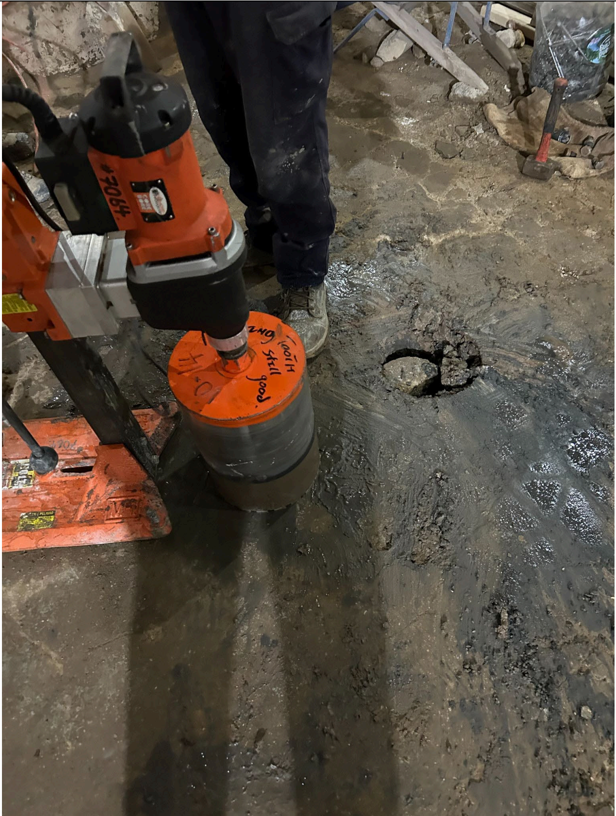
Photo 5: Refusal at initial location for SVE-11, coring at new location
