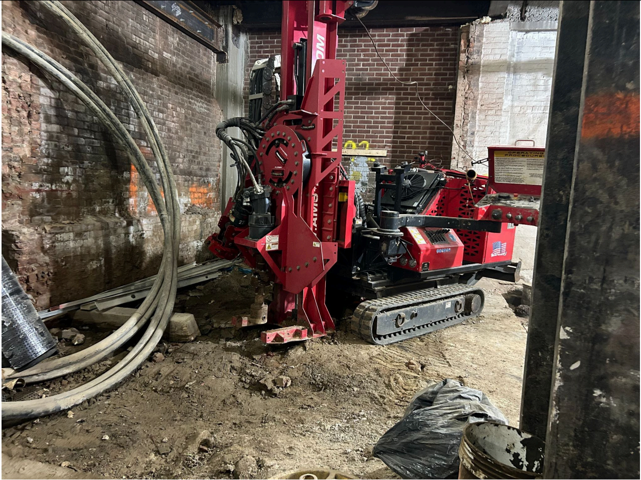
Photo 3: Installation of SVE-12
