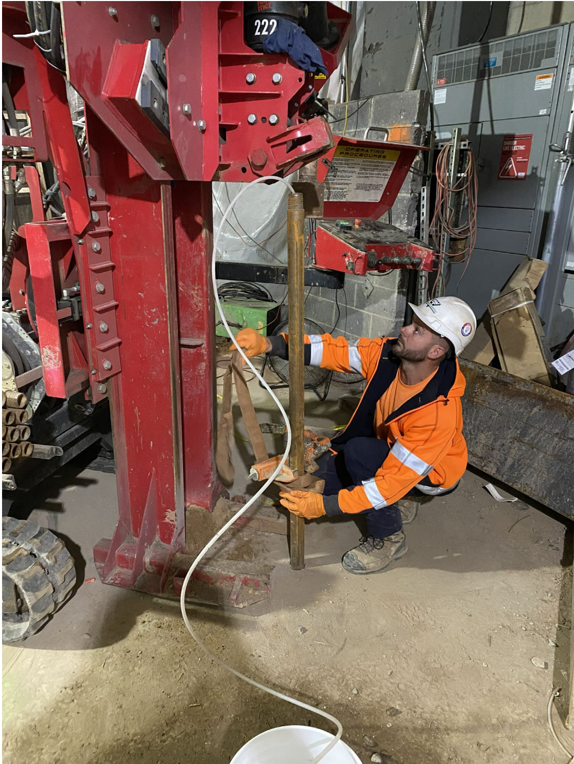
Photo 1: Installation of Vapor Probe at 15' east of SVE-3
