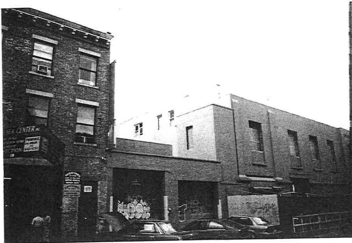
PHOTO 3. View of the east side of the subject building.
