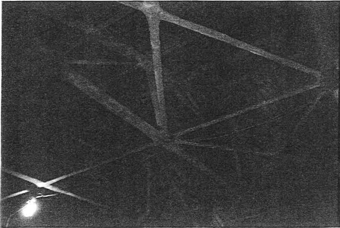
PHOTO 13. View of the ceiling structure of the subject building.
