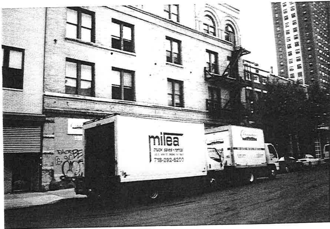
PHOTO 5. View of an adjacent property to the north of the subject property, beyond West 18 th Street.
