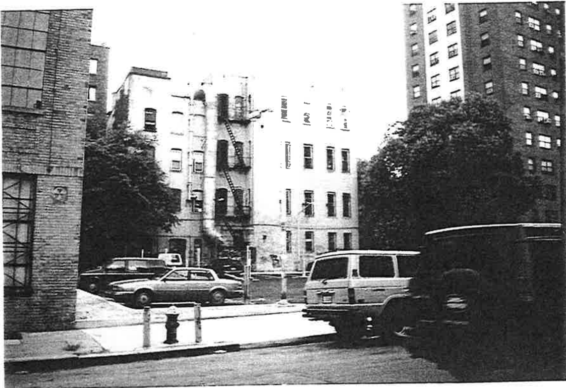
PHOTO 7. View of an adjacent property to the north of the subject property, beyond West 18 th Street.
