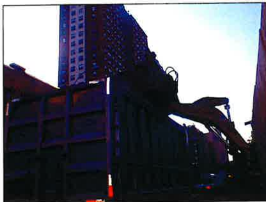
3. Loading of contaminated soil onto trucks for transportation to SRP.
