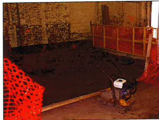
5. Back-filled excavation with clean recycled concrete aggregate to stabilize support column.
