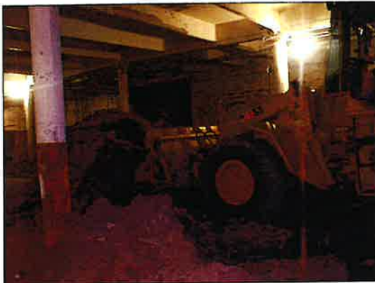
2. Removal of contaminated soil with a front end loader.
