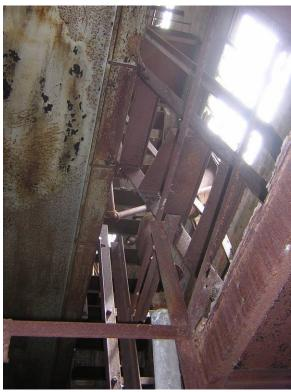
Photo No. 22 – Damaged Interior Metal Stairs at 1<sup>st</sup> Floor of Three-Story Building
