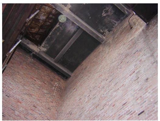
Photo No. 10 – Concrete Roof Beams On Masonry Bearing Walls of Three-Story Building
