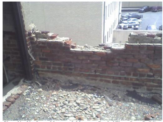
Photo No. 20 – Loose Masonry & Mortar at Roof of Three-Story Building
