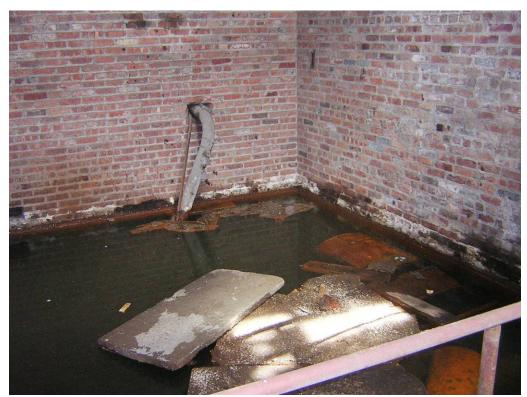
Photo No. 23 – Flooded Basement of Three-Story Building
