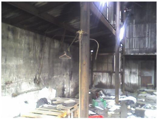
Photo No. 12 – Oil Tank Concrete Containment Wall & Steel Roof Framing of Two-Story Building
