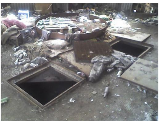
Photo No. 16 – Two Unprotected Floor Openings at 2<sup>nd</sup> Floor of Four-Story Building
