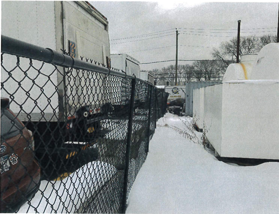
Photo 1. West side of treatment Compound
