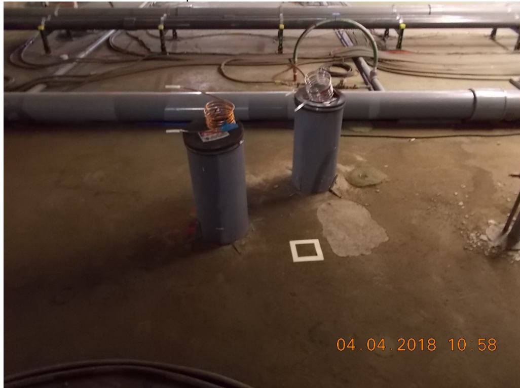
Photo # 22: Surface Sample Location #5 – Concrete Floor in front of MWR-4
