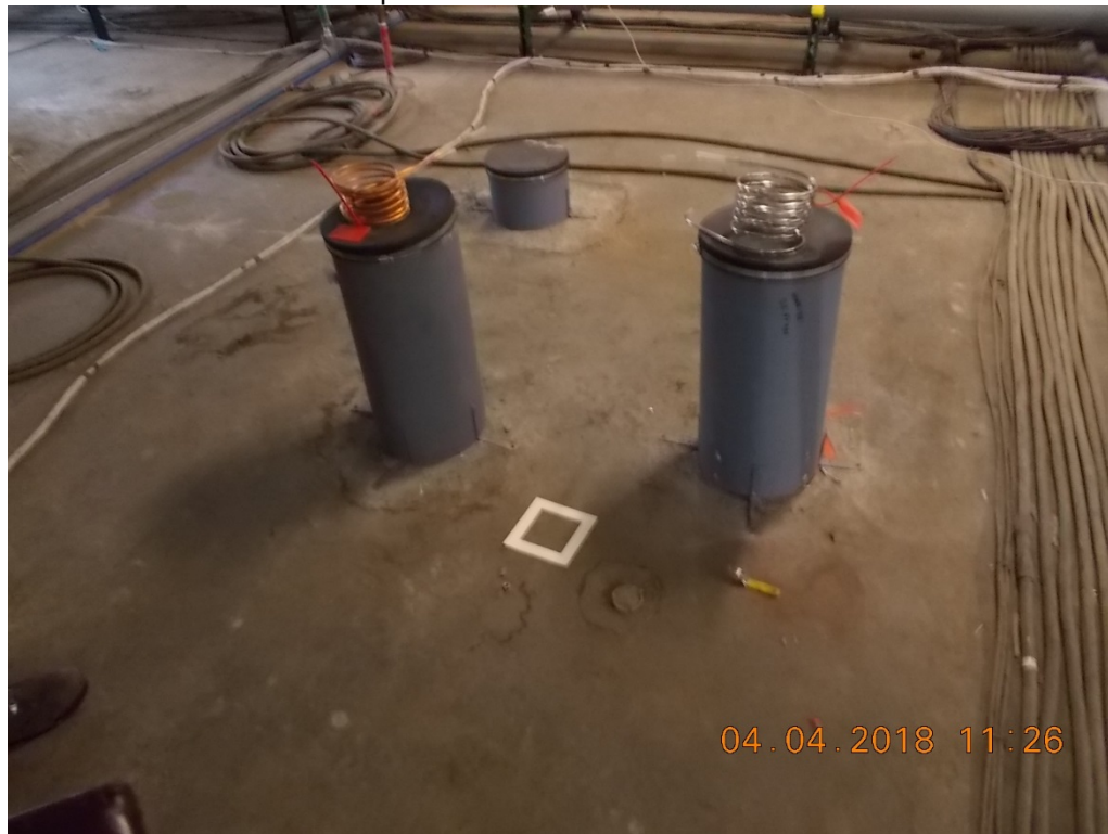
Photo # 27: Surface Sample Location #10 – Concrete Floor in front of MWR-3S
