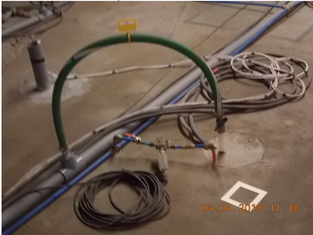
Photo # 25: Surface Sample Location #8 – Concrete Floor in front of G03
