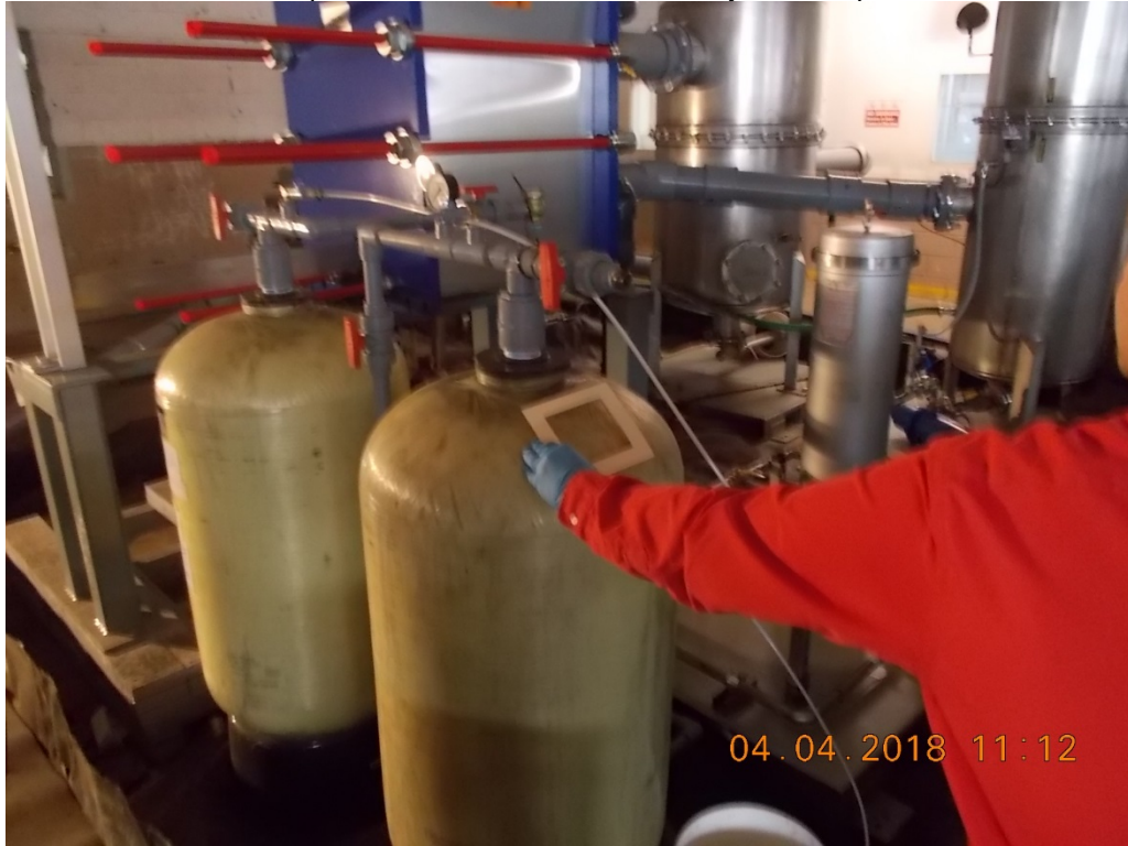
Photo # 24: Surface Sample Location #7 - Remediation System, Top of Carbon Cannisters
