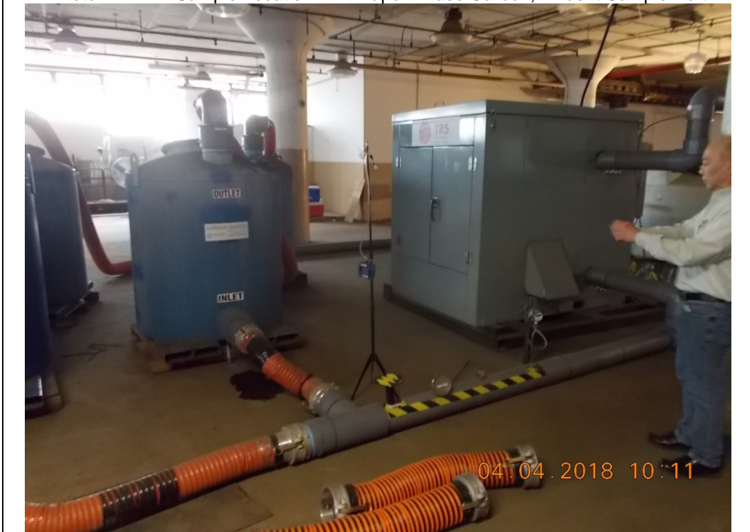
Photo # 14: Air Sample Location #2 – Vapor Phase Carbon, Influent Sample Port
