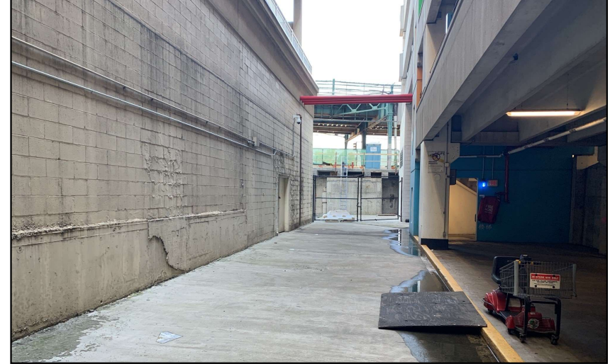
Photograph 6: The concrete slab between the retail space and the parking garage on the western portion of the Property (Parcel 2).
