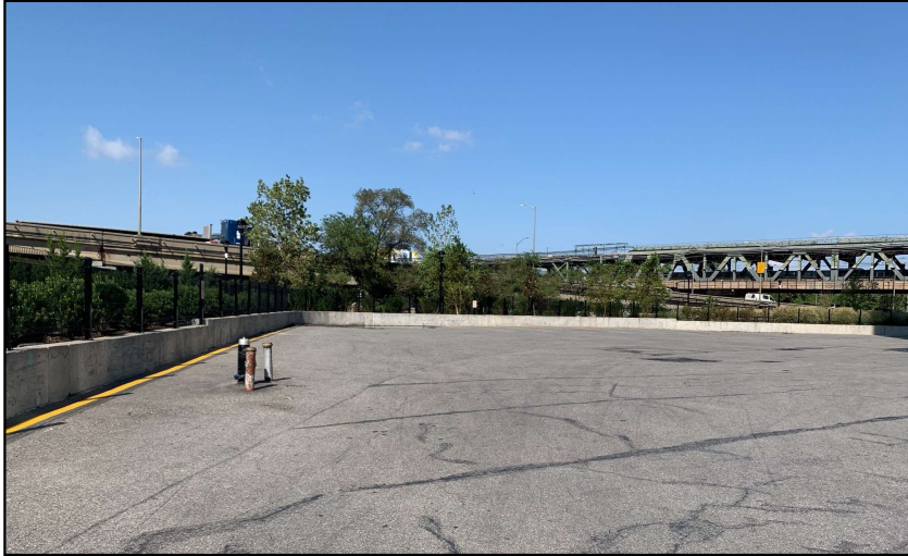
Photograph 1: The asphalt paved loading dock area on the southwestern portion of the Property (Parcels 2 and 3).
