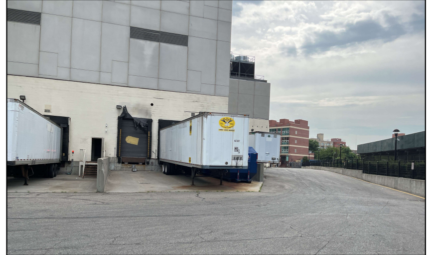
Photograph 6: The asphalt-paved loading dock area on the western portion of the Property (Parcel 2).
