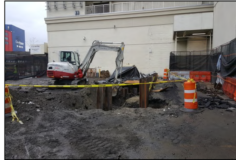
Photograph 6: Soil excavation to expose H-piles at the SVP West Entrance Pavilion.
