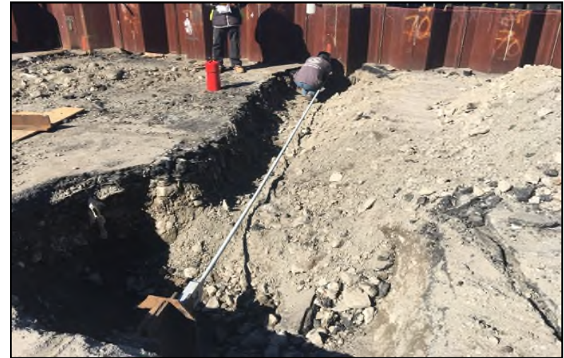
Photograph 18: Tie-back installation in RMZ A soil at the Parcel 3 marine bulkhead sheeting.
