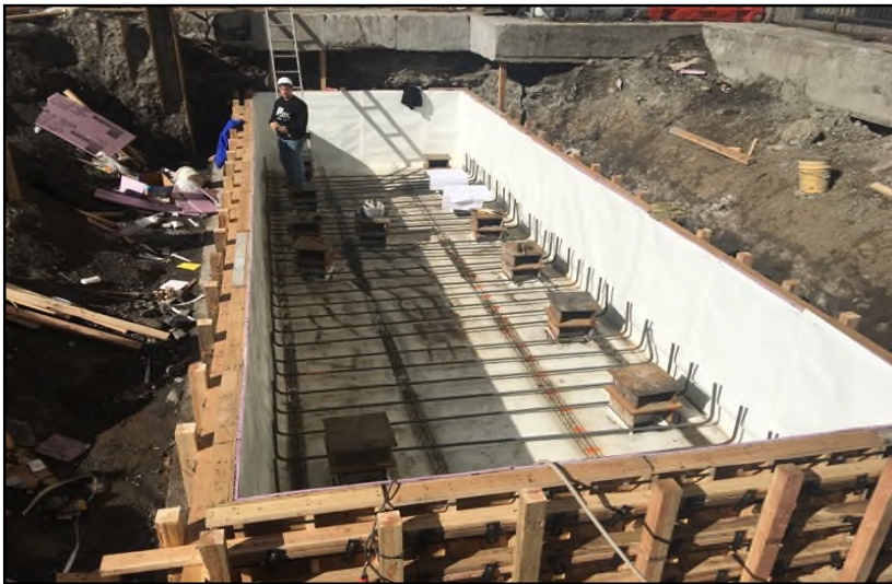
Photograph 11: View of the vapor barrier installed on exterior portions of the elevator pit.
