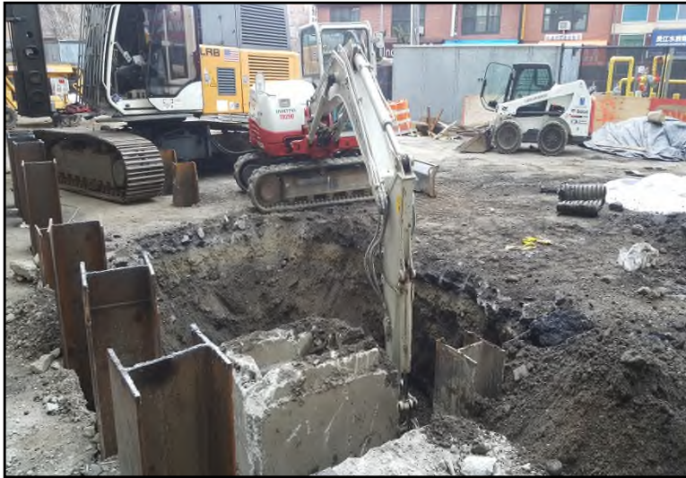
Photograph 5: RMZ A soil excavation to expose a catch basin at the SVP West Entrance Pavilion.
