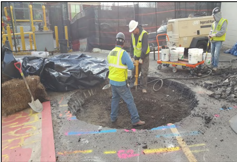
Photograph 3: RMZ A soil excavation to expose utilities at the SVP West Entrance Pavilion (Parcels 1 and 2).
