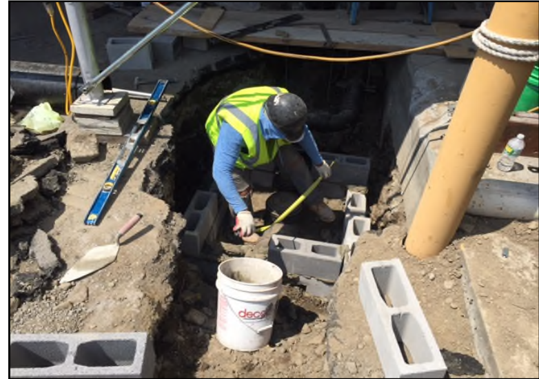
Photograph 2: Utility installation on the southern portion of Parcel 2.
