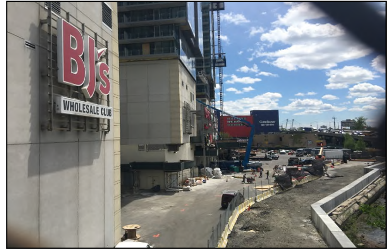
Photograph 2: The western portion of the Property (Parcels 2 and 3).
