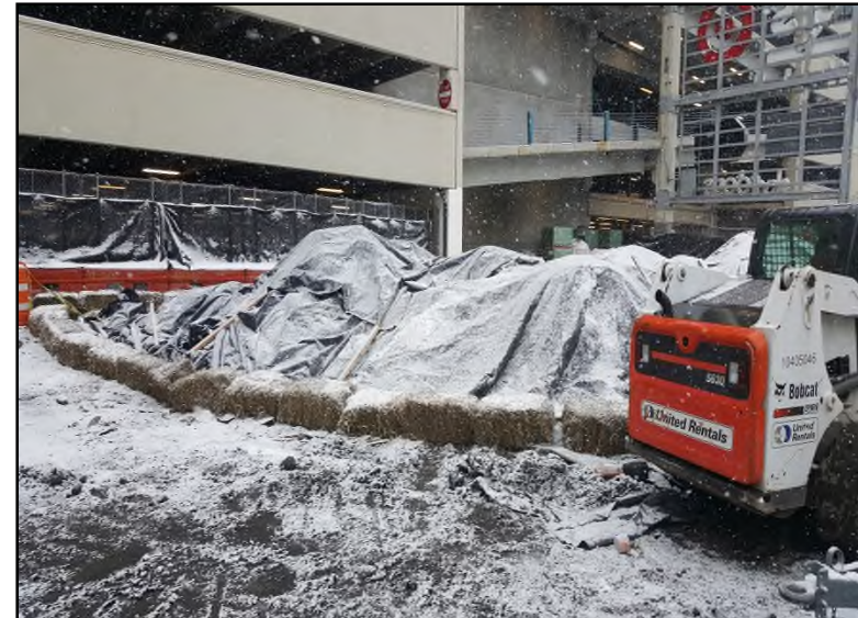
Photograph 8: RMZ A and RMZ B soil stockpiles and sediment control (hay bales) at the SVP West Entrance Pavilion.
