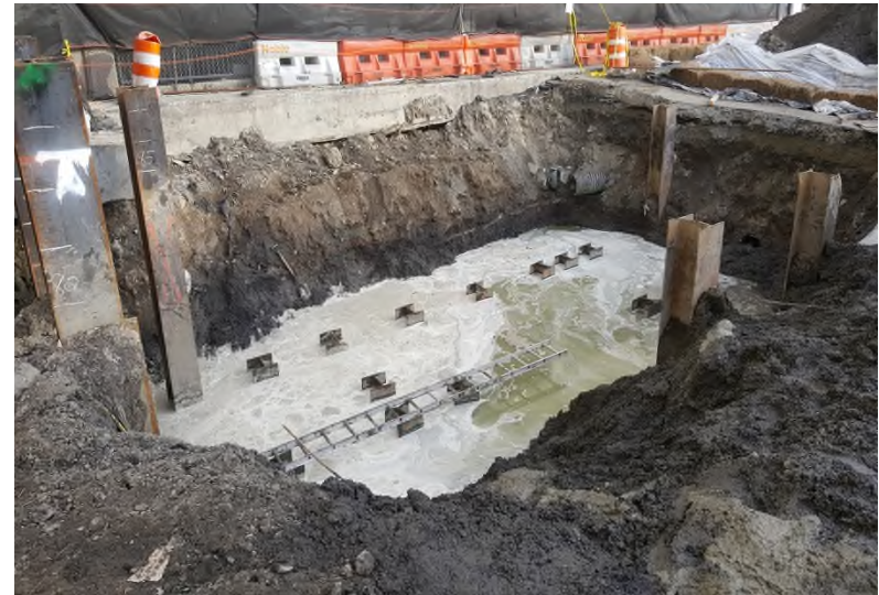
Photograph 10: View of the SVP West Entrance Pavilion elevator pit concrete mud slab (post-pour).
