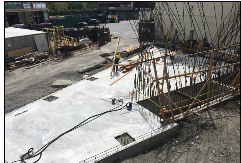
Photograph 16: Southwestern view of the SVP West Entrance Pavilion.
