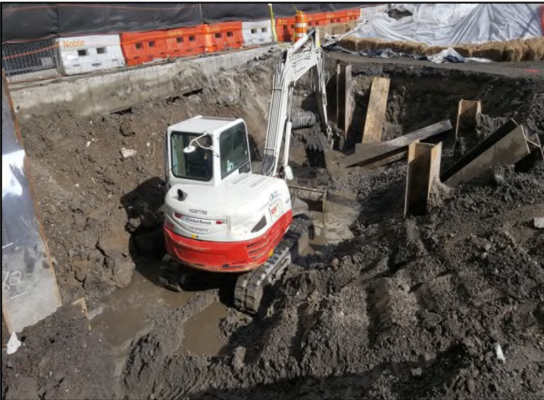
Photograph 7: RMZ B soil excavation for the SVP West Entrance Pavilion elevator pit.
