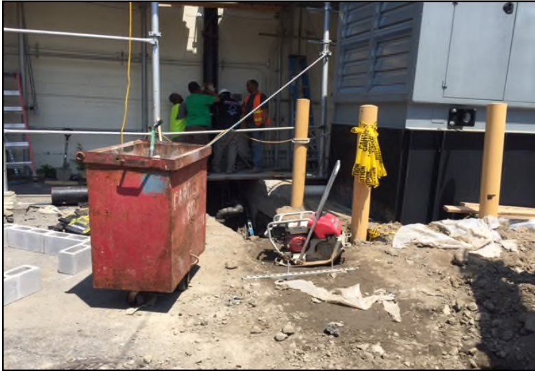
Photograph 1: Utility trench excavation on the southern portion of Parcel 2.
