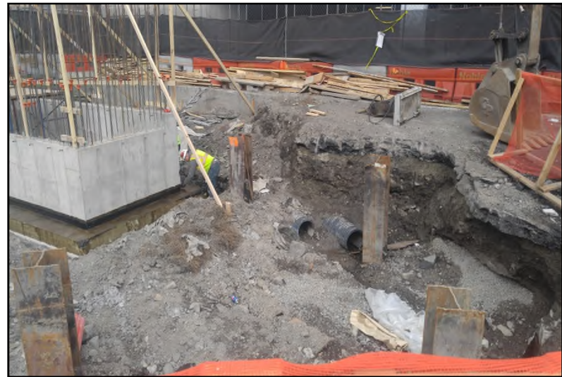
Photograph 12: Applying Aquafin® brand waterproofing on the elevator pit foundation.
