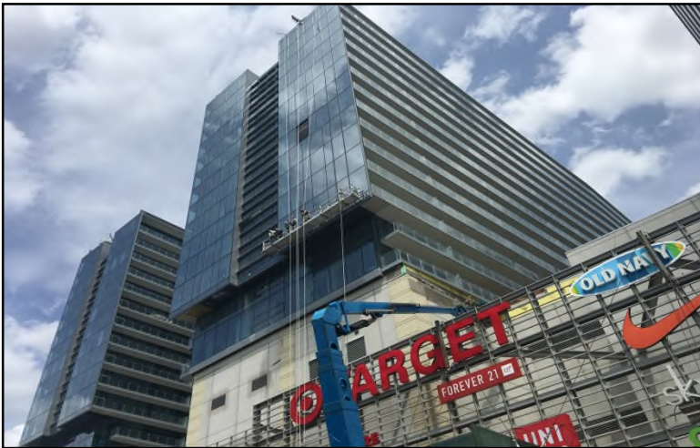
Photograph 7: The residential Towers atop the western retail podium (Parcel 2).
