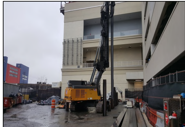
Photograph 4: Driving H-piles at the SVP West Entrance Pavilion.
