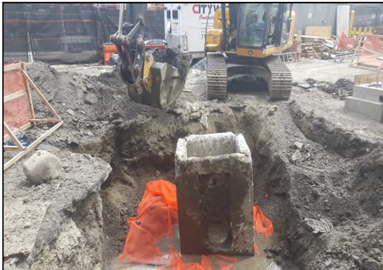
Photograph 15: Catch basin installation and orange snow fencing as a demarcation layer east-adjacent to the SVP West Entrance Pavilion.
