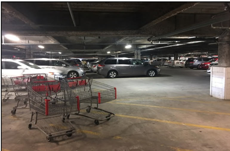
Photograph 11: Concrete slab as part of the site cover in the ground floor parking garage between the western and eastern retail buildings (Parcels 1 and 2).
