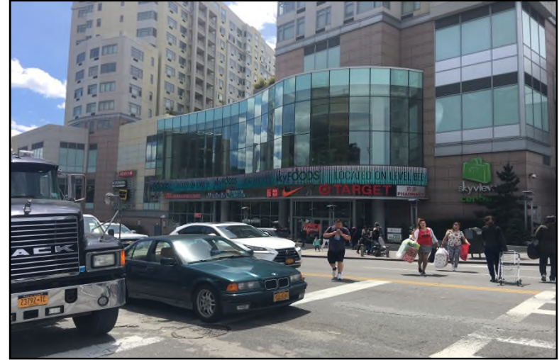
Photograph 6: The retail space and residential towers on the northeastern portion of the Property (Parcel 1).
