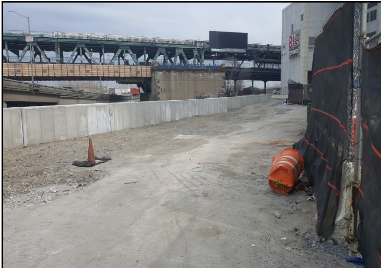
Photograph 19: Northern view of the Parcel 3 esplanade western retaining wall (post-concrete pour).
