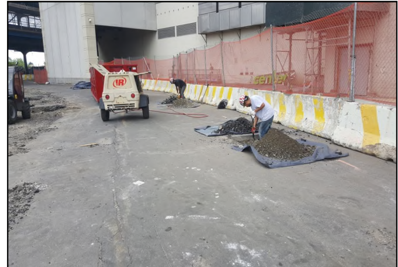
Photograph 20: RMZ A soil excavation for installation of the eastern retaining wall at the Parcel 3 esplanade.
