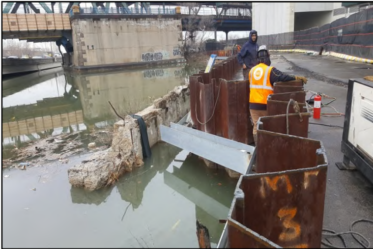
Photograph 17: Northern view of whalers (H-beams) being installed on the Parcel 3 marine bulkhead sheeting.
