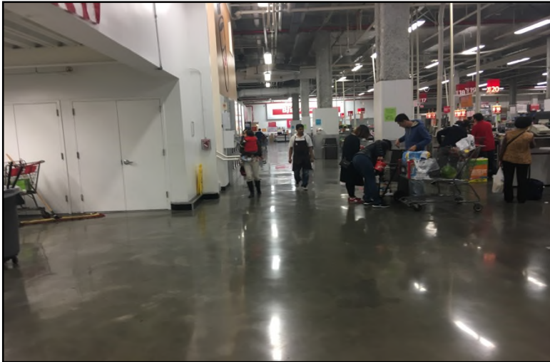
Photograph 9: Concrete slab as part of the site cover in the western retail building (Parcel 2).
