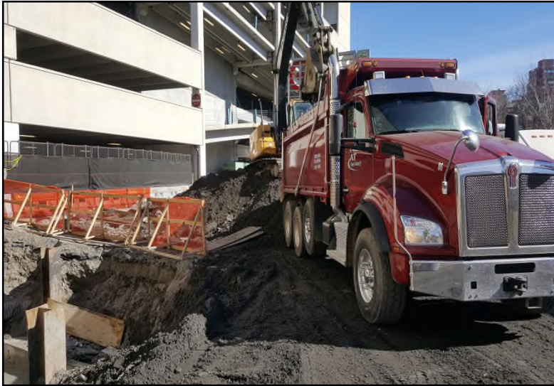
Photograph 9: Loading non-hazardous RMZ B soil into trucks for off-site disposal at Clean Earth of Carteret.
