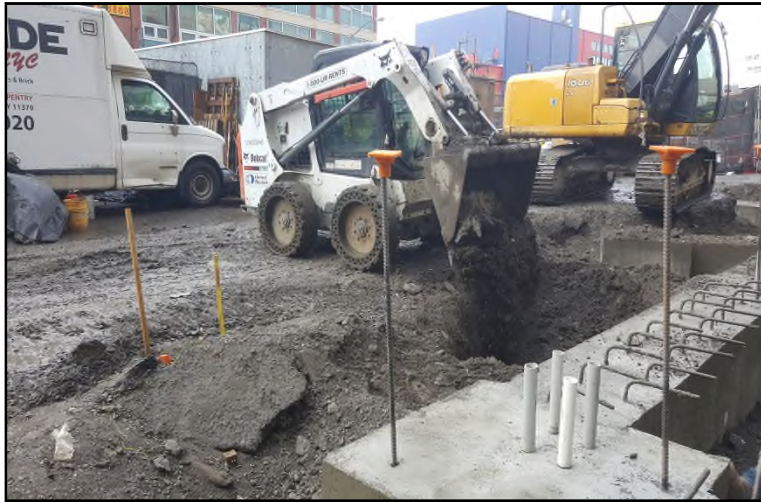
Photograph 13: Backfilling with RMZ A soil around the elevator pit foundation.
