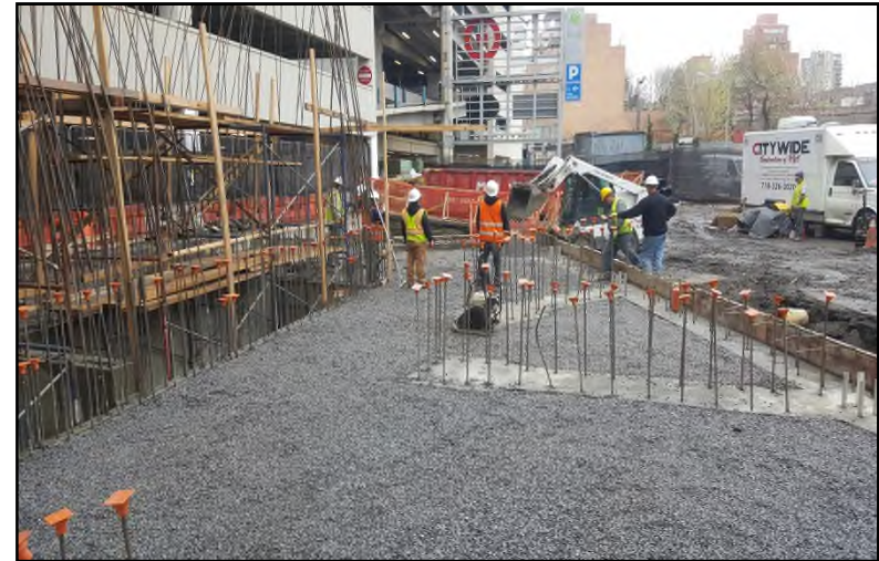
Photograph 14: Backfilling and compacting imported gravel within the elevator building foundation.
