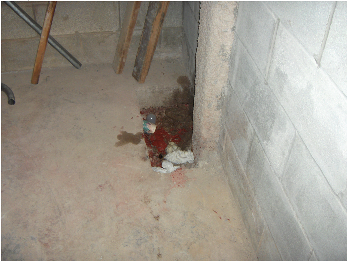
Photo 4, unfinished slab in close proximity to Suction Point 6-1
