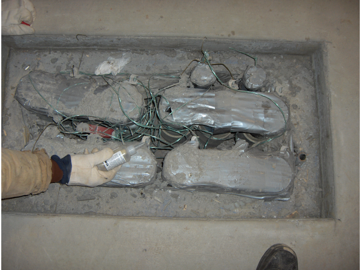
Photo 3, Smoke test of electrical conduits
