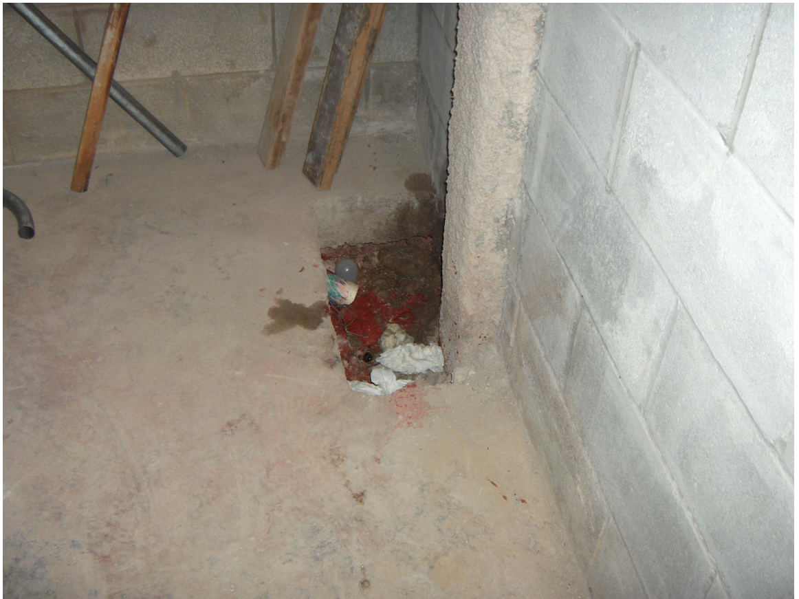
Photo 1, unfinished slab in close proximity to Suction Point 6-1
