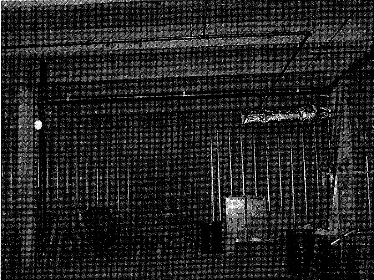
Photo 5: Overhead SSDS piping from suction pit 3-2 south east of building 3 with a T-connection. T connects to riser to the second floor and suction pit 3-1
