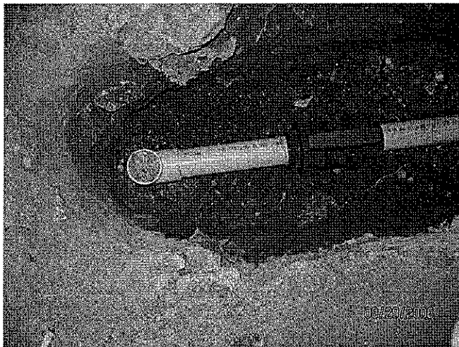
Photo 2: VEW-1 riser connected w\TEE to Sch80 2" PVC pipe connecting to a ball valve;
