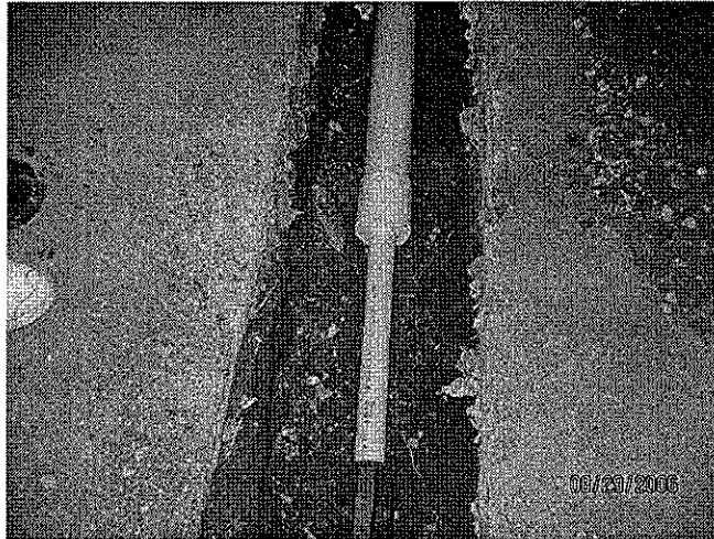
Photo 3: VEW-1 riser connected w/TEE to Sch40 2" PVC pipe connecting to a ball valve; connecting to a 4" Sch 40 pipe using 4" to 2" pipe reducer joint.
