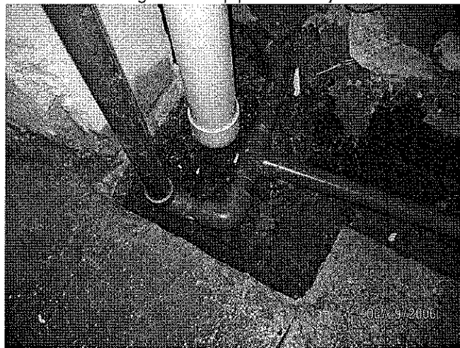
Photo5: AS-1 Sch 80 2" pipe connected AS-2 piping.
