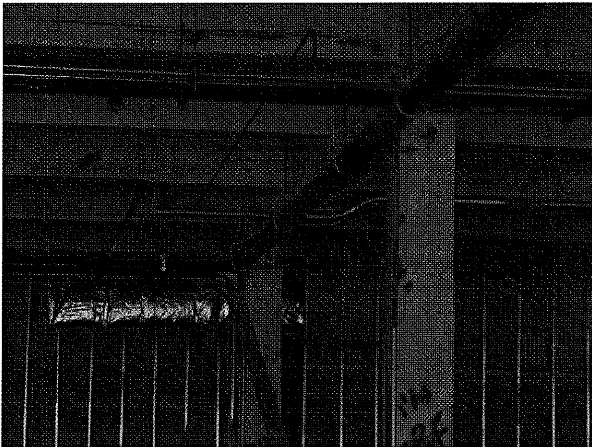
Photo 4: Overhead SSDS piping from suction pit 3-2 south east of building 3
