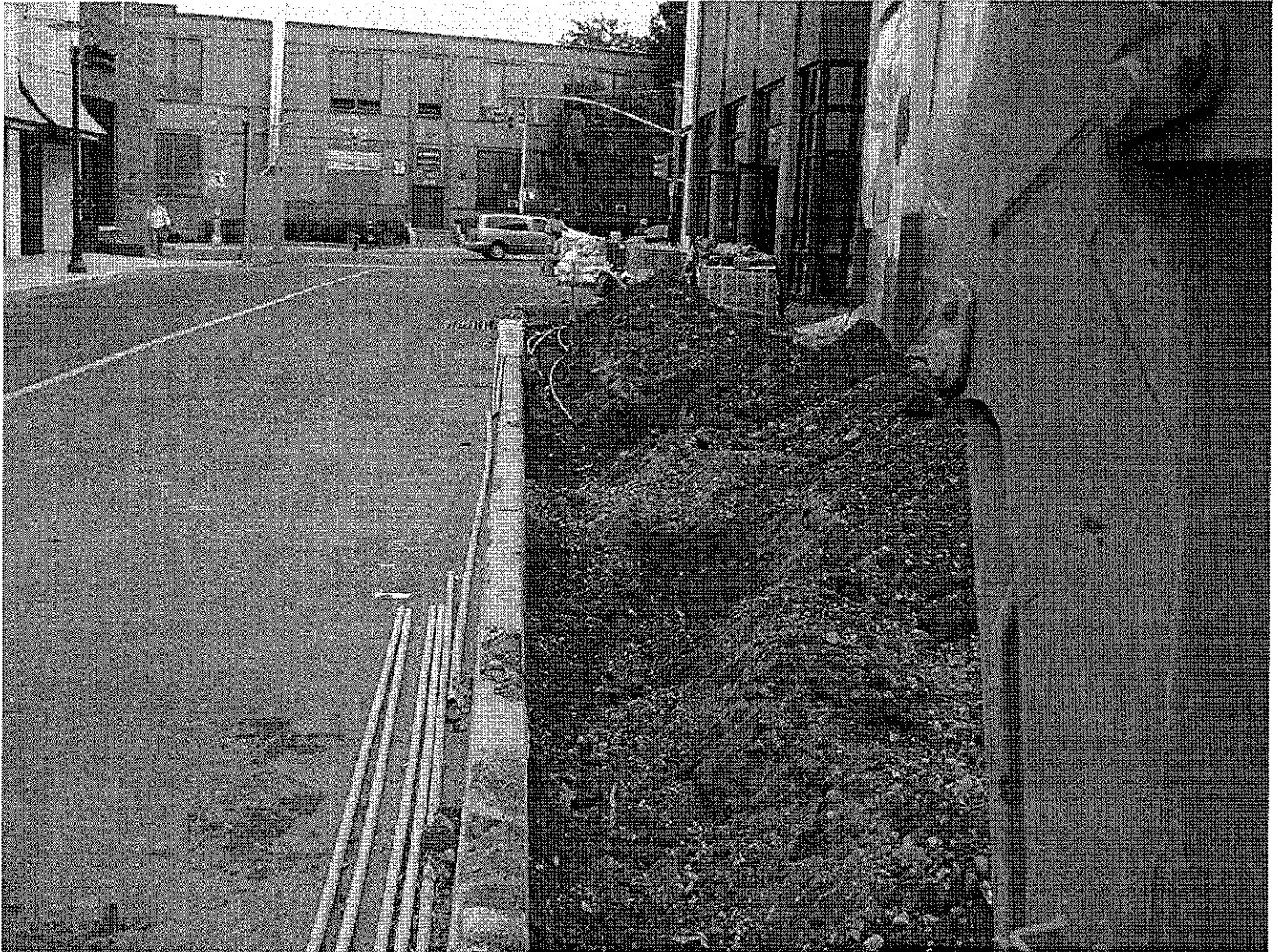
Photo 1: Electric piping for Light Poles South of building 3 sidewalk.
