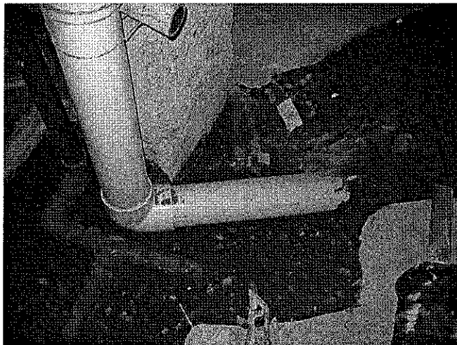
Photo6: Sch 40 4" pipe connection from VEW-1
