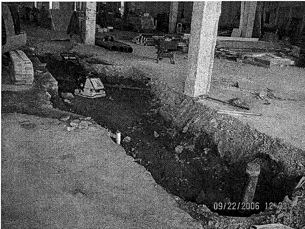
Photo 1: Trench at sanitary sewer partially backfilled (Building 3).
