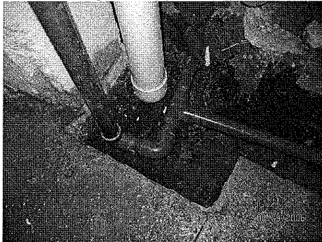
Photo 4: AS-1 Sch 80 2" pipe connected with 2 45° elbows; connected to a TEE to attach AS-2 and AS-1 piping. The TEE than connects to 2 90° elbows to connect to a riser. 4"Sch 40 (white pipe) connected with a 90° elbow to riser up the column.
