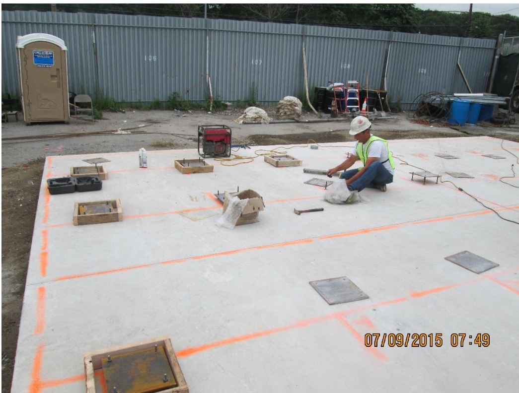
Layout and installation of LNAPL tank bearing plates
