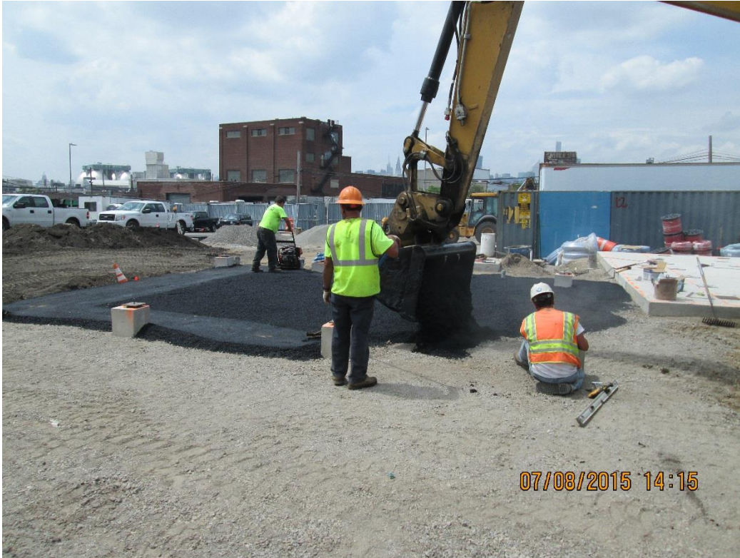
Base paving course under equipment trailers
