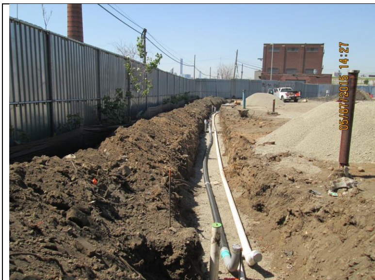
Installation of SVE pipe and HPDE sleeves in TF-5 trench
