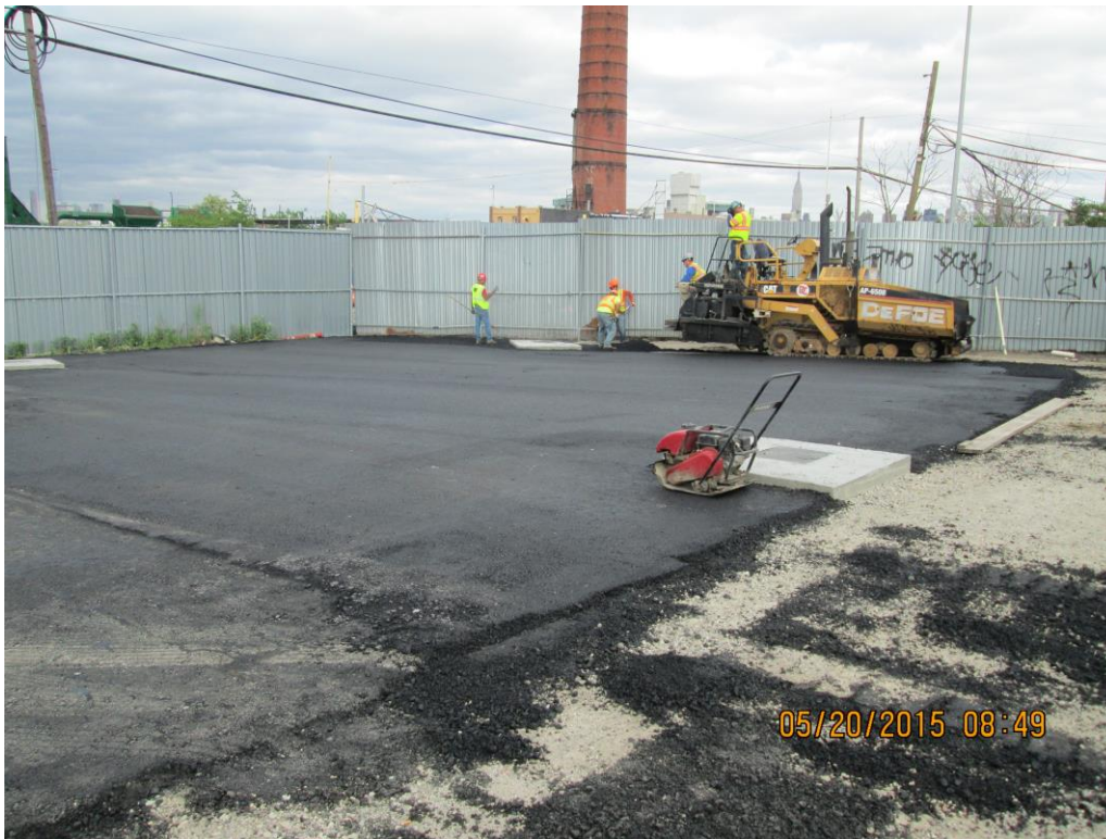
Base Paving RAD II Work Area I
