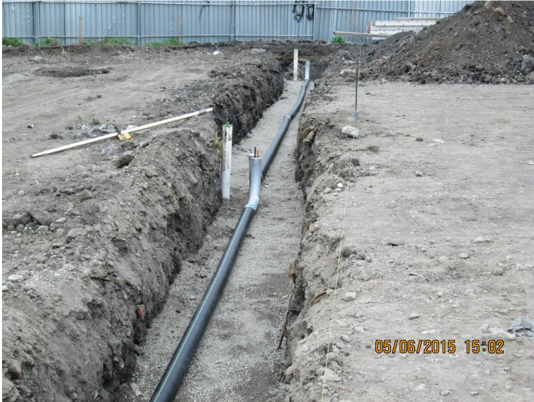
Installation of HPDE sleeves in TF-4 trench
