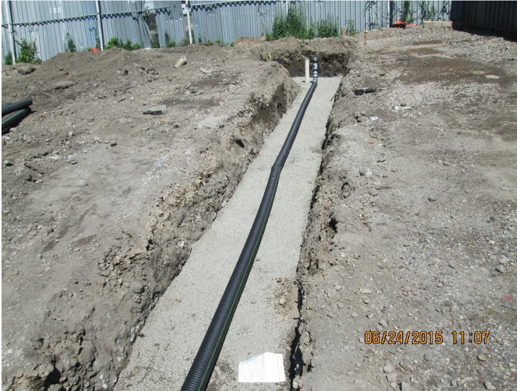
Install HDPE pipe sleeve from S-1D to S-1C
