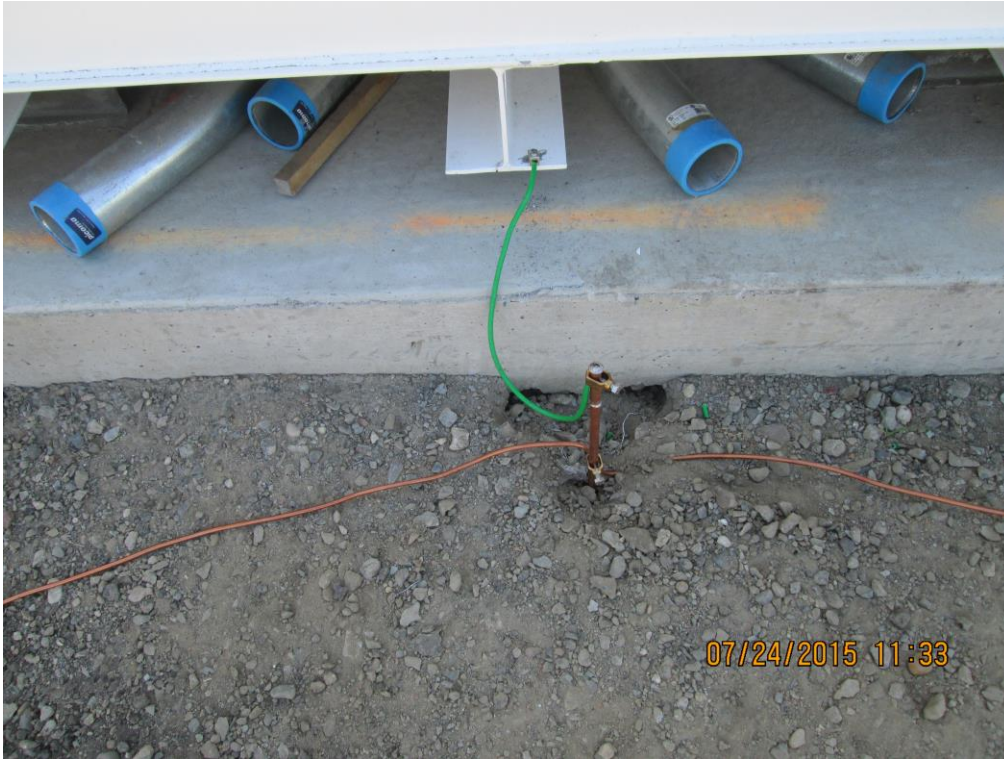
Grounding at LNAPL tanks
