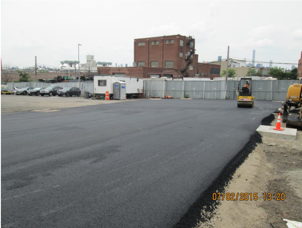
Top course of pavement between Tf-1 line and S-1 line
