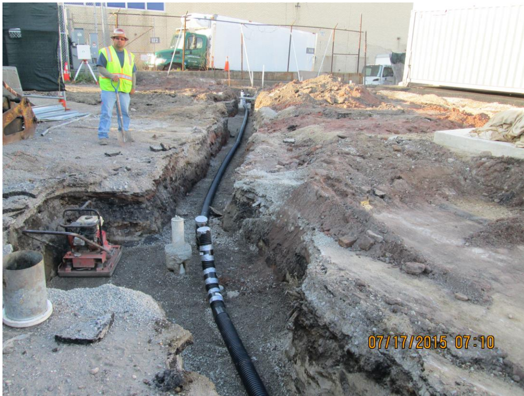
HPDE sleeves in trench segments 48 and 50
