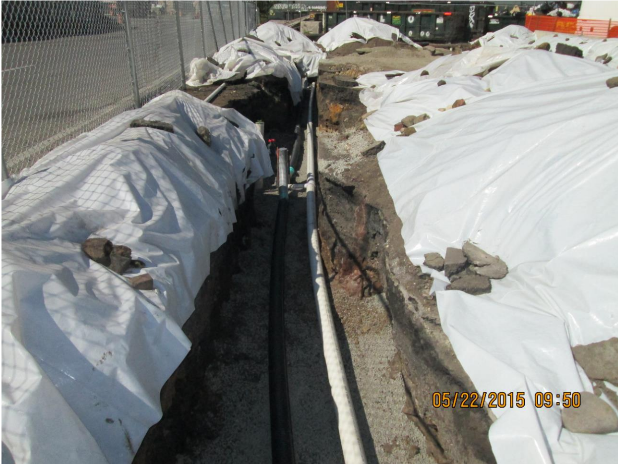
Install VER Piping and HPDE Piping Sleeve in TF-6 Trench
