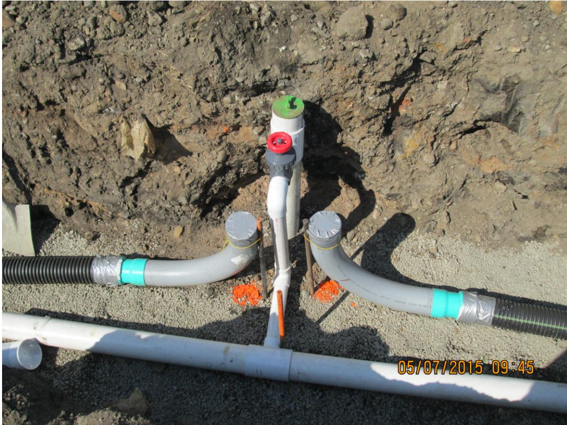
TF-5C Well Head Piping- Typical VER Well Head detail
