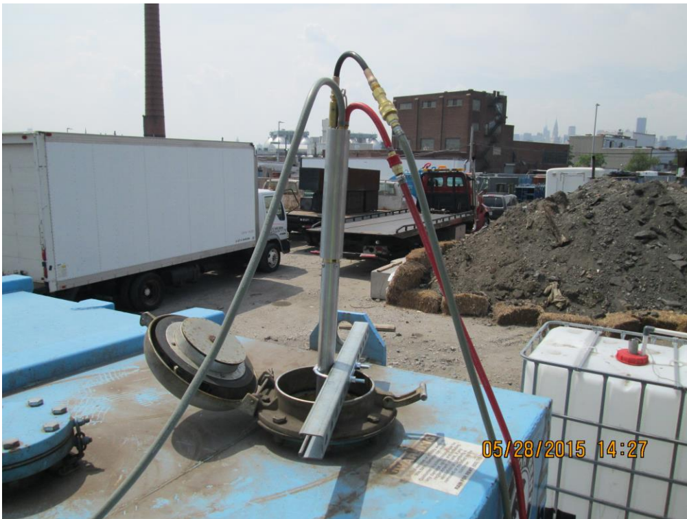
Skimmer pump installed and operational on frac tank
