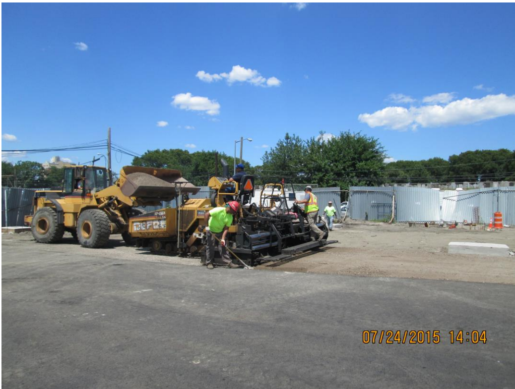
Install DGA base in final pavement section on RAD II
