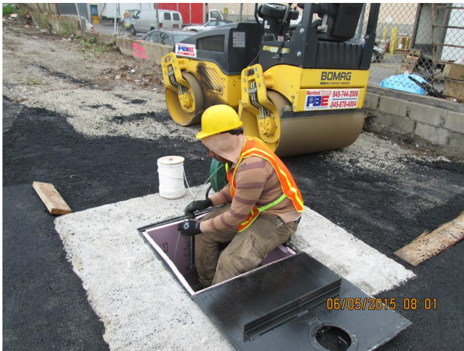
Electricians Pull Drag Lines for Process Piping Installation
