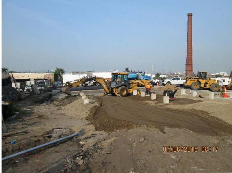
Fill under Equipment trailers
