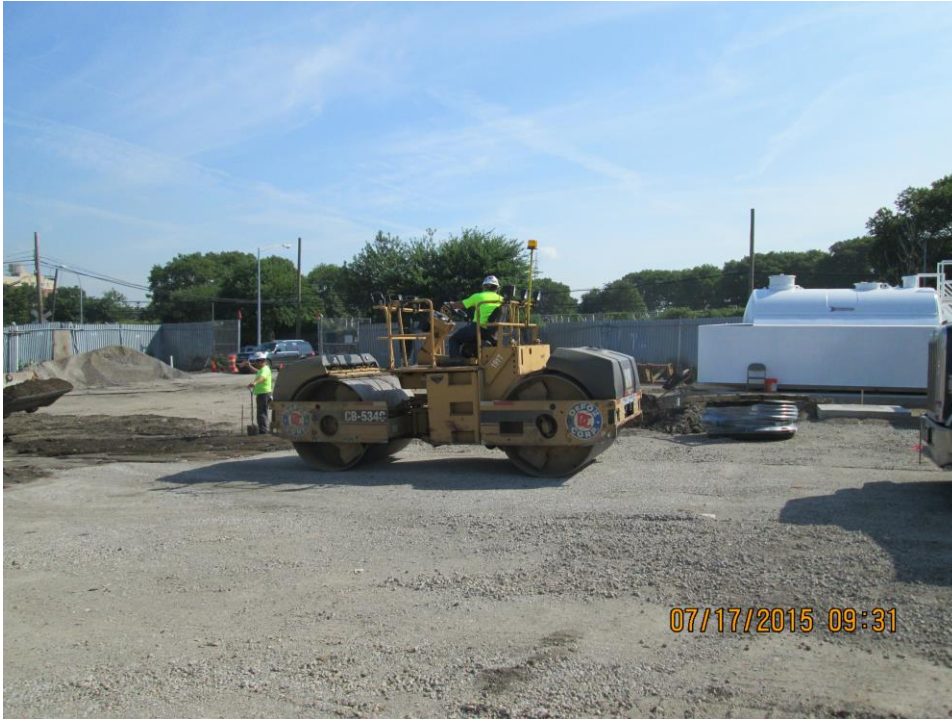
Compact DGA subbase between S-1 line and Equipment trailer
