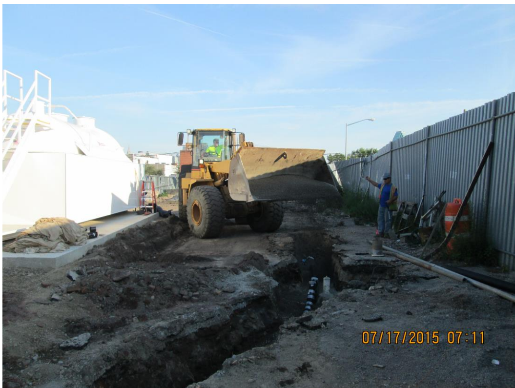
Backfill trench segments 48 and 50
