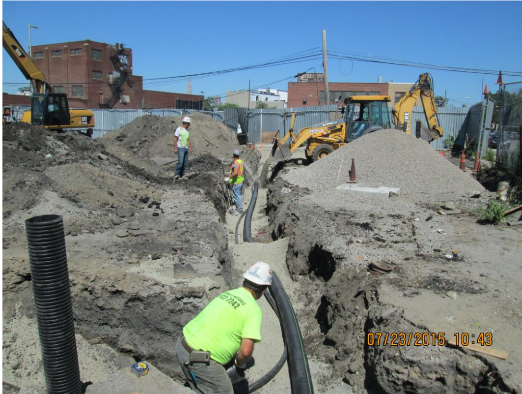
Trench segment 44 showing force main installation
