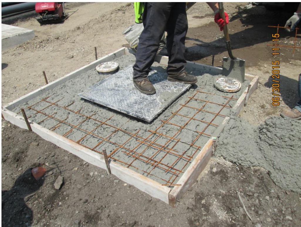
Pour Hose Vault Pad note two sumps on TF-7 and TF-6 lines
