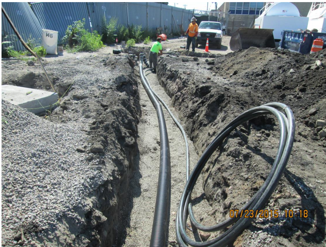
Trench segment 54 from S-3A to north crossing vault showing force main
