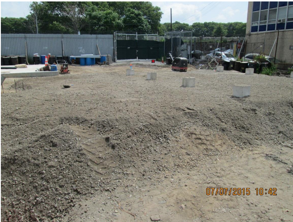
DGA subbase under equipment trailers
