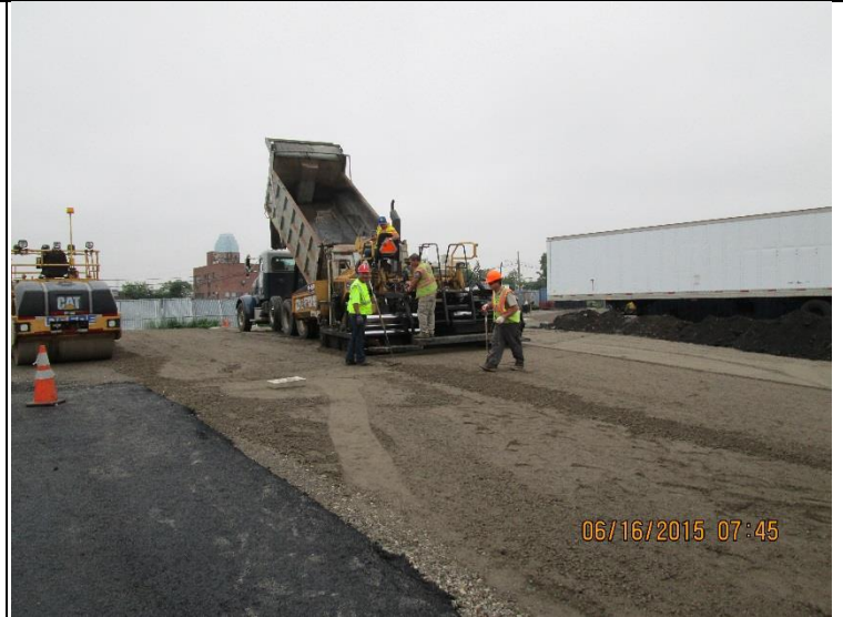
Install DGA between TF-2 line and TF-1 line on RAD II
