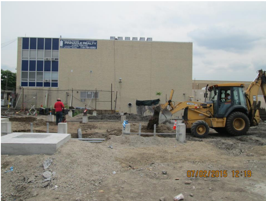
Using imported fill to bring grade at pier footing to elevation
