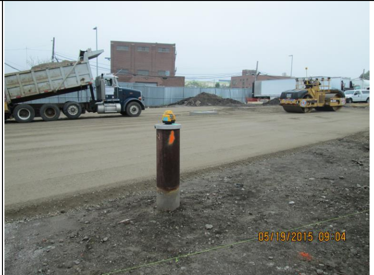
Place and Compact DGA RAD II Work Area I
