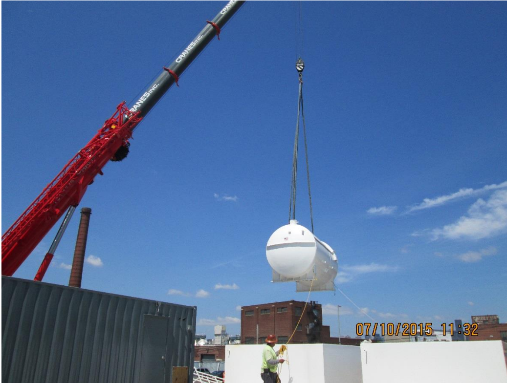
Rig LNAPLE tank into containment structure
