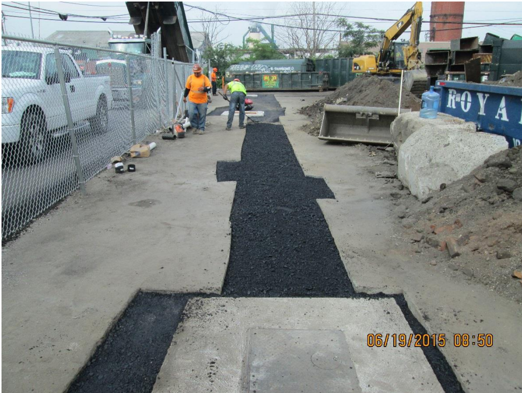
Binder on RAD I trench segments 25 and 26 between TF-6D and TF-6B
