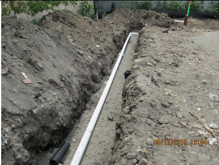
North-South Trench from TF-5A to TF-4A. SVE piping only
