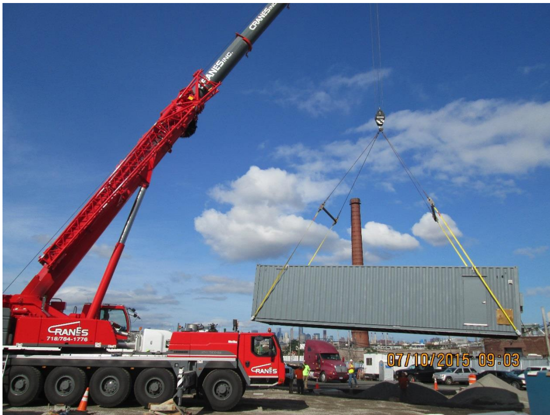
Rig equipment trailer onto pier footing base plates
