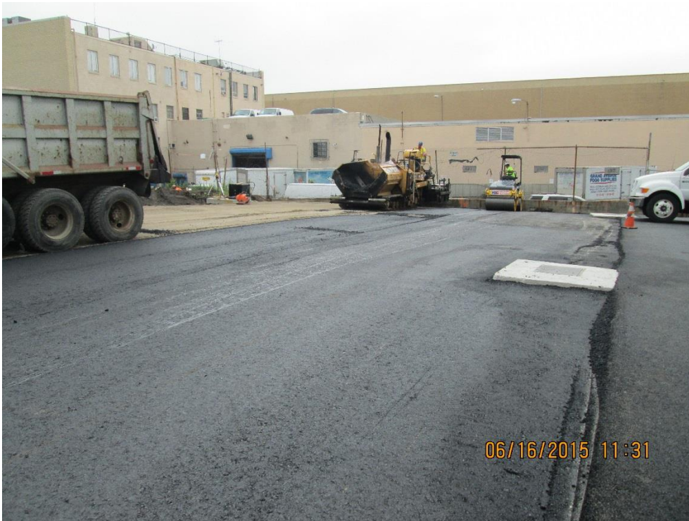
Install binder course between TF-2 line and TF-1 line on RAD II
