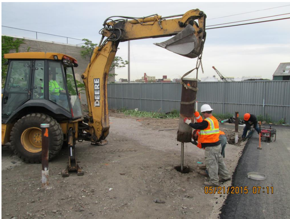
Remove VER-2 Protective Casing
