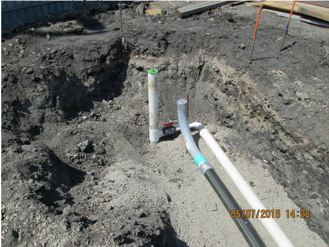
TF-4D Well Head Piping- End of line VER Low Point Well Head detail
