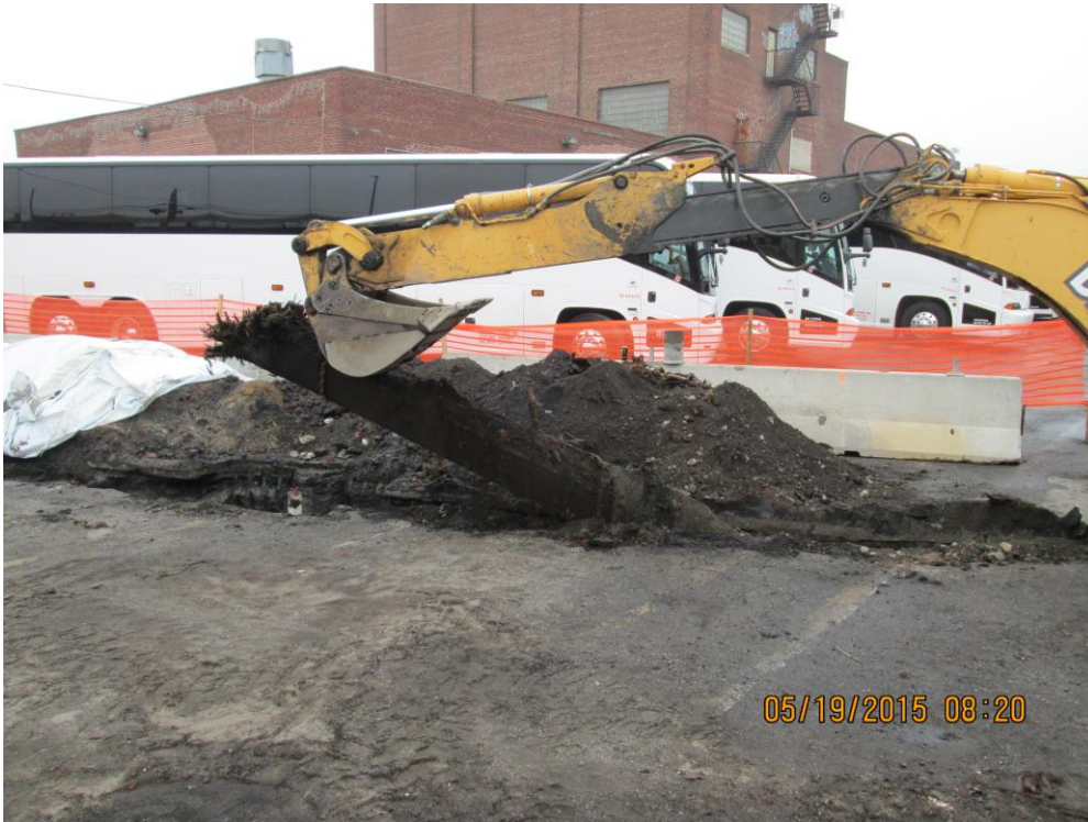
Remove Timber from TF-7 Trench
