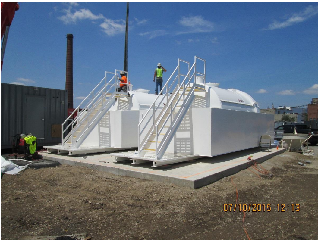
Final LNAPLE tank installation
