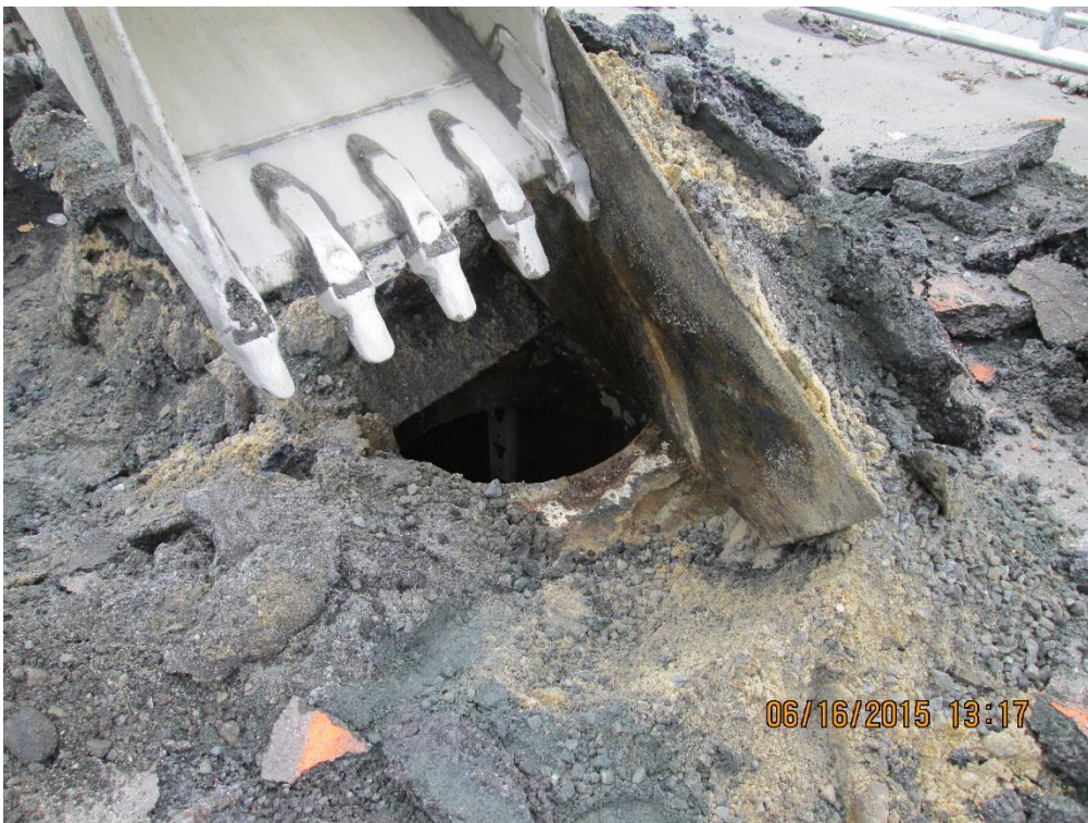
Uncover abandoned concrete vault on RAD I between TF-6C and TF-6D trench segment 26
