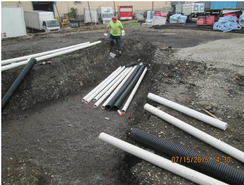
Trench segment 1 between Hose Vault and Equipment Trailer (TE-1)
