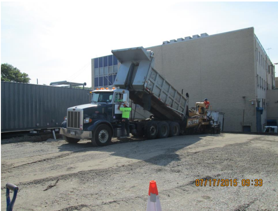
Place DGA subbase between S-1 line and Equipment trailer
