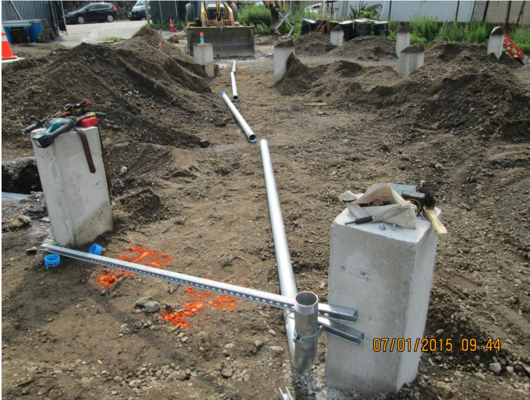
Install primary electrical conduit from switchgear to equipment trailer
