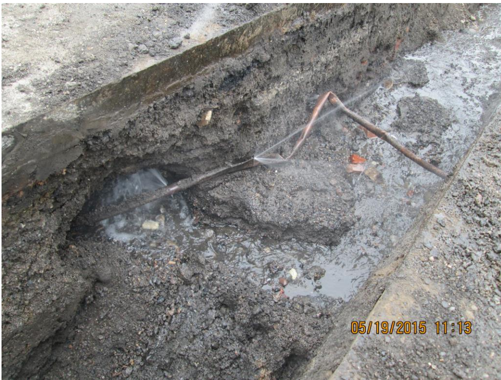
Broken Water Line TF-7 Trench
