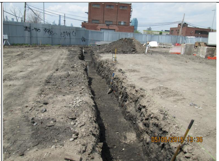
TF-4 trench showing compacted subgrade
