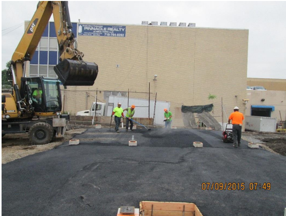
Top course of pavement under equipment trailers
