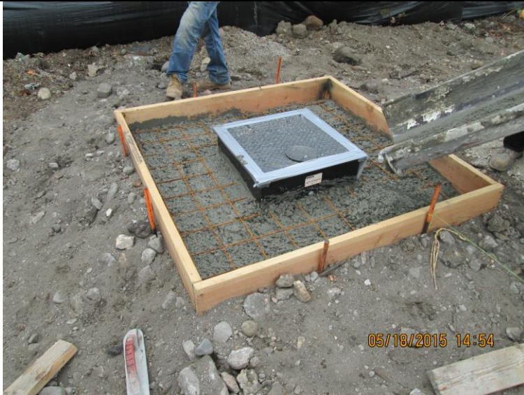
Concrete Pad for TF-5C Well Vault
