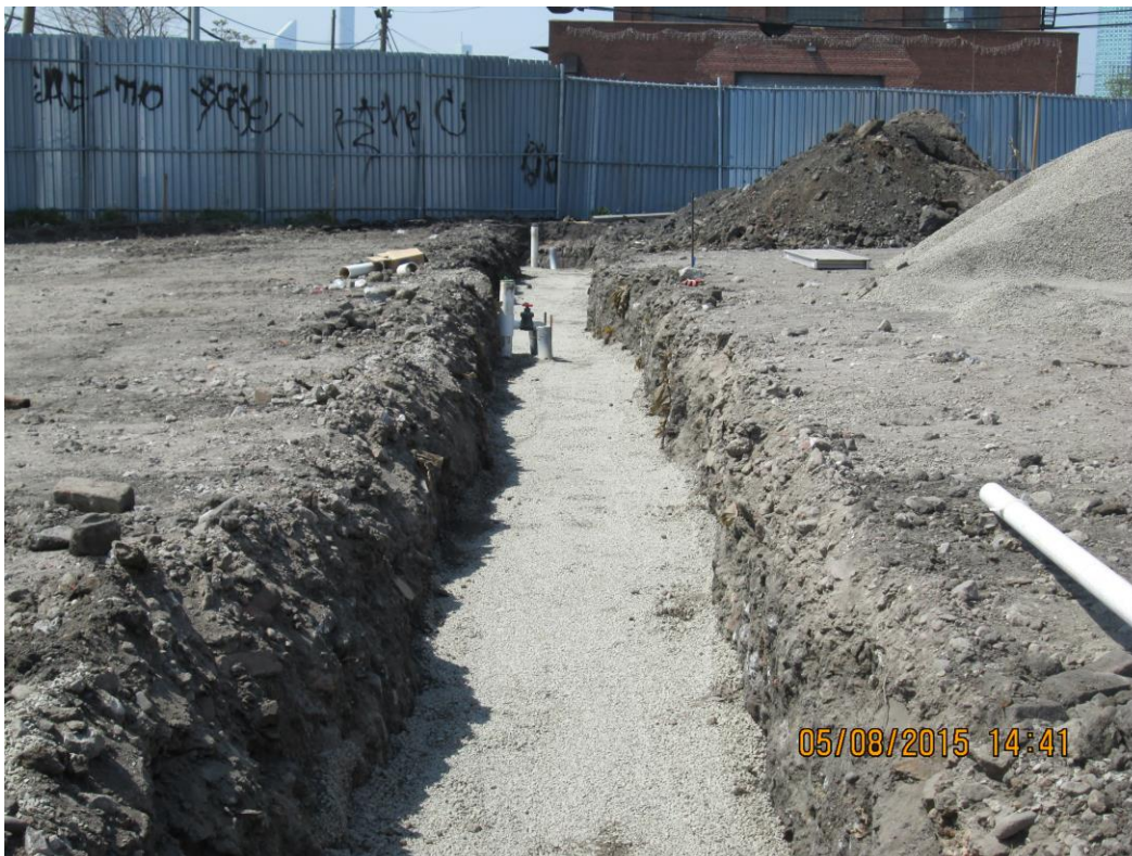
Second layer of bedding gravel over pipes in TF-4 trench
