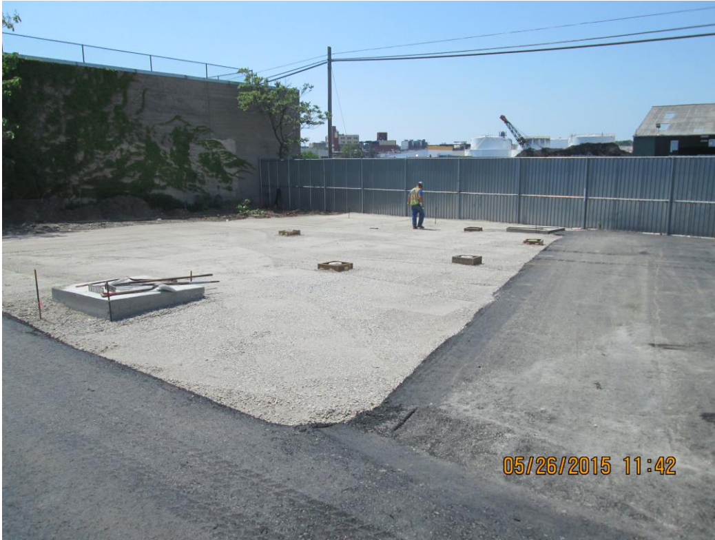
RAD II Work Area 1 Base course with monitoring wells framed for pour.
