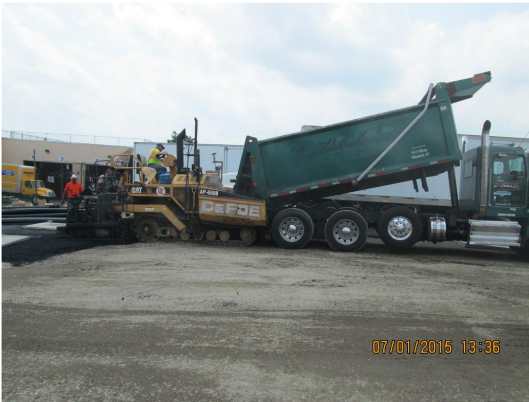
Base pavement between TF-1 line and S-1 line
