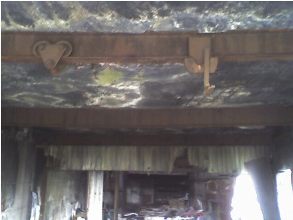
**Photo No. 24 – Damaged Roof Slab of One-Story Building**
