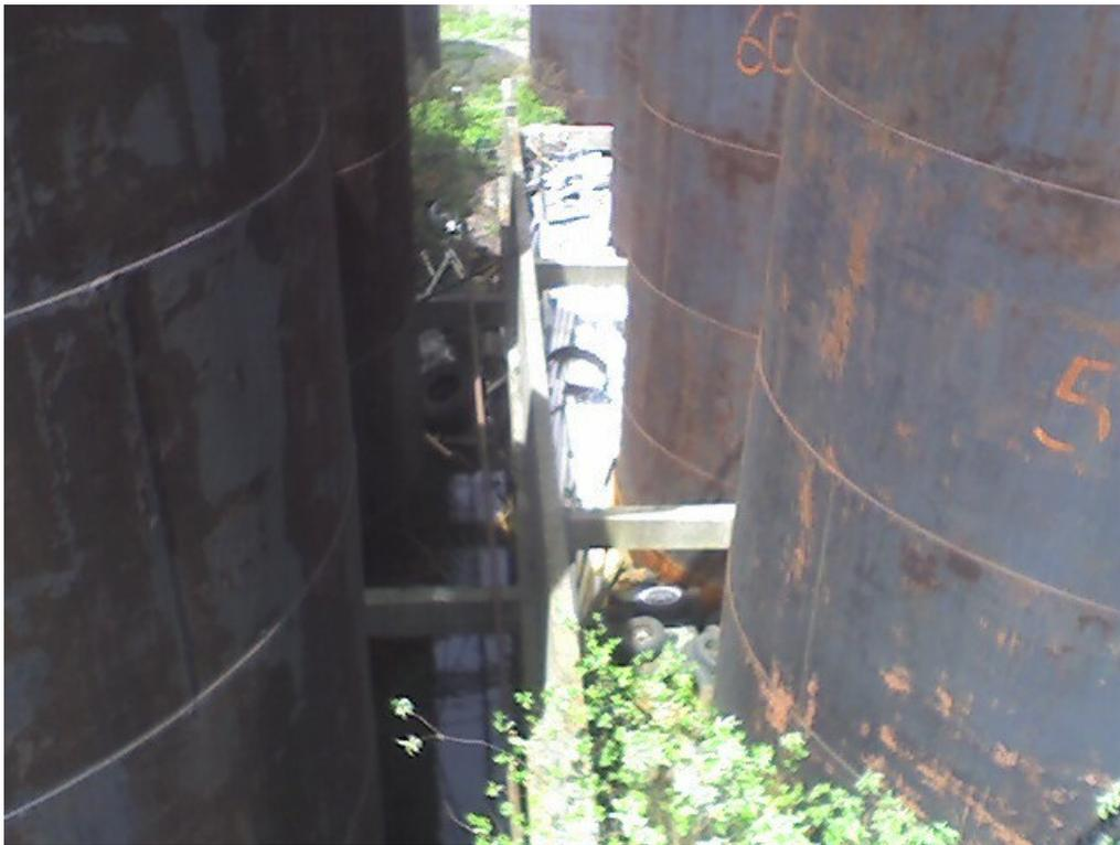
**Photo No. 14 – Oil Tank Containment Concrete Walls and Beams**
