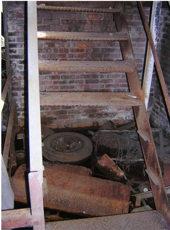
**Photo No. 21 – Damaged Interior Metal Stairs at 1<sup>st</sup> Floor
