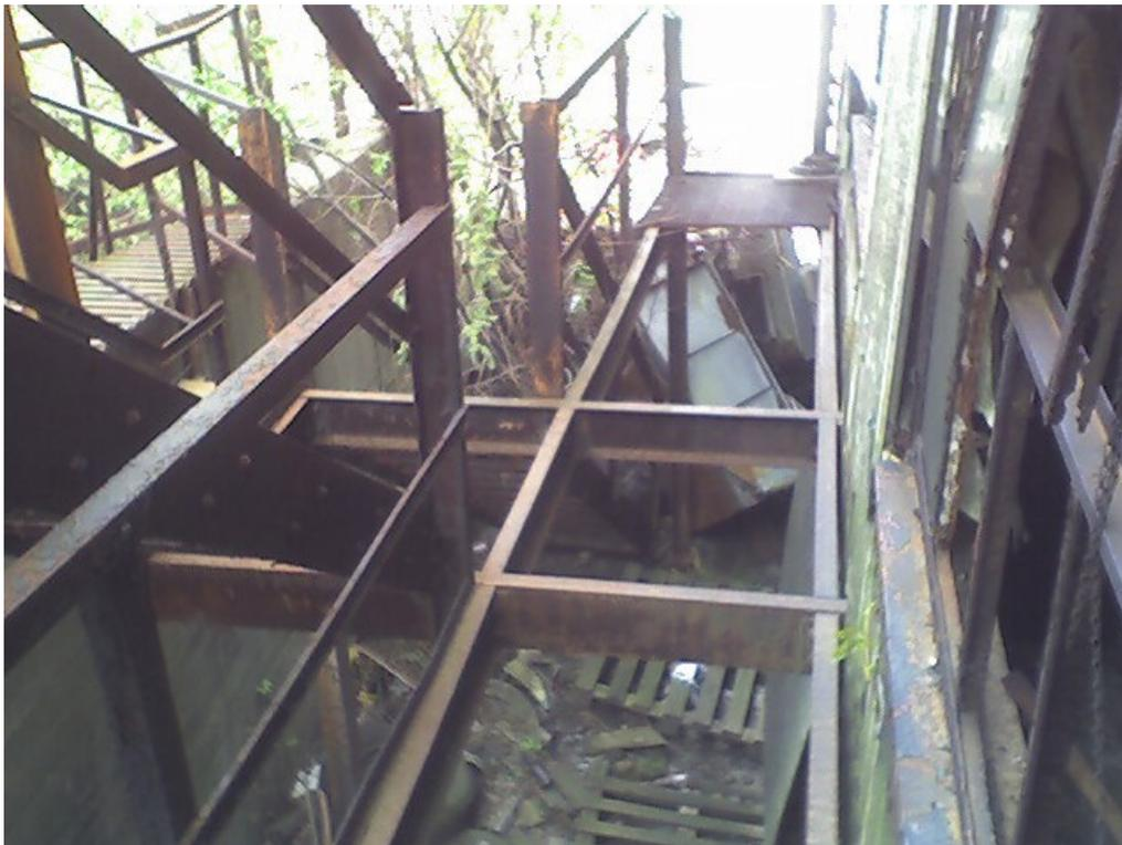
**Photo No. 18 – Missing Landing at Western Exterior Metal Stairway of Four-Story Building**
