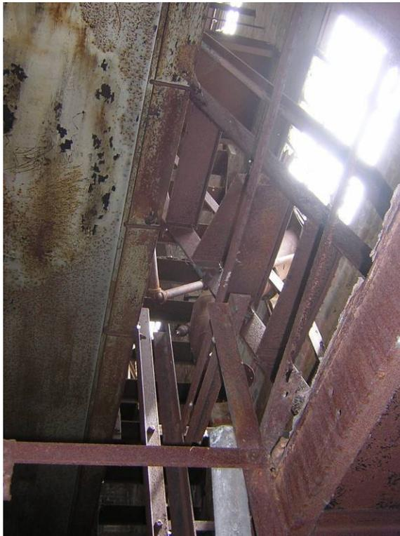
**Photo No. 22 – Damaged Interior Metal Stairs at 1<sup>st</sup> Floor
