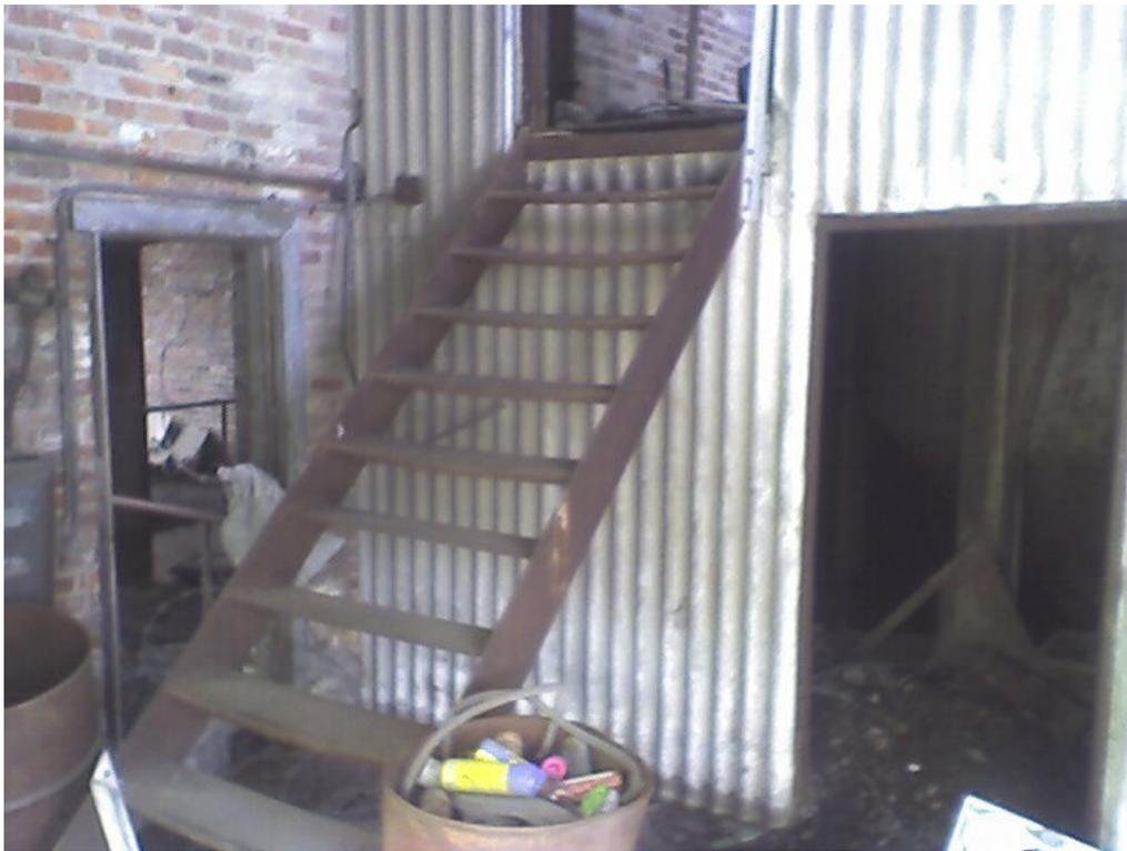
**Photo No. 17 – Missing Handrails at Eastern Exterior Metal Stairway of Four-Story Building**
