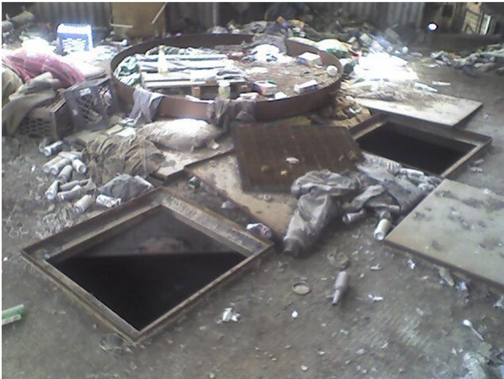
**Photo No. 16 – Two Unprotected Floor Openings at 2<sup>nd</sup> Floor of Four-Story Building**
