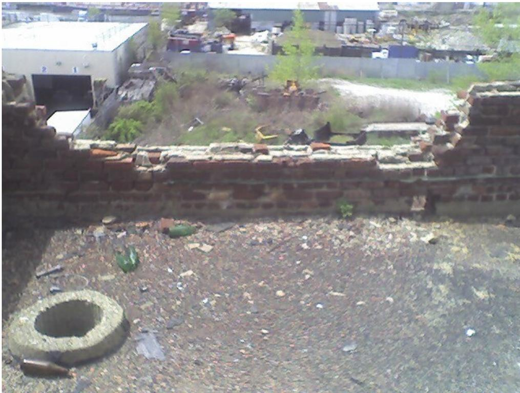
**Photo No. 19 – Loose Masonry & Mortar at Roof of Three-Story Building**
