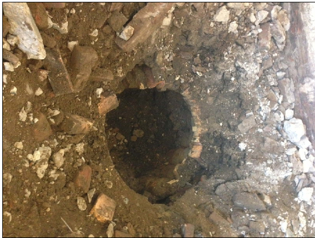
Photograph 2: Underground cooking pot structure made of brick.
