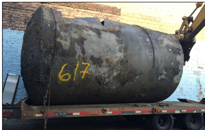
29. Photo taken on March 11, 2015. View of CT 6 loaded on trailer bed for disposal offsite.
