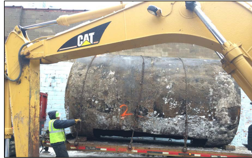
14. Photo taken on February 2, 2015. View of CT 2 prior to removal from site.
