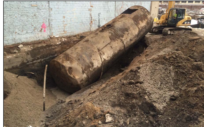
16. Photo taken on February 5, 2015. View of CT 9 being removed from the excavation.
