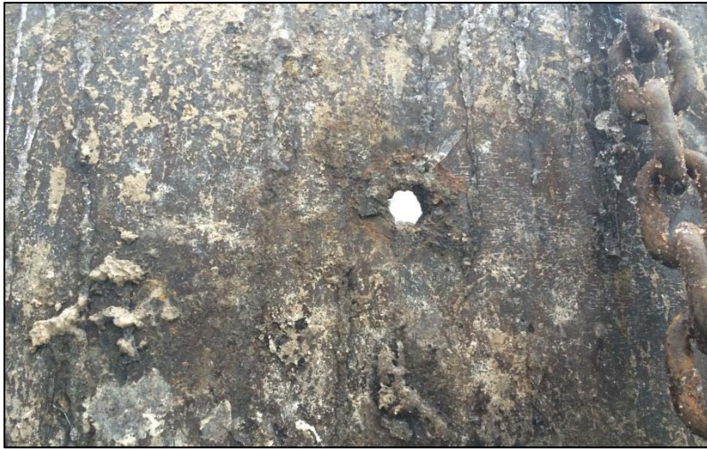
13. Photo taken on February 2, 2015. View of the hole in the side CT 5.
