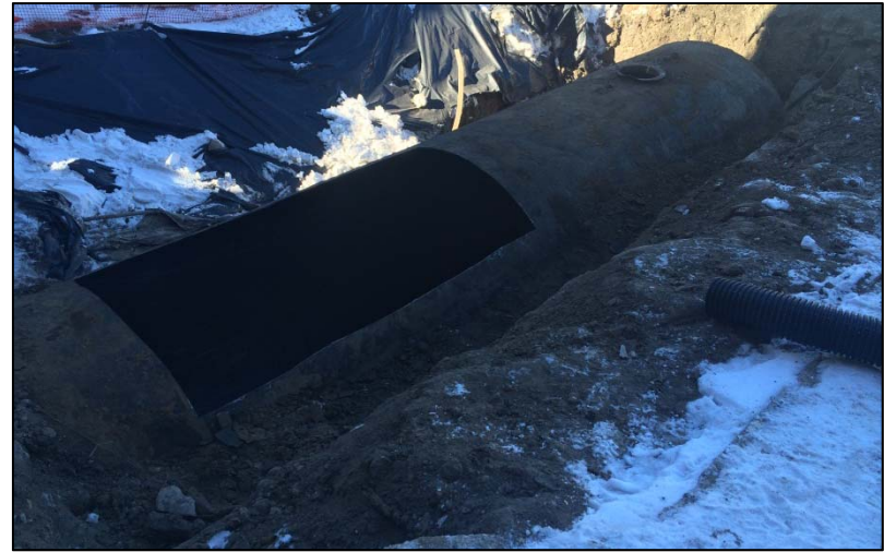
10. Photo taken on January 28, 2015. View of CT 2/5 ready to be pulled from excavation.
