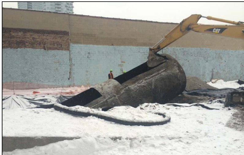
11. Photo taken on January 30, 2015. View of CT 2/5 being pulled from the excavation.
