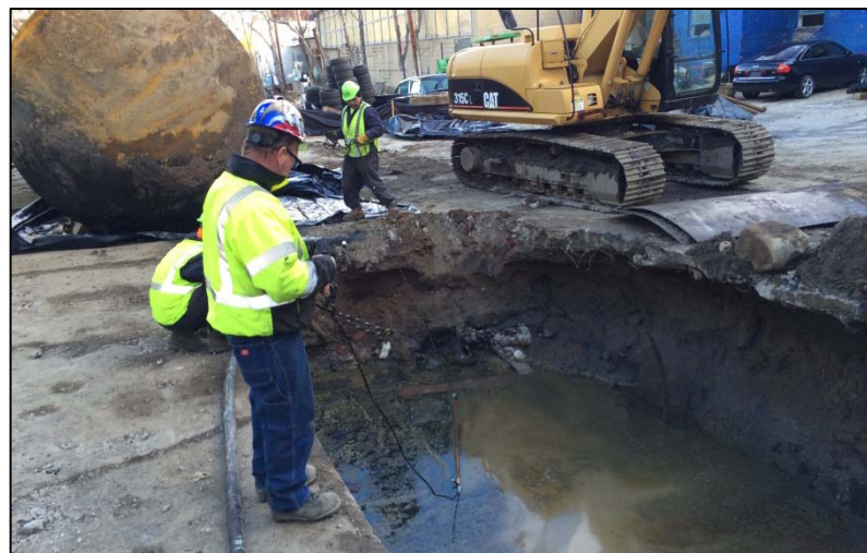
6. Photo taken on January 20, 2015. View of Metro laborer skimming product off of the top of the groundwater in the excavation of CT 3/4.
