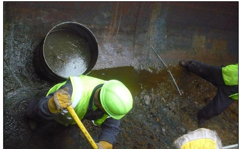
4. Photo taken on January 18, 2015. View of Metro laborers cleaning the tank bottoms from CT 3/4 and containing the tank bottoms in drums.
