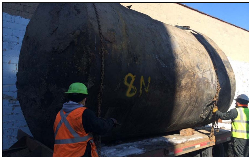
23. Photo taken on February 24, 2015. View of CT 8 (North) loaded on trailer bed for disposal offsite.
