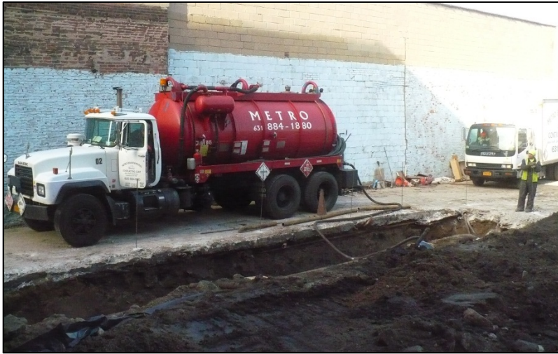
1. Photo taken on January 15, 2015. View of a vacuum truck pumping the contents of CT 3/4.
