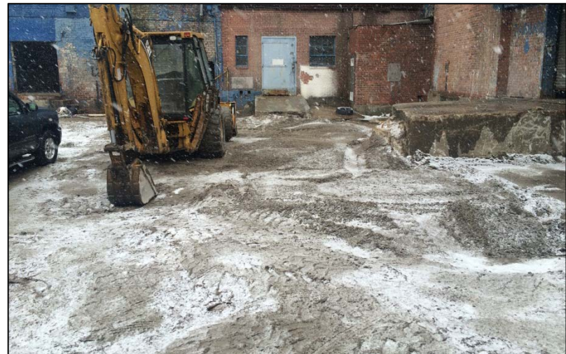
35. Photo taken on March 20, 2015. View of the courtyard following the removal of all known USTs.
