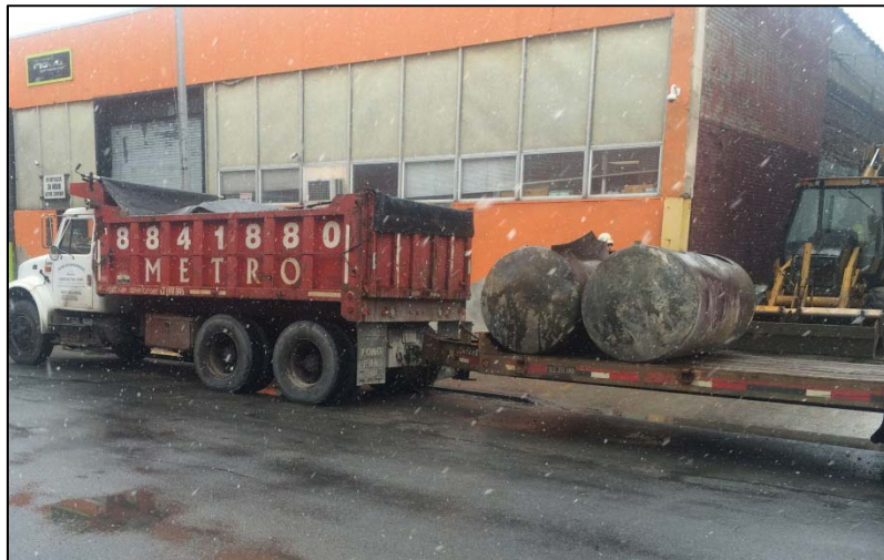
34. Photo taken on March 20, 2015. View of F1 and F2 loaded on trailer bed for disposal offsite.
