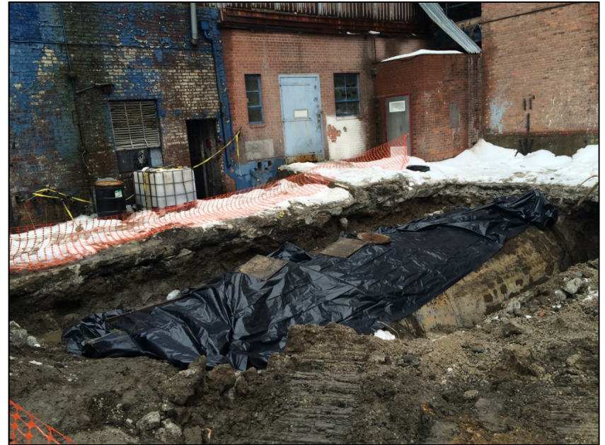
26. Photo taken on March 4, 2015. View of CT 6/7 in excavation.
