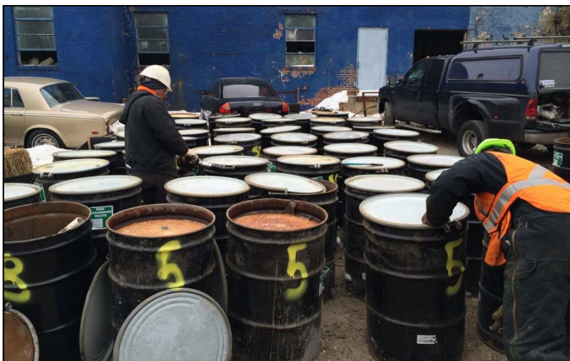
27. Photo taken on February 26, 2015. View of Metro laborers labeling drums containing tank bottoms.
