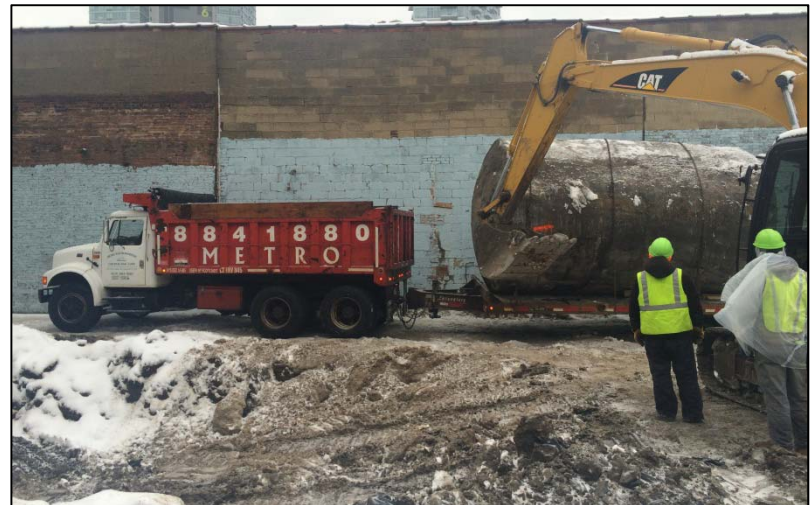
12. Photo taken on February 2, 2015. View of CT 5 prior to removal from site.
