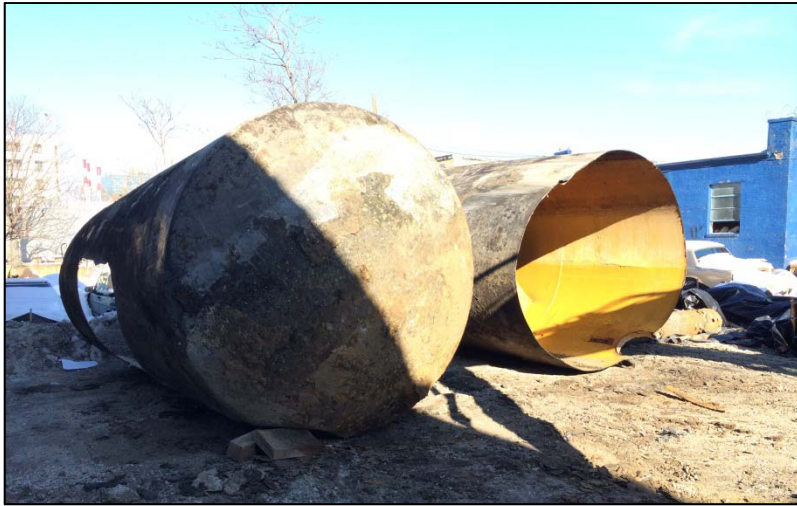
17. Photo taken on February 6, 2015. View of CT 9 split in half ready to be loaded on a truck for disposal offsite.
