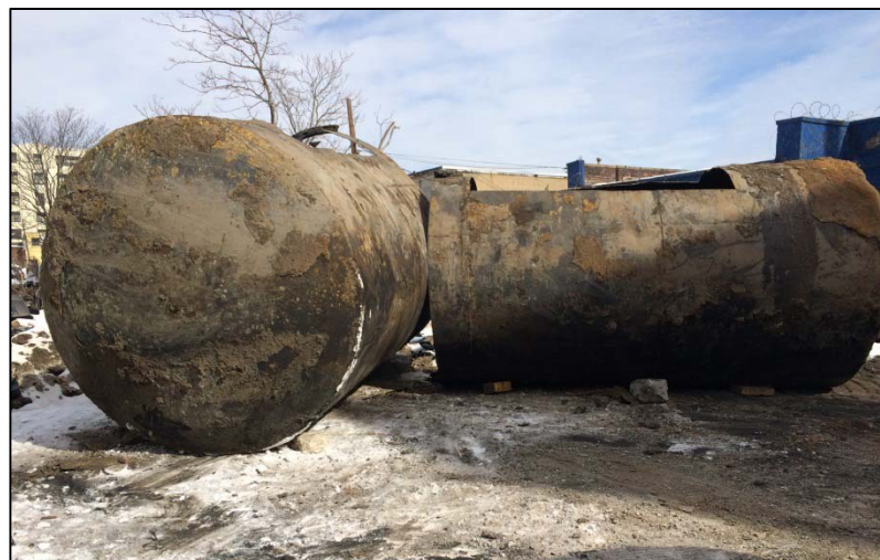
22. Photo taken on February 23, 2015. View of CT 8 cut in half following removal from excavation.
