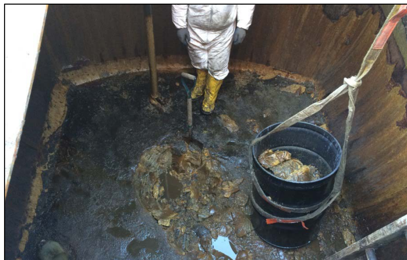
28. Photo taken on March 6, 2015. View of Metro laborer cleaning tank bottoms from CT 6/7.
