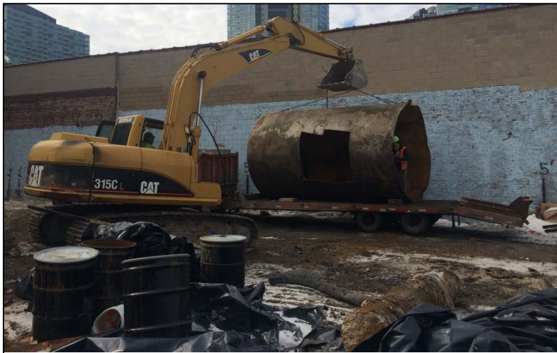
19. Photo taken on February 10, 2015. View of CT 9 (North) loaded on a trailer bed for disposal offsite.
