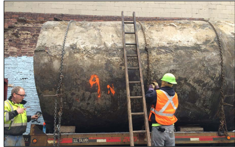
18. Photo taken on February 9, 2015. View of CT 9 (South) loaded on trailer bed for disposal offsite.
