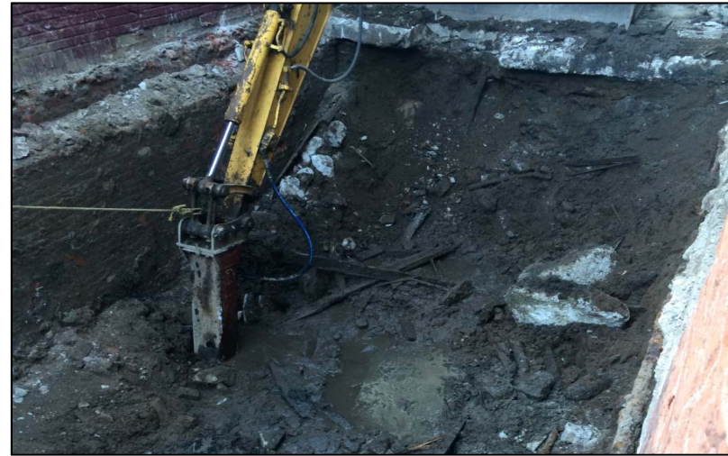
33. Photo taken on March 17, 2015. View F1 and F2 excavation following UST removal.
