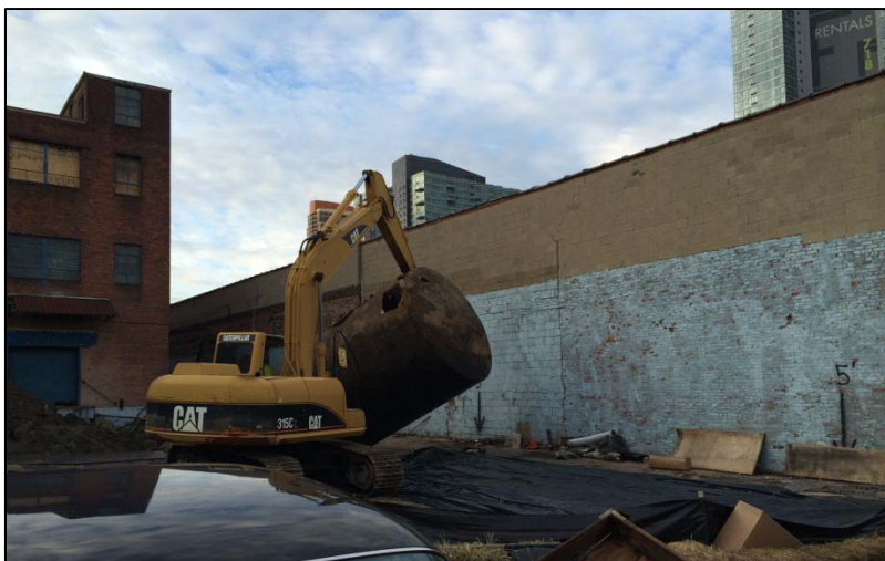
5. Photo taken on January 20, 2015. View of Metro operator using excavator to remove CT 3/4 from excavation.
