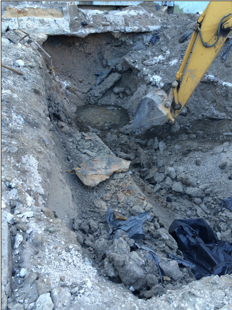
25. Photo taken on February 20, 2015. View of CT 1 tank excavation.
