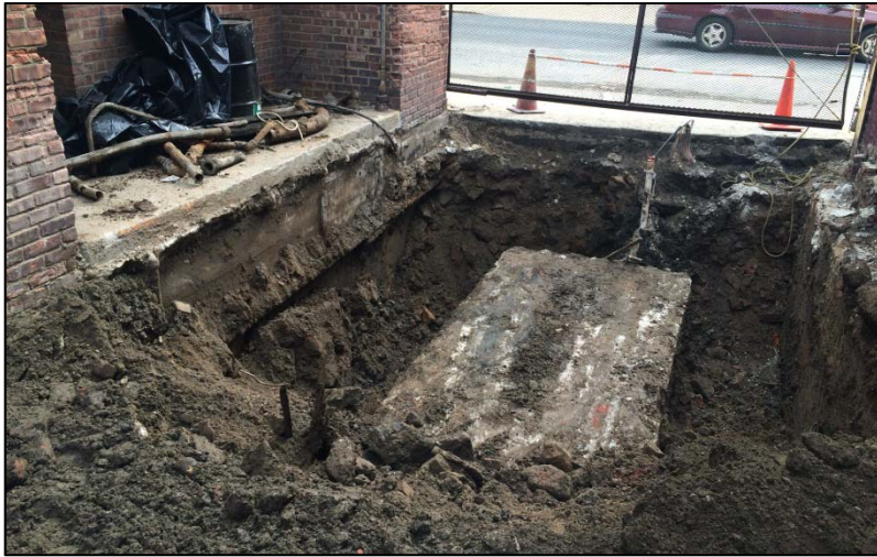
32. Photo taken on March 16, 2015. View of concrete vault containing F1 and F2.
