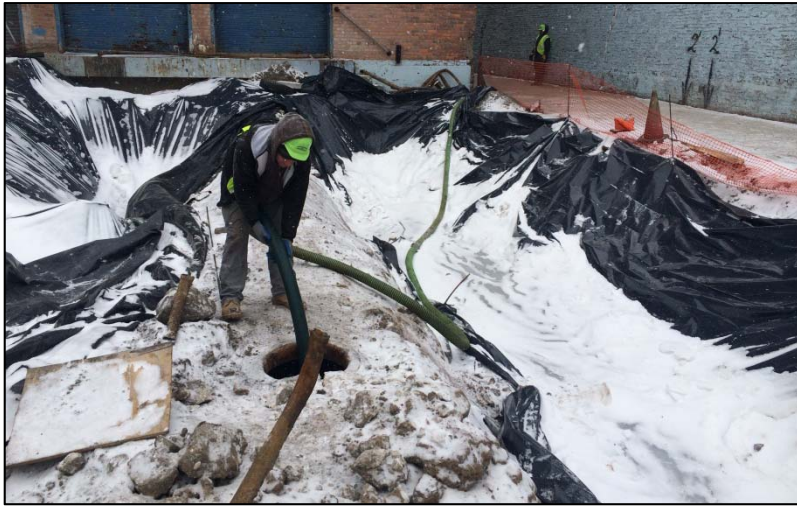
9. Photo taken on January 26, 2015. View of Metro laborer vacuuming contents of CT 5/6 in to a vacuum truck.
