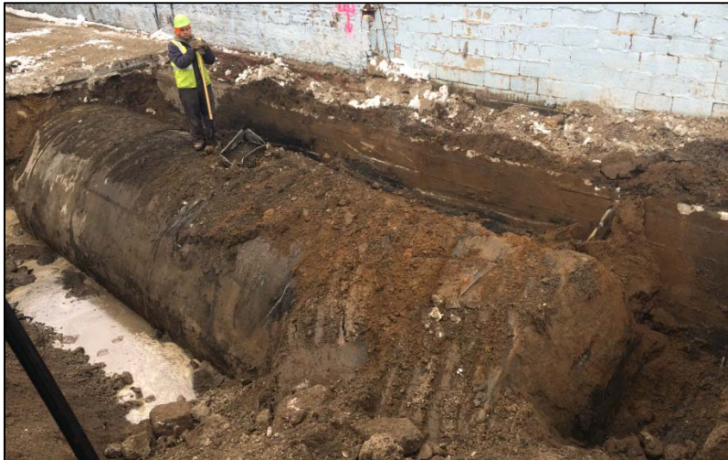
15. Photo taken on February 4, 2015. View of Urban laborer removing soil from the top of CT 9.
