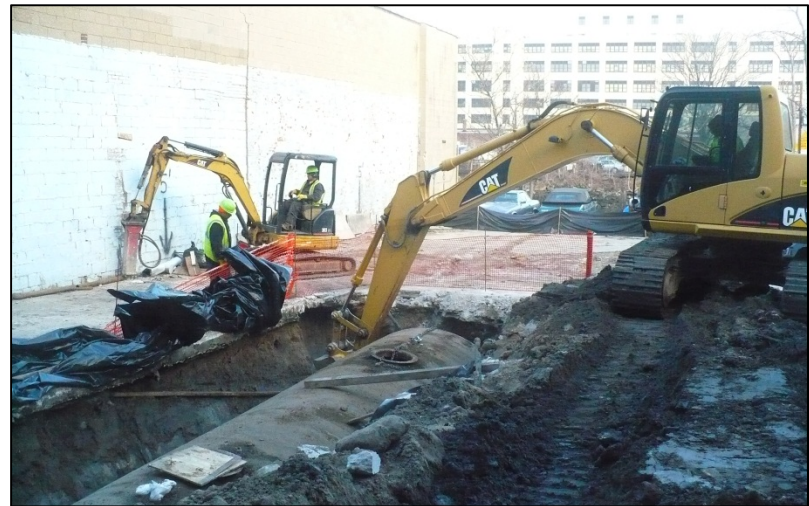
2. Photo taken on January 15, 2015. View of the excavator loosening CT 3/4 within the excavation and preparing it for removal.
