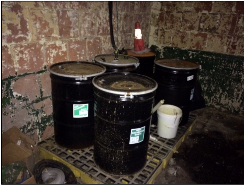
Photograph 11: Designated drum storage area with secondary containment pad
