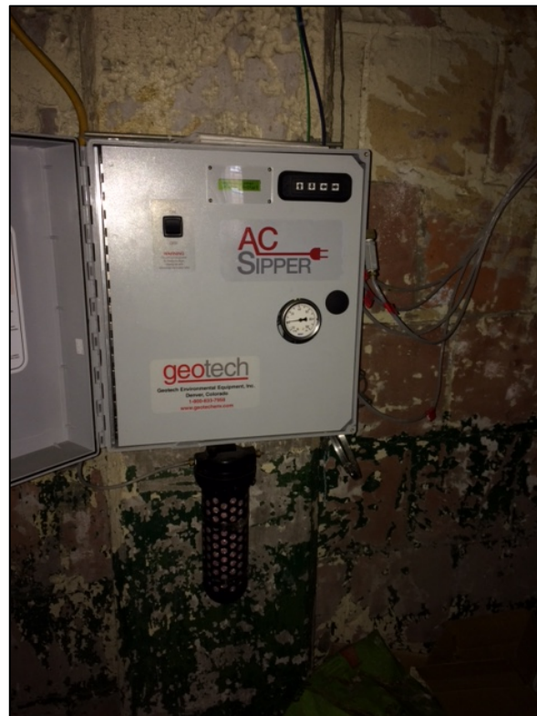
Photograph 12: Geotech AC Sipper control panel
