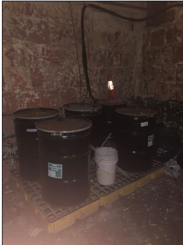
Photograph 11: Designated drum storage area with secondary containment pad
