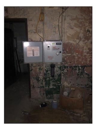
Photograph 10: Geotech AC Sipper control panel
