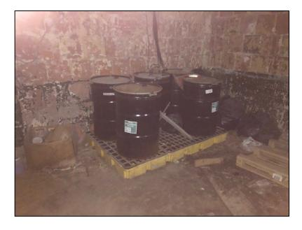
Photograph 9: Designated drum storage area with secondary containment pad
