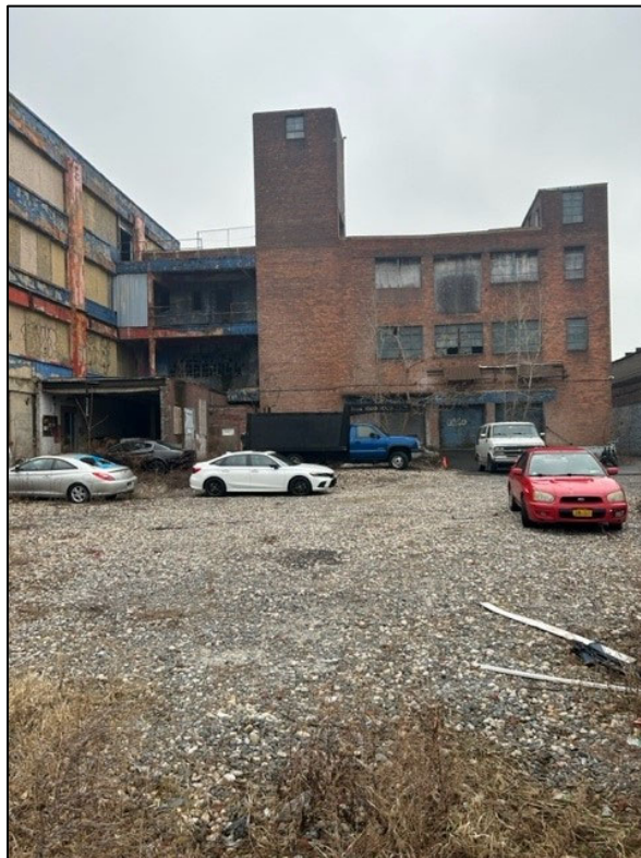
Photograph 4: Condition of warehouse and garage looking south
