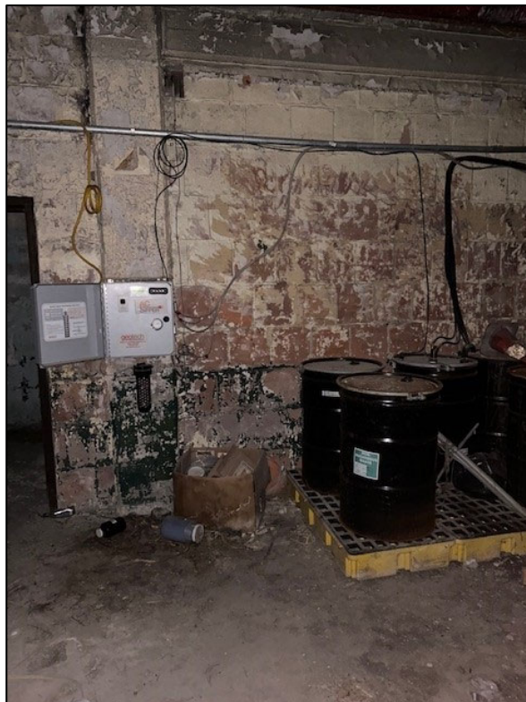
Photograph 10: Geotech AC Sipper control panel
