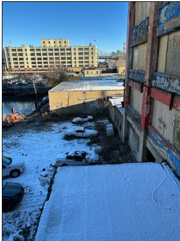
Photograph 6: Condition of courtyard looking north
