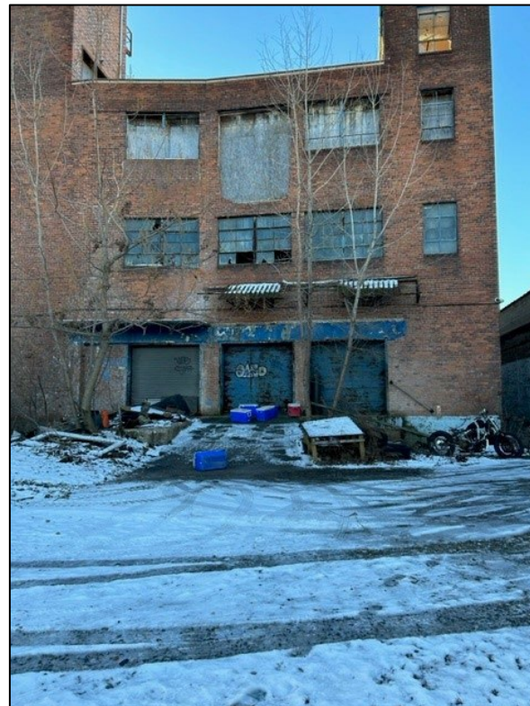
Photograph 2: Conditions of warehouse looking south
