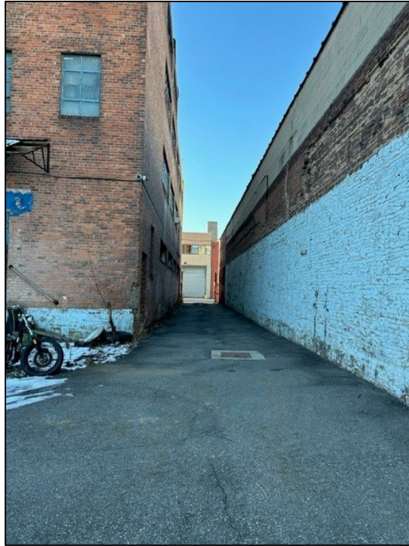
Photograph 1: Condition of driveway looking north
