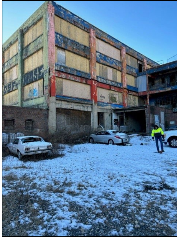
Photograph 3: Condition of paint factory and garage looking east
