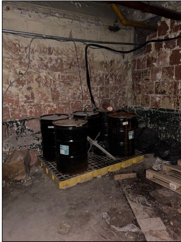
Photograph 9: Designated drum storage area with secondary containment pad
