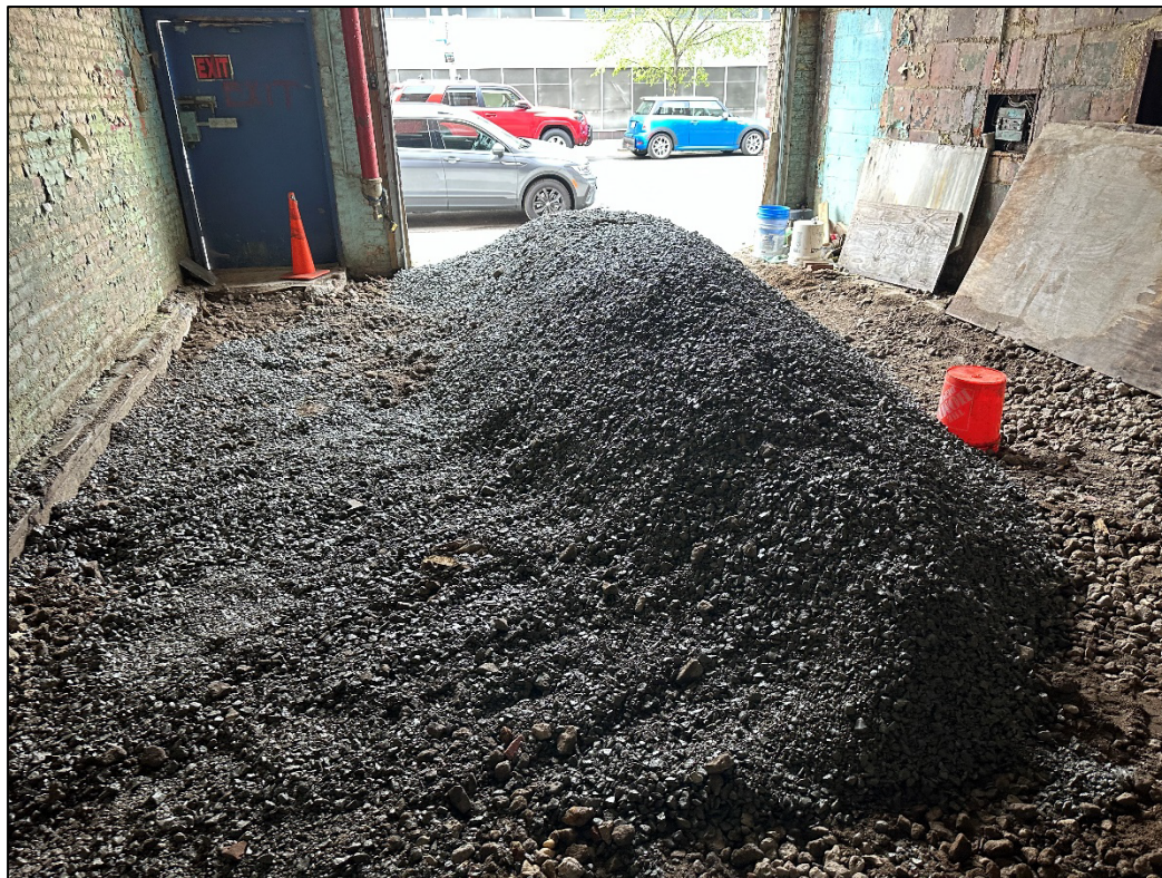
Photograph 14: RCA cap disturbance in garage covered with 2' of clean stone on April 18, 2024.
