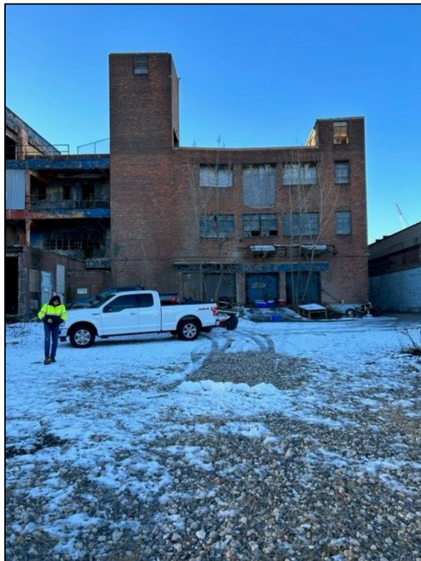
Photograph 4: Condition of warehouse and garage looking south
