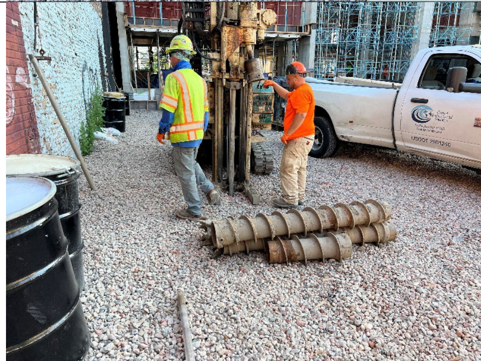
Photo 2: Facing northeast, view of Coastal drilling cores for RMW-7.
