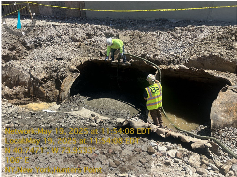
Photo 2: Facing east, Brookfield crew vacuuming out fluids from UST GT-4.
