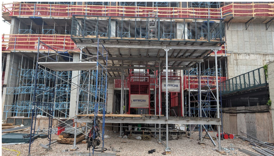
Photo 4: Facing north, truck platform and hoist support area being constructed.
