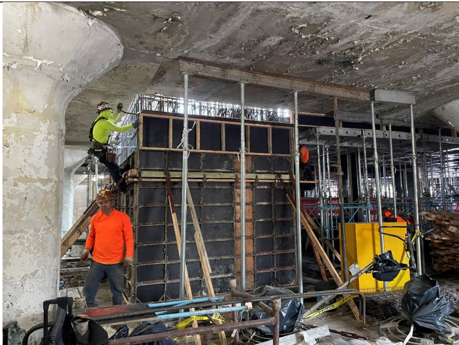
Photo 2: Facing southwest, NY Axon continues with form work around the building.
