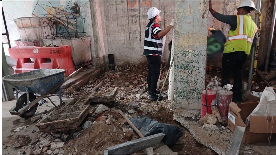
Photo 1: Facing south, view of Li Xiang Plumbing in trench work area.
