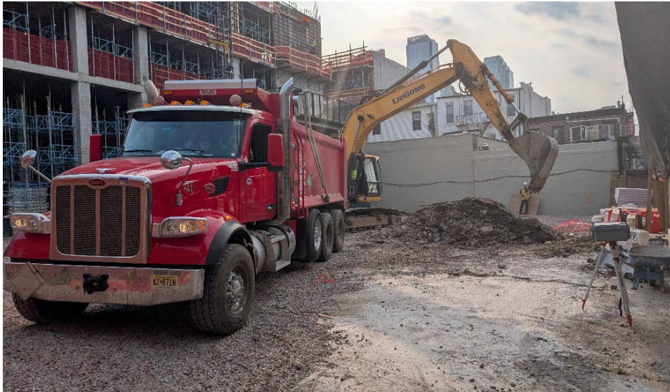
Photo 1: View facing east, the stockpile of GT-4 being loaded for transport.
