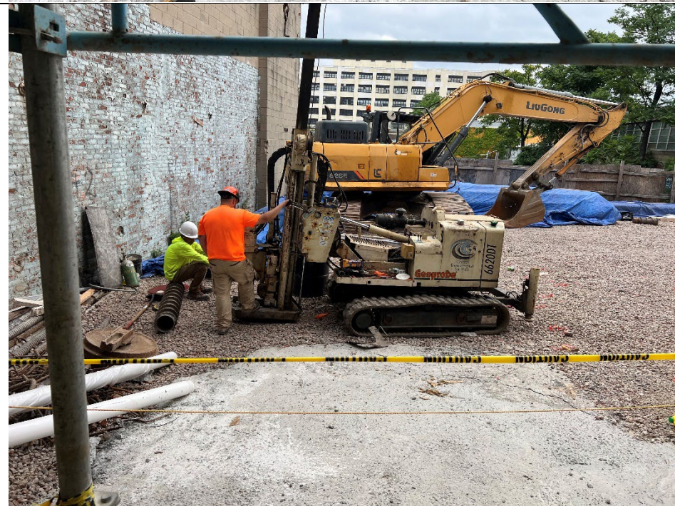
Photo 2: Facing north, view of Coastal drilling RMW-1.
