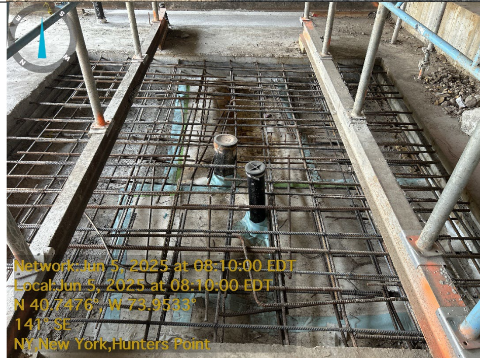
Photo 2: Facing southeast, view of un-poured pit with soil vapor barrier sealed.
