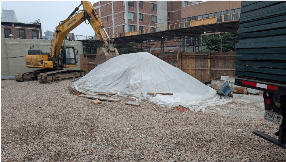
Photo 1: View facing southeast, stockpile of GT-4 material covered with poly.
