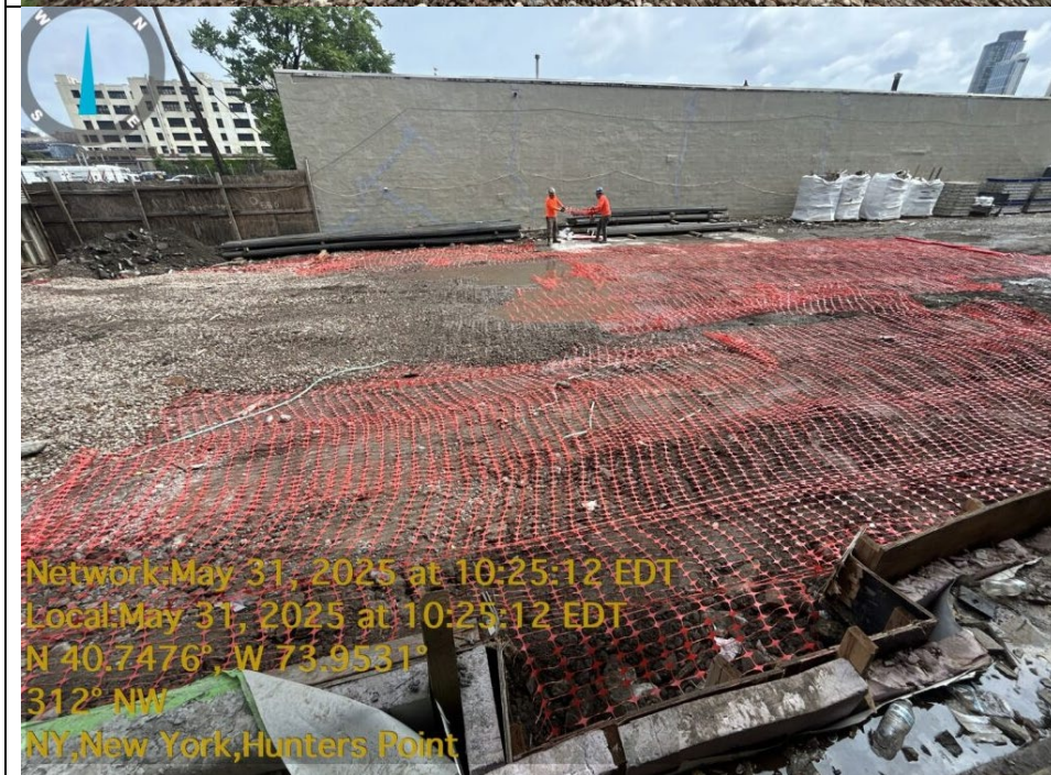
Photo 2: Facing north, view of demarcation layer placed in the northern portion of the Site.
