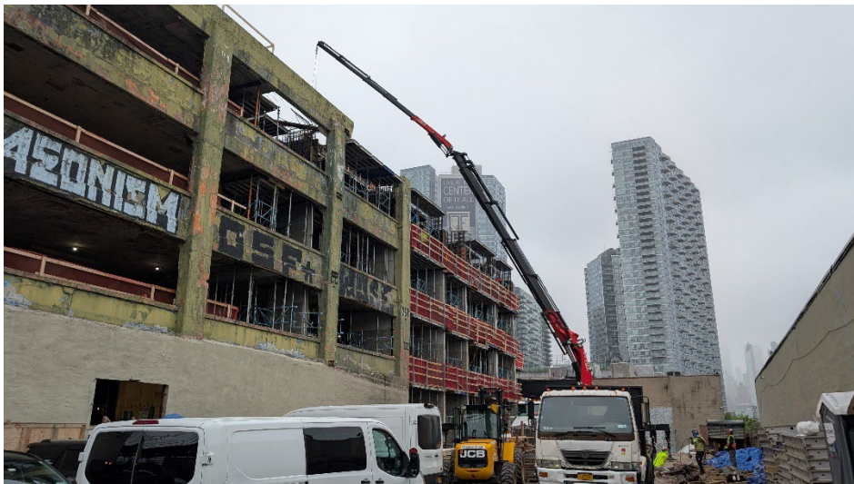
Photo 2: Facing west, Axon offloading rebar and materials.
