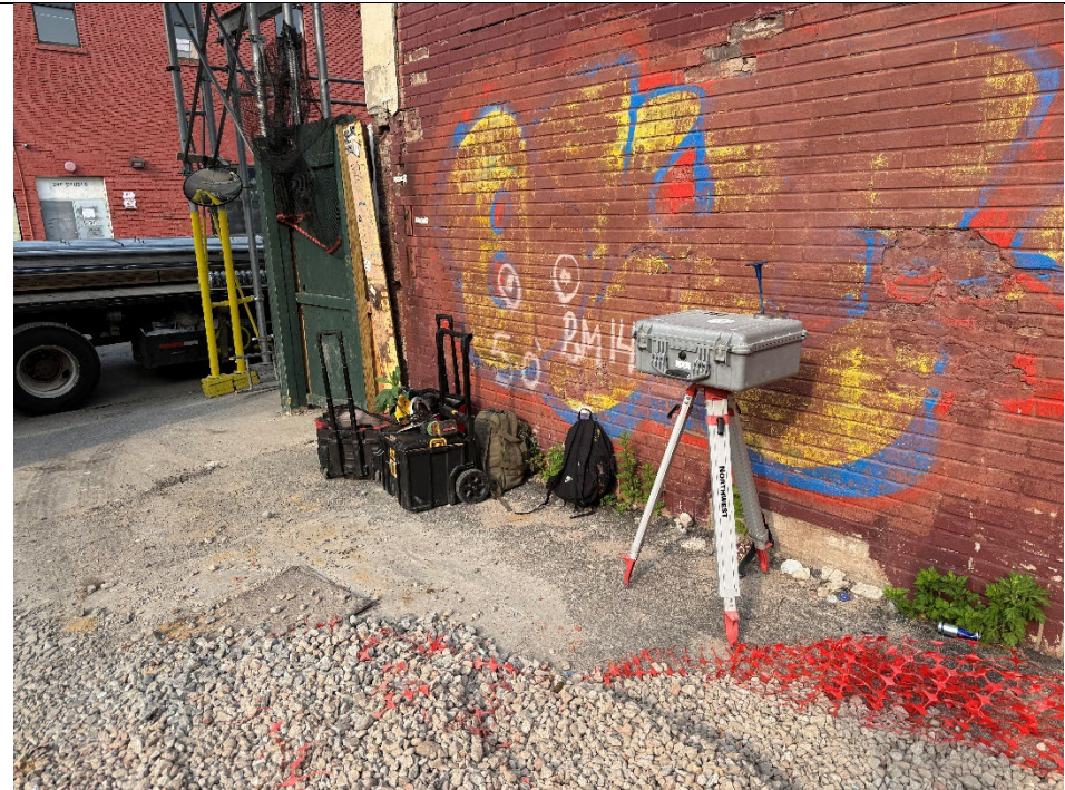
Photo 2: Facing south, view of downwind CAMP station location
