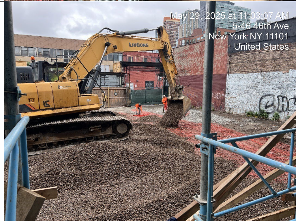
Photo 2: Facing southwest, view of NYC Axon spreading RCA stone on snow fence demarcation in southern portion of the Site.
