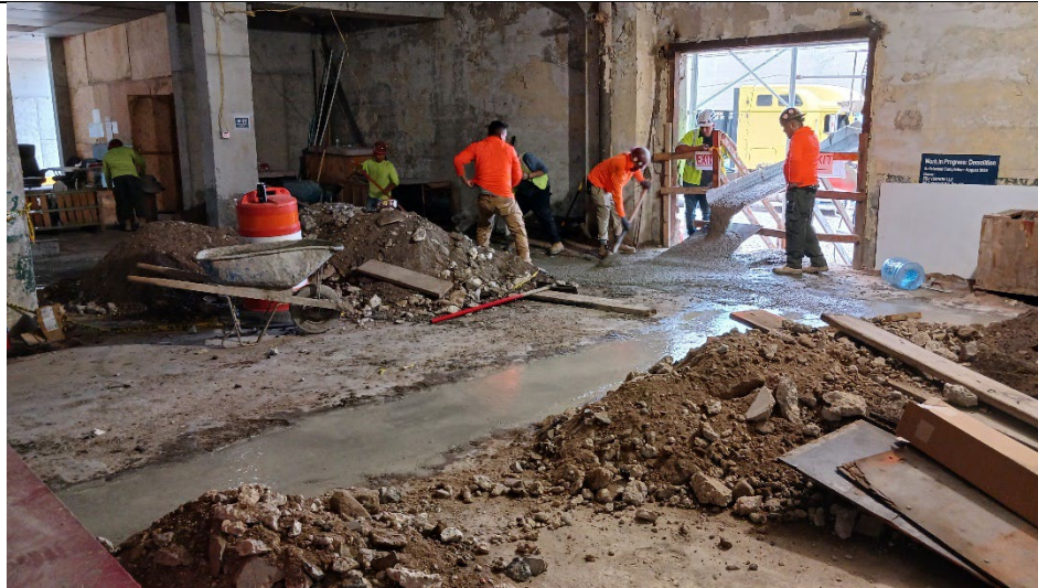
Photo 4: Facing north, view of pouring concrete to trench.
