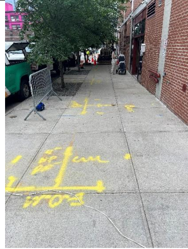
Proposed location for OS-MW-6 (down sidewalk by rig), unable to drill due to multiple utilities both marked and unmarked. Drillers hand cleared 2 holes and found utilities in both running in parallel with the HPG main and electrical. OS-MW-6 used as name for next well in series.
