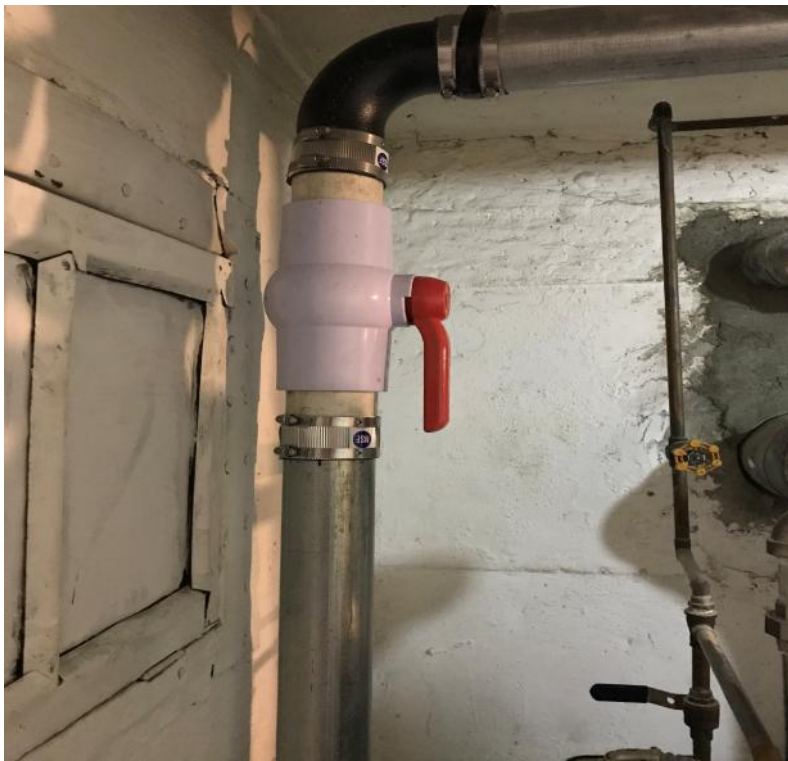
Photograph #5 – Suction point S5 PVC ball valve
