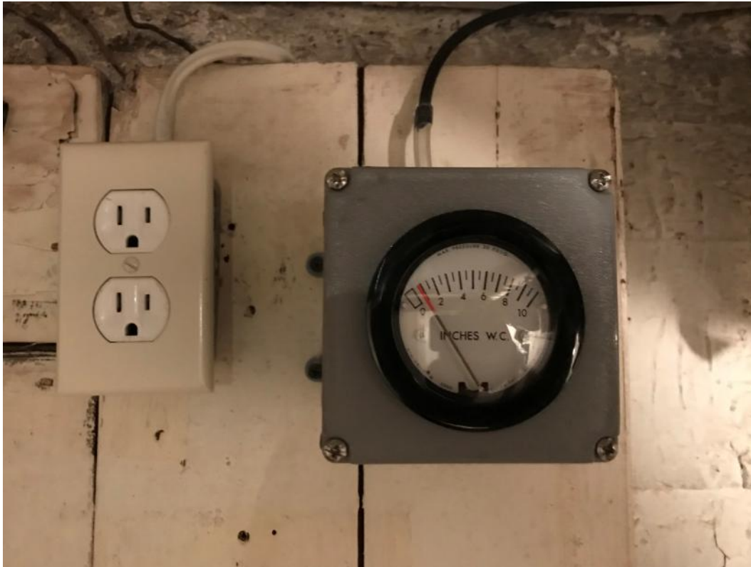
Figure 3. Properly functioning vacuum meter
