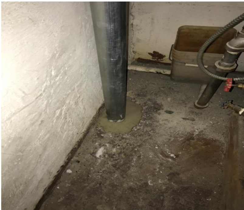
Photograph #6 – Suction point S5 floor seal
