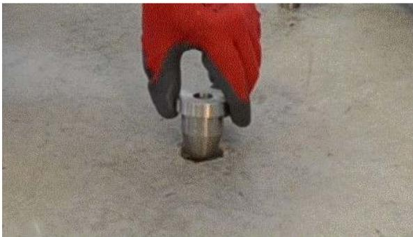
**Figure 3.** Installing the Drilling Guide.
